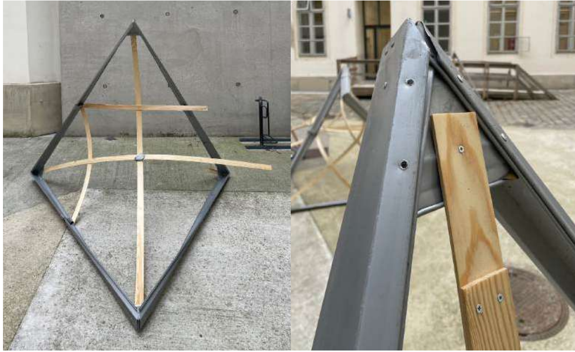
Fig.127 The detached connection stripes, one disassembled module, unriveting at one angle' side
