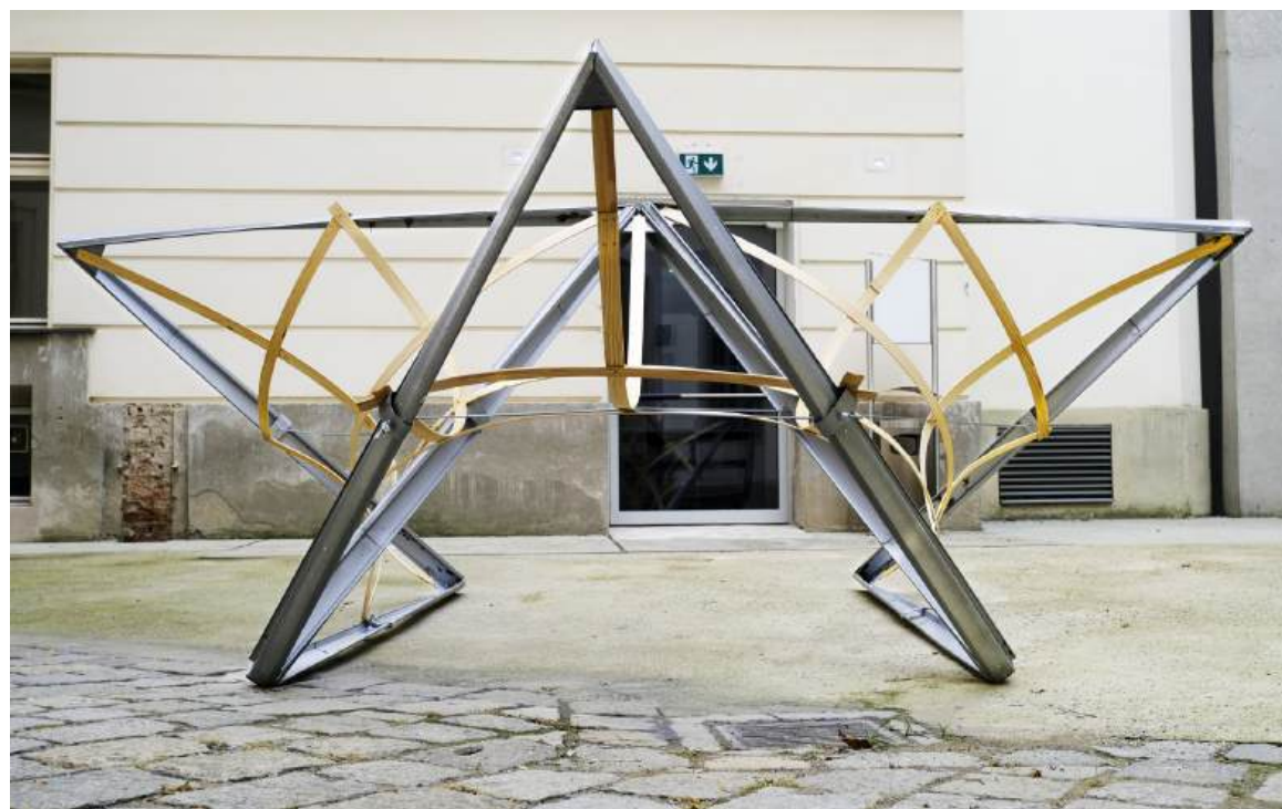
Fig.122 Three modules tied up together via steel and wood
