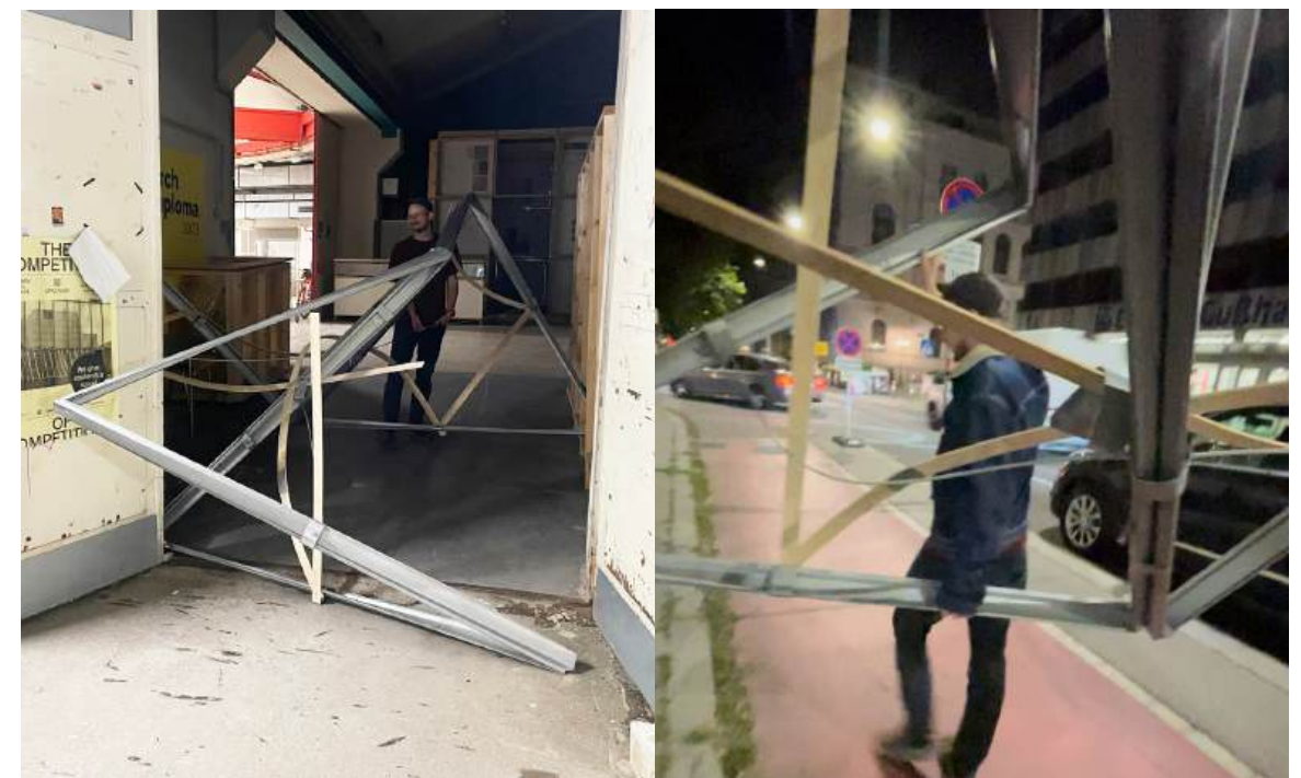
Fig.121 Left: transportation of the three partially connected bottom modules (variation 'bird'); right: transportation of the three upper modules
