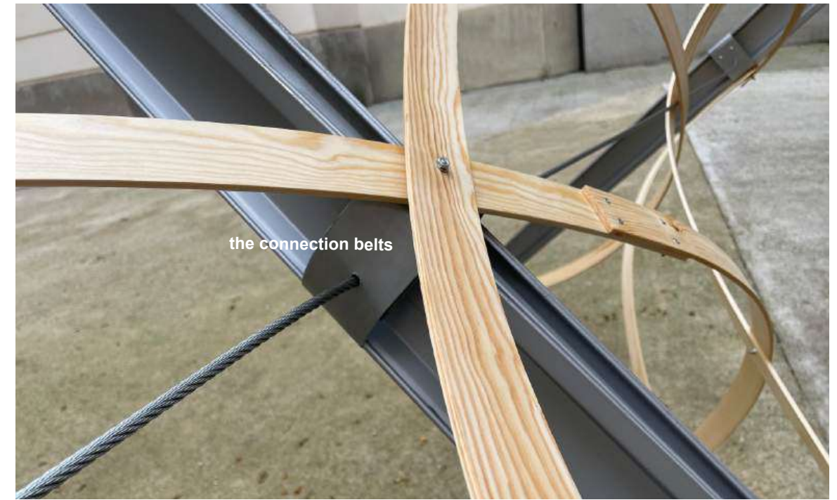
Fig.126 Connection between two modules
