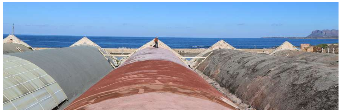
Fig. 19: The fifth bay after the collapse of the wooden roof in the 2006 earthquake.
