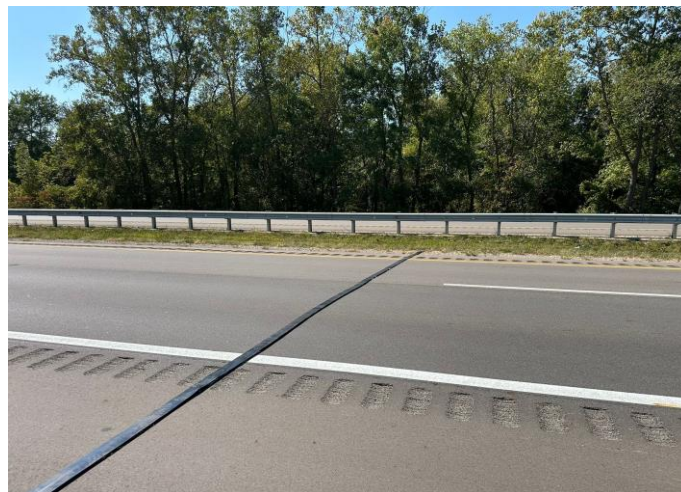
Figure 2. Strip laid across the road width at US 127, Mason, adjacent to a WIM system.
