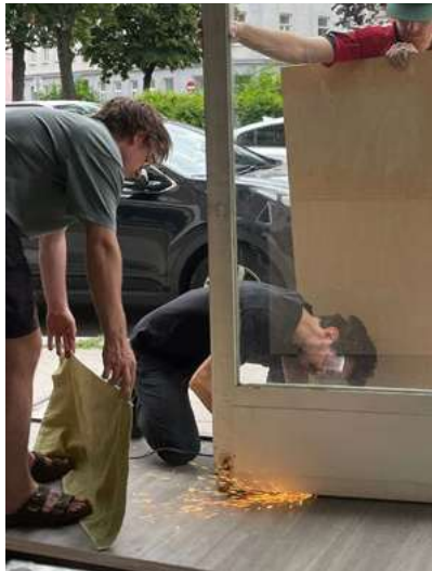
intervention on the stuck door: 07/2024 cutting the stuck bolt open
