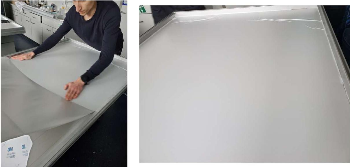
Figure 4.17: Application of the 3M PVC foil
