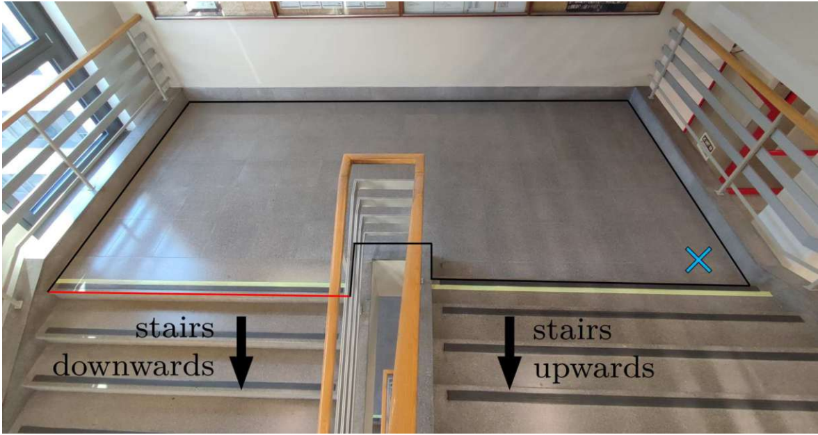
(a) View on the scene from the staircase with the ground truth plane marked in black and red
