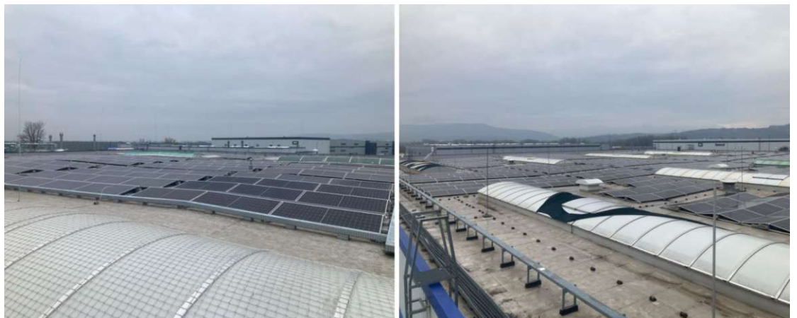
Picture 30 Installation of 2 MWp solar cells at HSK finished by Dec/24
