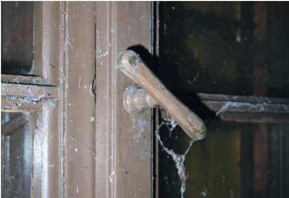
Abb. 272 Olive, Fenster, EG_02_F_01
