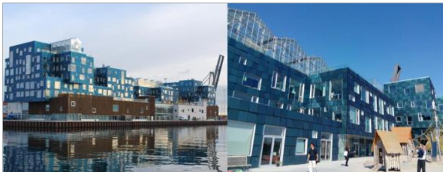
Abbildung 155 -156: International School (Quelle Active House, 2017; 2017a: online)
