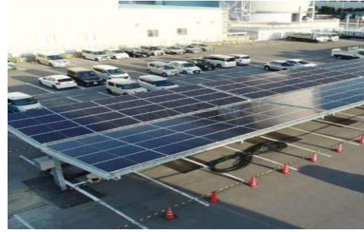
Figure 16: Carbon steel mounting structure PV canopy. Source: (KSENG, 2024)
