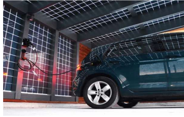
Figure 26: EV charging infrastructure on PV carport. Source: (Stumbraite, 2024)
