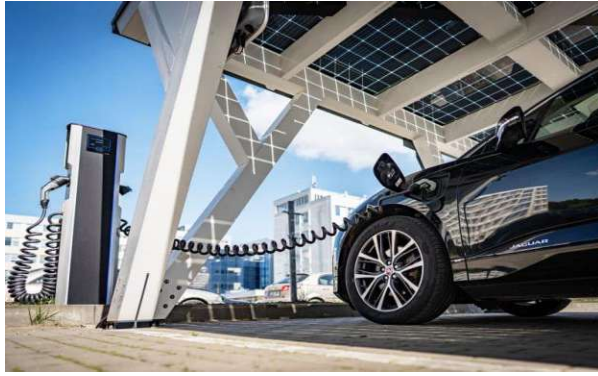
Figure 26: EV charging infrastructure on PV carport. Source: (Stumbraite, 2024)
