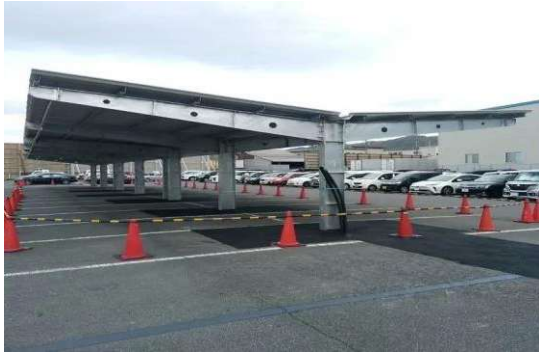
Figure 16: Carbon steel mounting structure PV canopy. Source: (KSENG, 2024)
