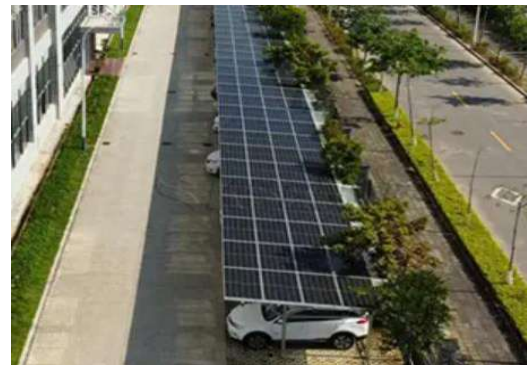
Figure 17: Aluminium mounting structure PV canopy. Source: (KSENG, 2024)
