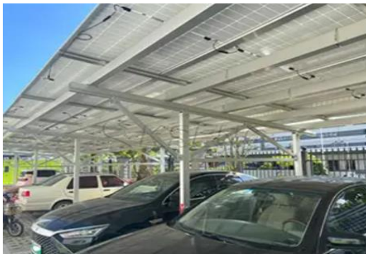
Figure 17: Aluminium mounting structure PV canopy. Source: (KSENG, 2024)
