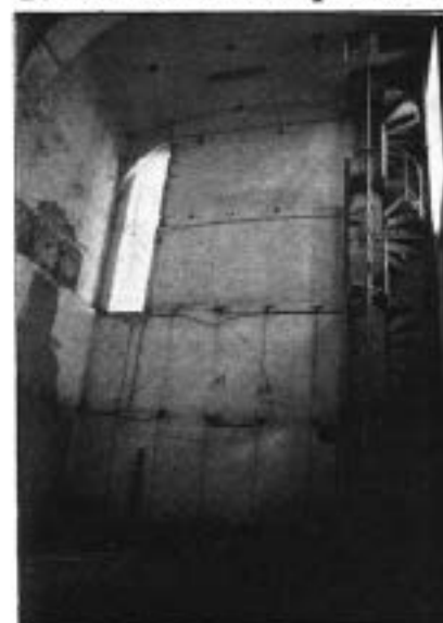
2. Former library rooms
