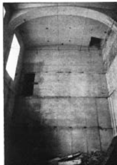
1. Former library rooms
