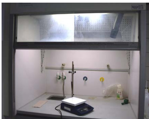
Figure 30 The room with a fume hood in it.
