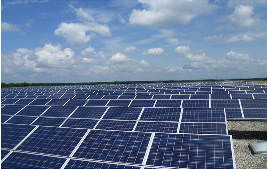
Abb. 9.9: Installation von Photovoltaik-Paneelen
