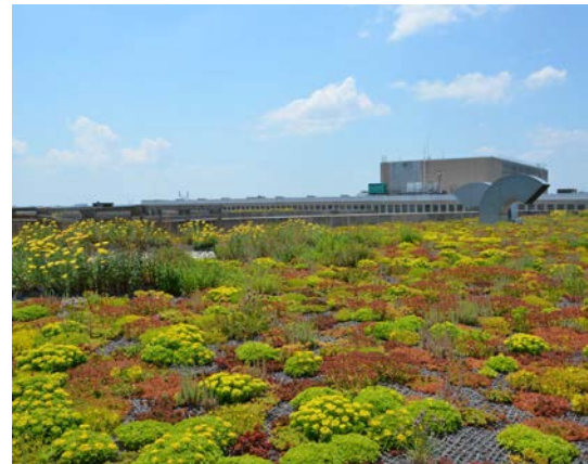
Figure 9 - Extensive green roof (photo: www.sftool.gov )
