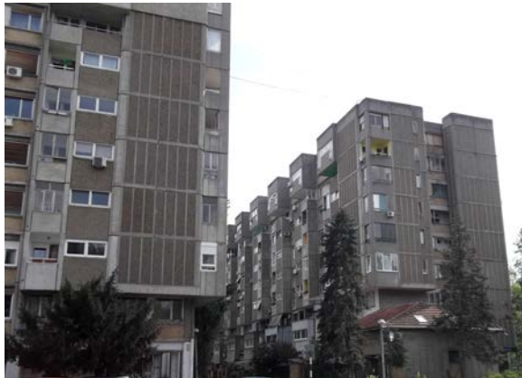
Figure 26 - Residential buildings built in NS-71 system Figure 27 - Facade detail of NS-71 system
