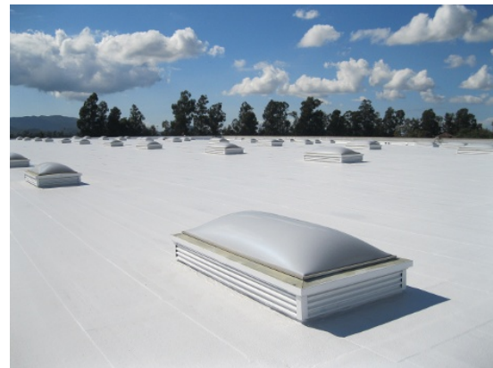
Figure 15 - White roof coating (photo: http://www.nationalcoatings.com/ )
