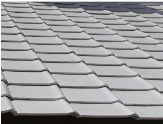
Figure 14 - White roof tiles (photo: http://www.tettogresusa.com/ )
