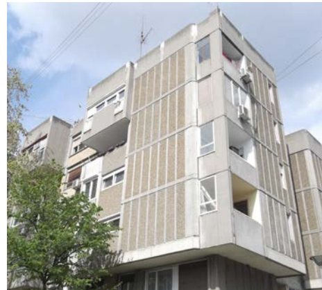
Figure 26 - Residential buildings built in NS-71 system Figure 27 - Facade detail of NS-71 system
