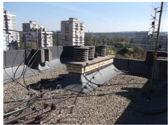
Figure 32 - Roof over corridor
