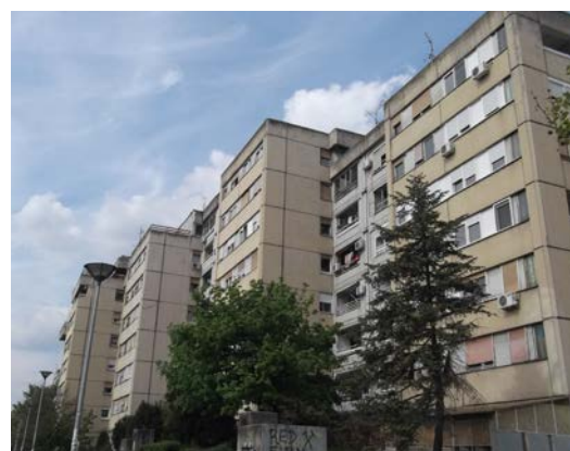
Figure 23 - Residential building built in the IMS system in the 1970s
