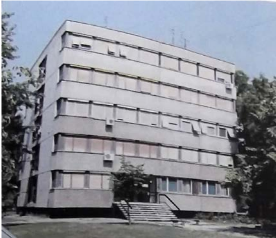
Figure 34 - Residential building IMS NS-1 (photo: M. Laban, 2012)
