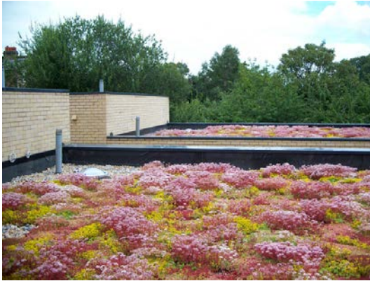
Figure 11 - Sedums on extensive green roof (photo: www.green-roofing.co.uk )
