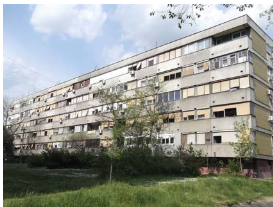
Figure 22 - Residential building built in the IMS system in the 1960s
