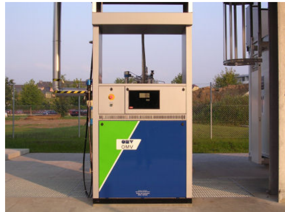
Figure 6.3: Fuel dispenser at Hycent Hydrogen Center, Austria [3]
