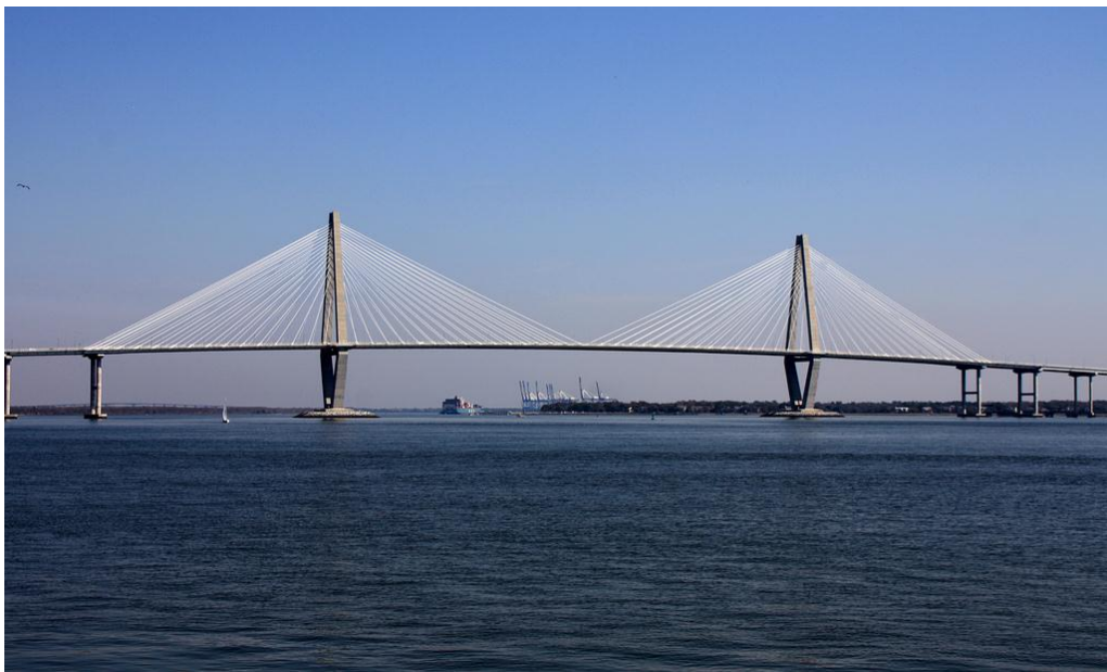
Abb. 1: Arthur Ravenel jr. Bridge in South Carolina [Tin09]
