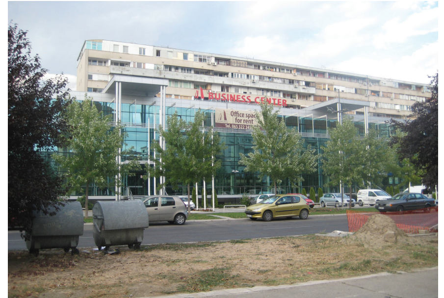
Fig. 51 A new Business Centre on formerly open green space next to apartment-building, 2012
