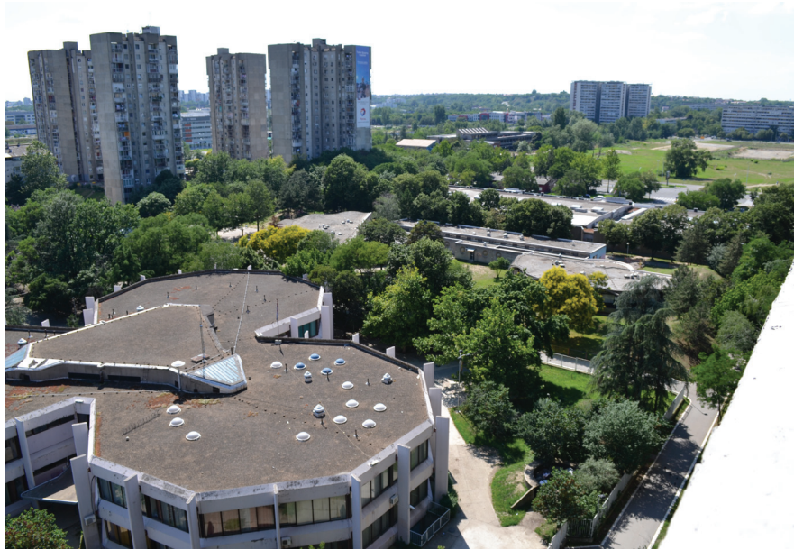
Fig. 53 View from roof-top over Block 28, 2013
