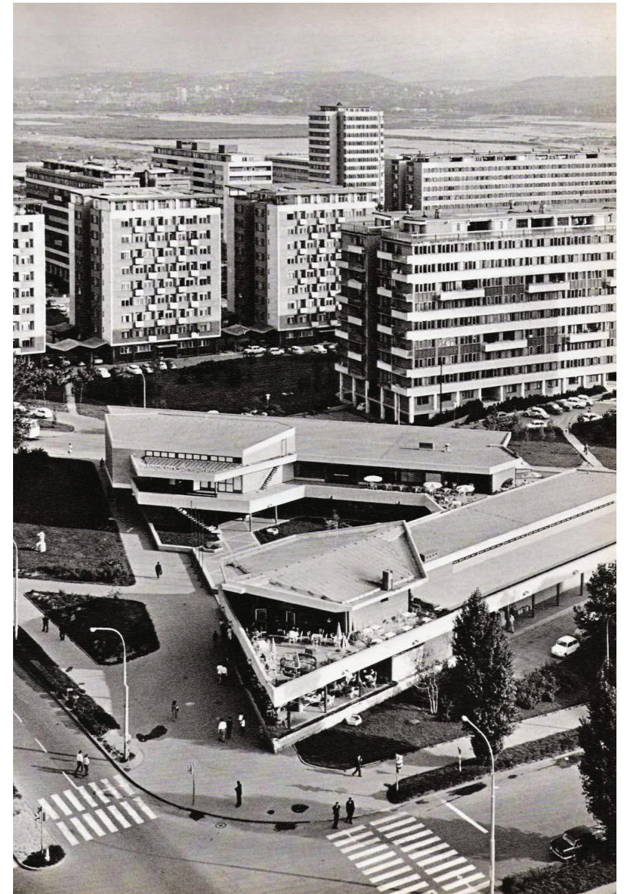
Fig. 37 Local Community Centre ‘25th of May’ with Cinema ‘ Fontana ’, around 1970
