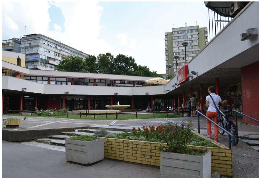
Fig. 49 'Local Community Centre and Cinema 'Fontana' in Block 1, 2013 after renovation
