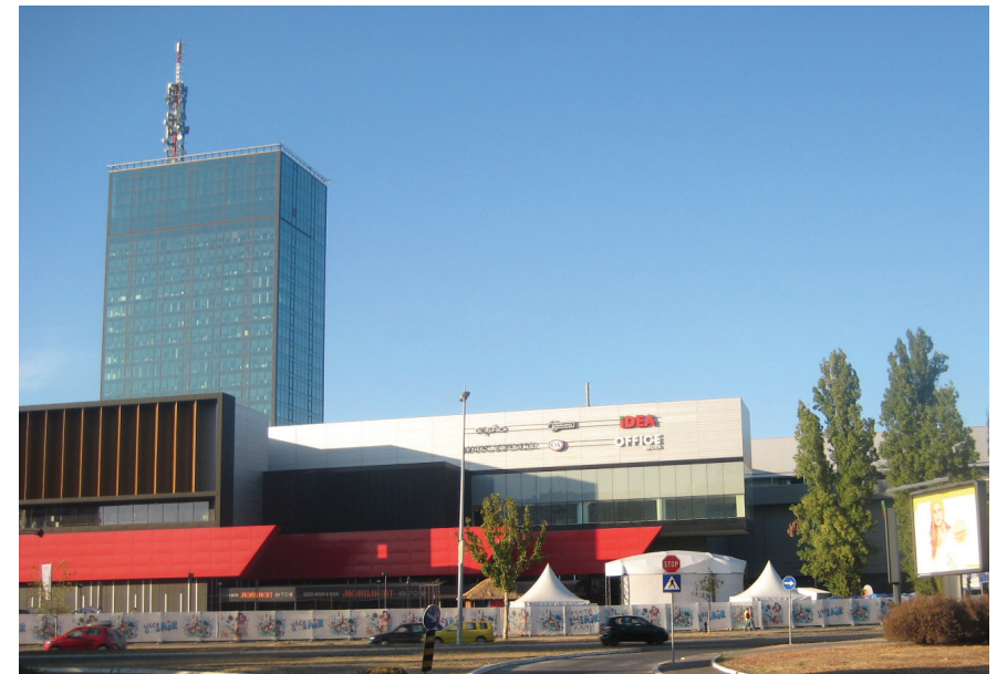
Fig. 56 Former CK-Tower (Building of Political and Social Organisations), Ušće -Shopping Mall
