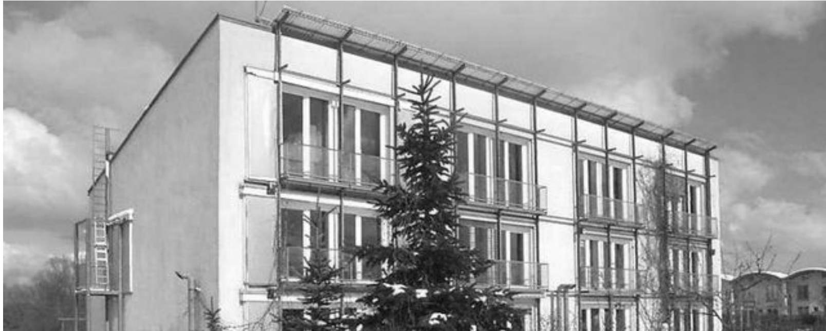
Building based on the passive house concept in Darmstadt, Germany. © Passivhaus Institut
