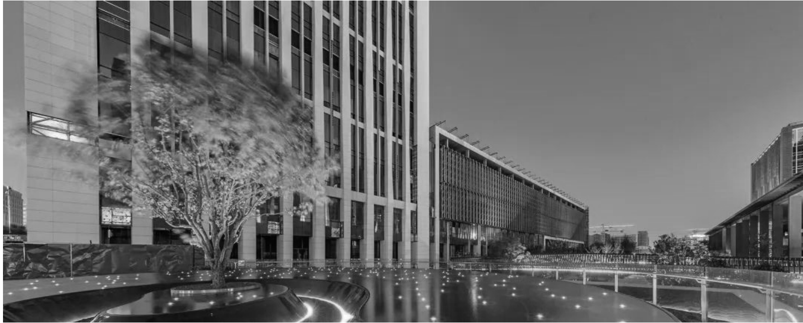
The CFLD Feng Tai Science Park in Beijing, achieved LEED Gold for Core and Shell. © Haozhen Pan
