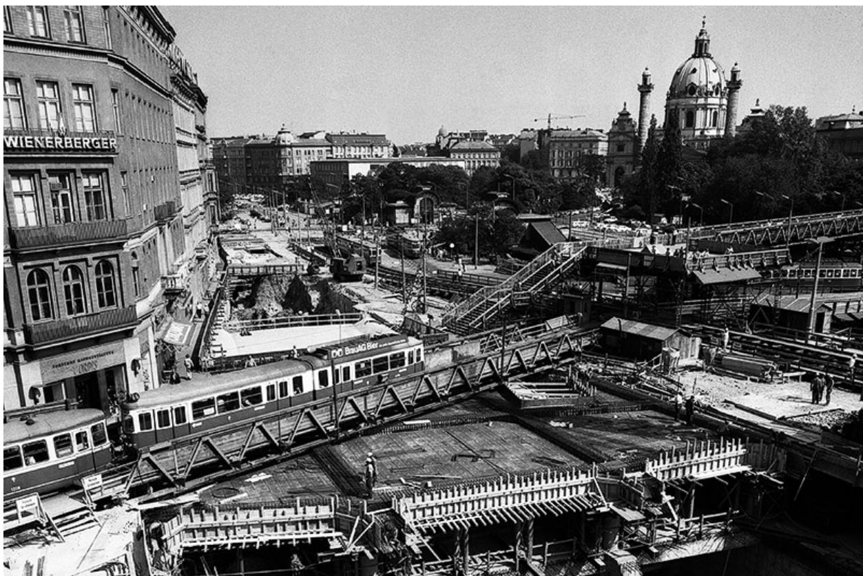
Fig.49 Photo of the railway building site from 1969.
