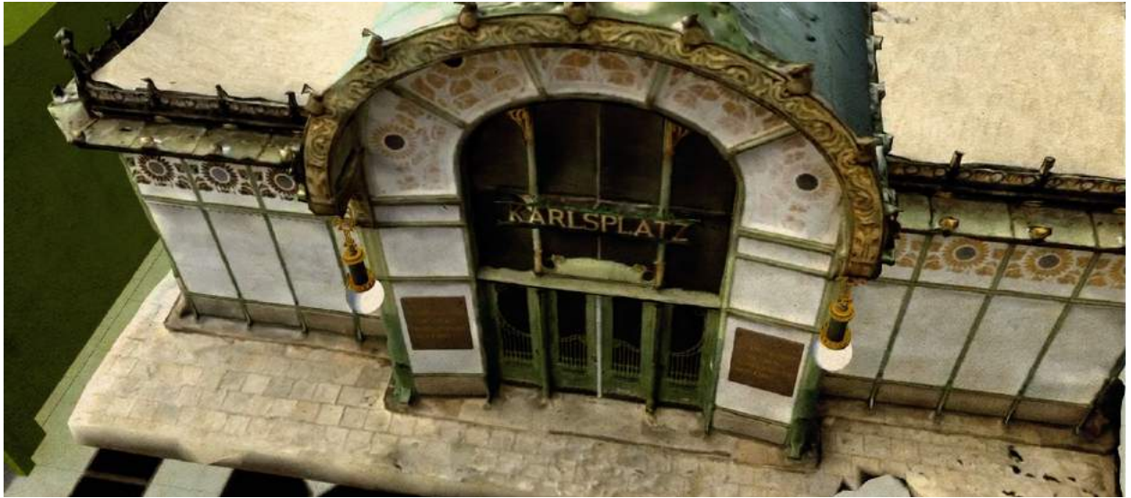
Fig.125 Original parts, lamps and plaques missing in actual state.
