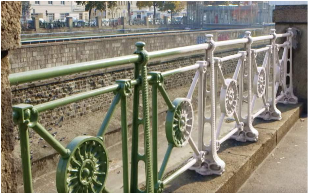
Fig.41 The original colour next to the current green coloured railing, photo from document Otto Wagner - Visionär der Moderne Doku (2017).
