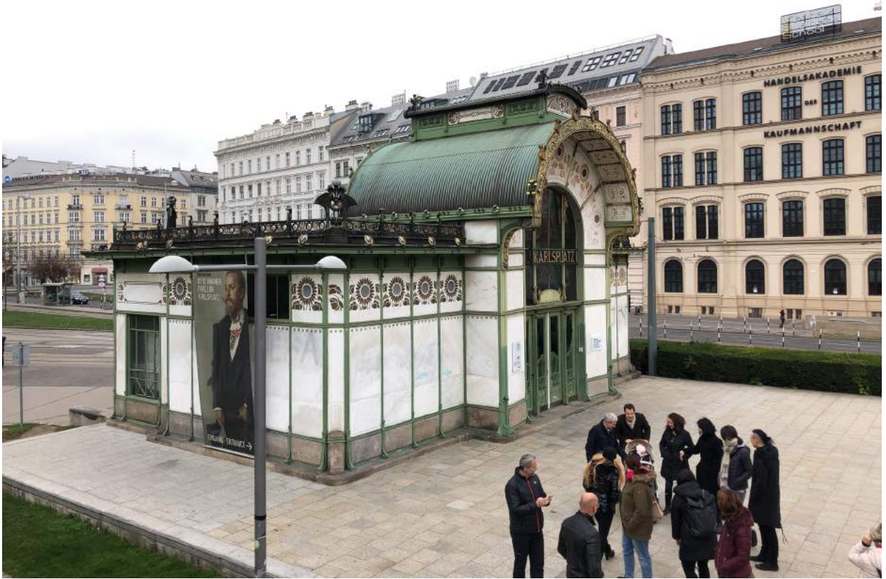
Fig.83 Input photo taken with the inspection pole.
