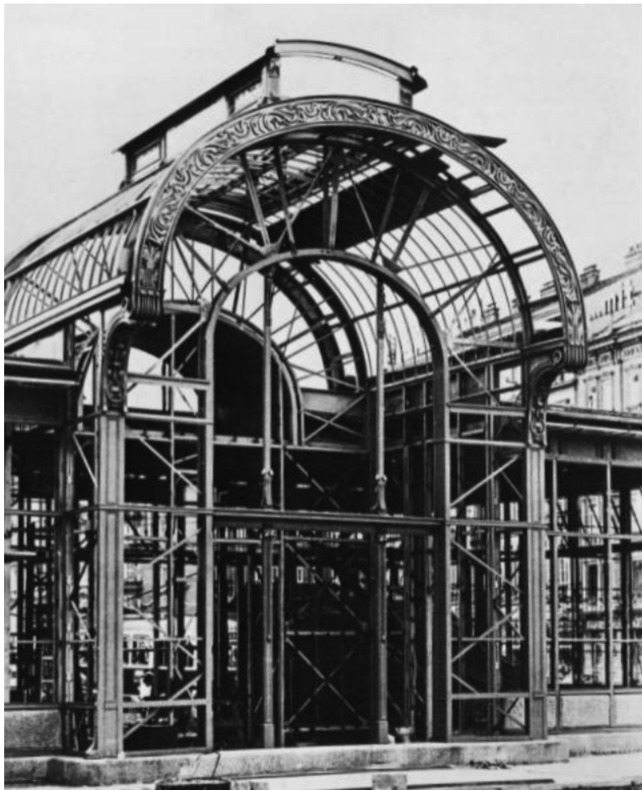
Fig.50 Karlsplatz Pavilion during reassembling, 1977.
