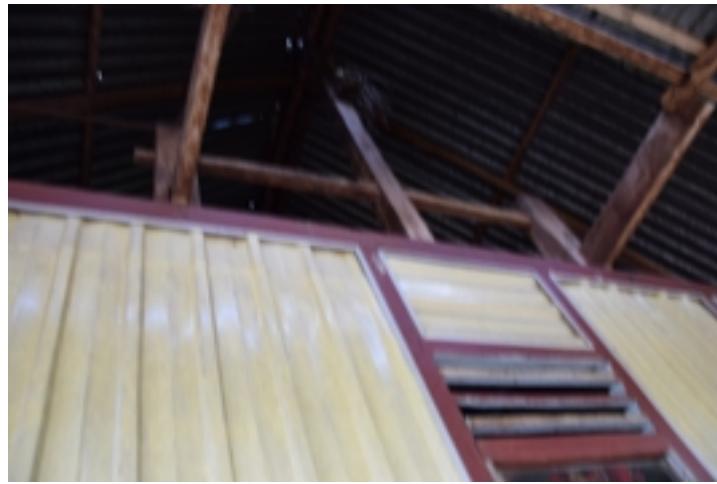
Figure 5.81: Z1-BT-01 : Pole direct from ground to roof. Source : Field survey 2015
