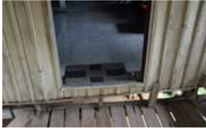
Figure 4.8: applying flat floor on watangpola and tamping but floor of lego-lego low slightly. Source : Field survey 2015
