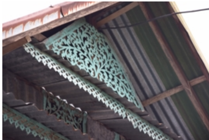
Figure 5.183: Z2-BT-33 : Detailed ornamental wood carving on the gable wall. Source : Field survey 2015
