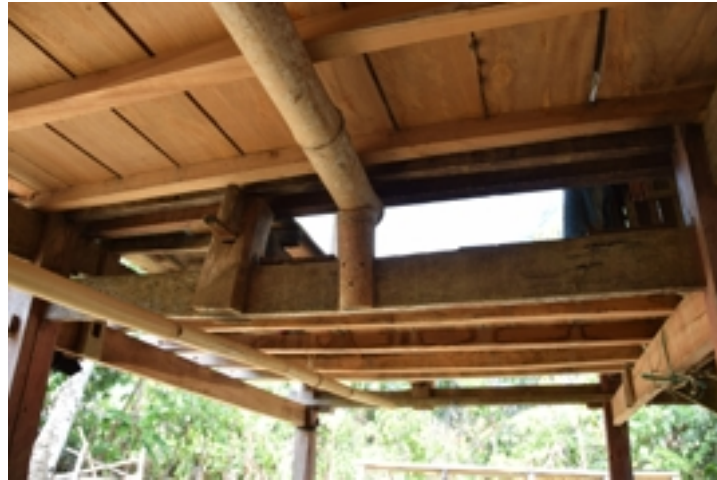
Figure 5.72: Z1-PL-33 : lego-lego and tamping floor construction. Source : Field survey 2015
