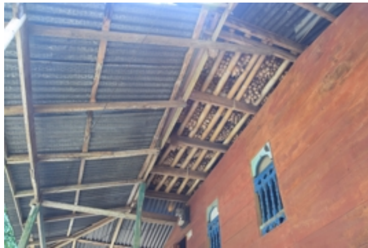
Figure 5.147: Z1-BN-36 : lego-lego roof construction. Source : Field survey 2015
