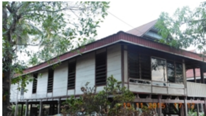
Figure 5.36: Z1-PR-28 : : Front and side jalousie windows Source : Field survey 2015
