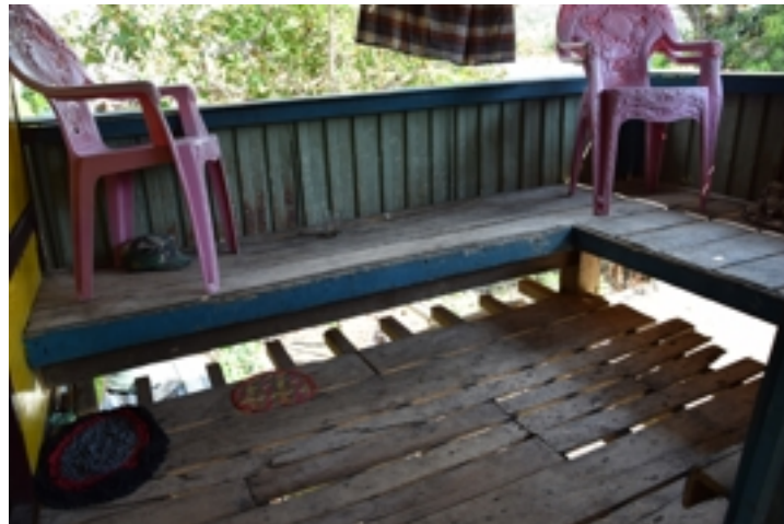
Figure 5.412: Z3-BL-21 : lego-lego floor Source : Field survey 2015
