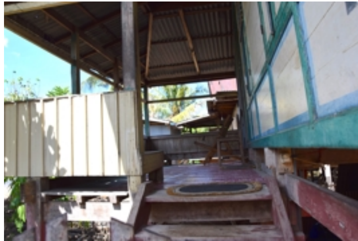
Figure 4.62: lego-lego floor is slightly lower than floor of the main house. Source : field survey 2015
