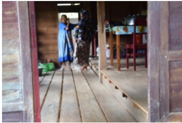
Figure 5.61: Z1-PL-30 : tamping floor at its original position i.e. lower than the watanpola floor. Source : Field survey 2015
