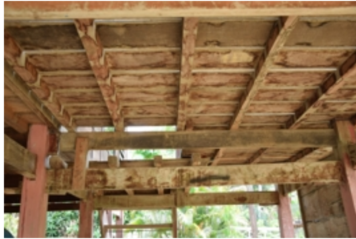
Figure 5.68: Z2-PL-32 : lego-lego floor construction..Source : Field survey 2015
