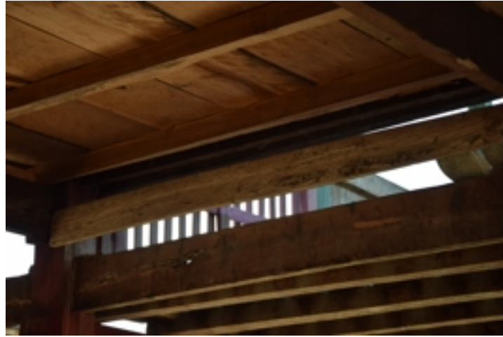
Figure 5.90: Z1-TT-06 : floor contruction between tamping and lego-lego . Source : Field survey 2015
