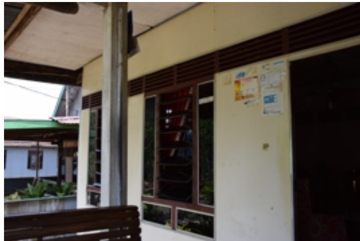
Figure 5.84: Z1-TT-05 : Jalousie window surrounded by plate glass inserts and open doorway Source : Field survey 2015
