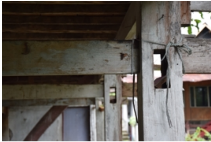
Figure 5.179: Z2-BL-33 : Figure 5.179: Z2-BL-33 : Empty holes showing the original floor level of the old style tamping . Source : Field survey 2015
