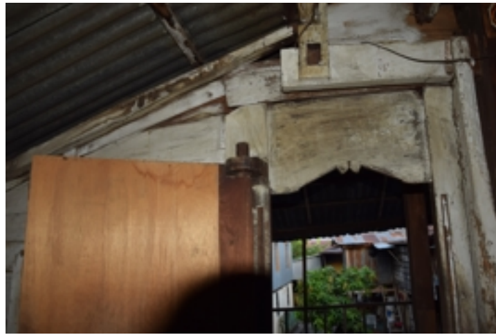
Figure 5.222: Z2-PA-17 : Old style hinge. Source : Field survey 2015
