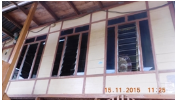
Figure 5.109: Z1-PR-15 : Jalousie windows with plate glass leaves installed across the top and at either side. . Source : Field survey 2015
