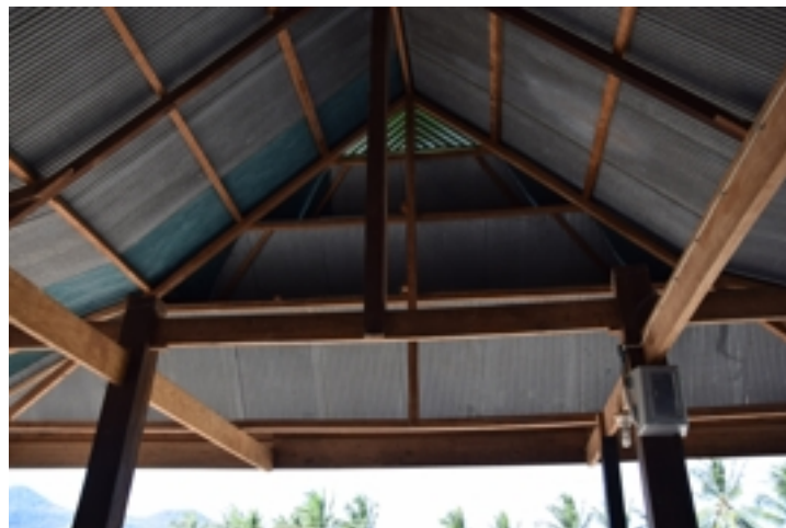
Figure 5.451: Z3-BL-24 : timplaja construction Source : Field survey 2015
