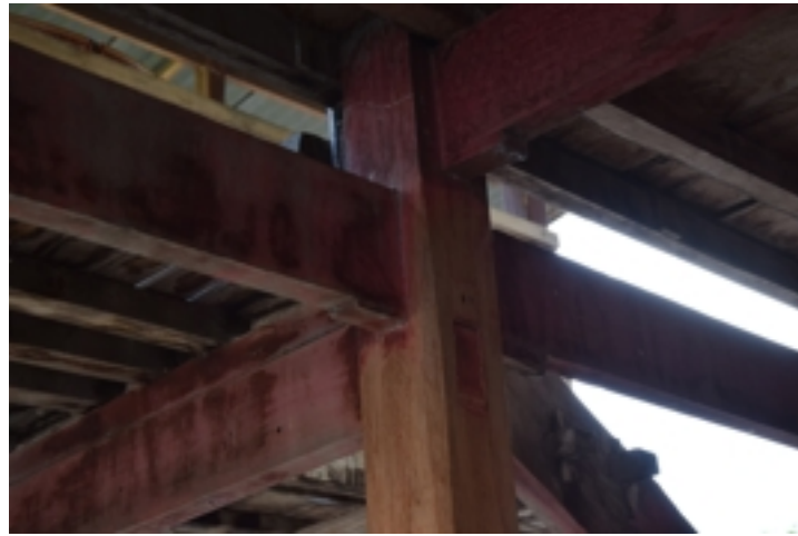
Figure 5.261: Z2-PA-19 : Support beam for the staircase. Source : Field survey 2015
