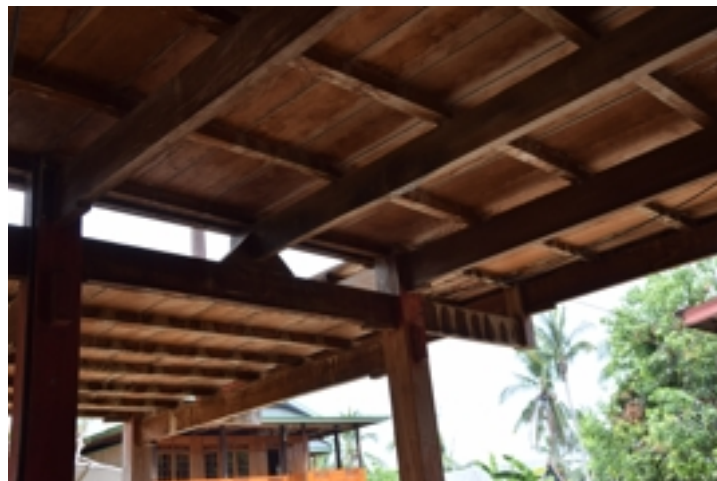
Figure 5.64: Z1-PL-31 : Floor construction. Source : Field survey 2015
