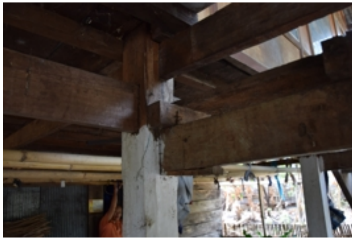
Figure 5.104: Z1-PR-11 : Connection of the pole and beams. Source : Field survey 2015
