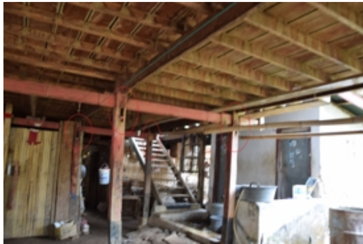
Figure 5.51: Z1-TT-04 : Hole in post showing the original tamping floor level. Source : Field survey 2015
