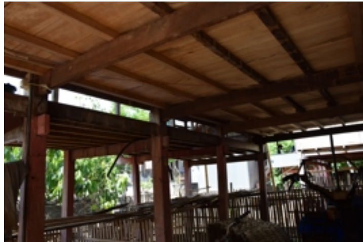
Figure 5.56: Z1-TT-07 : Floor construction. Source : Field survey 2015
