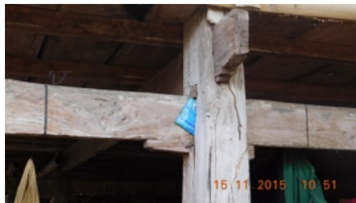
Figure 5.114: Z1-PR-12 : Connection between pole and beams. Source : Field survey 2015
