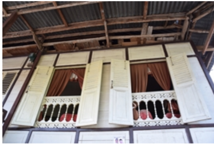
Figure 5.361: Z3-TJ-01 : Malay style windows with shutters and five spindles.
