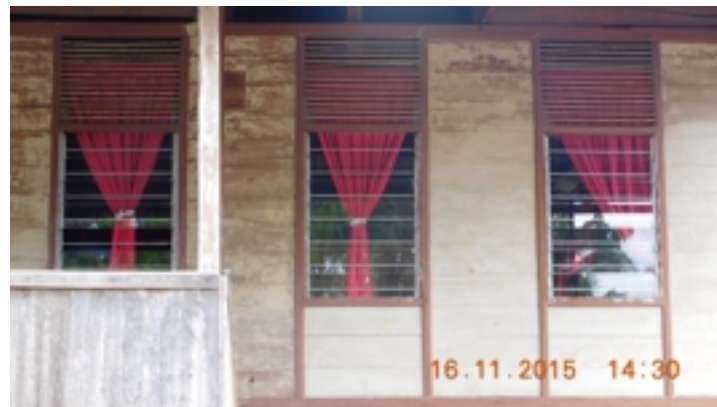
Figure 5.129: Z1-TL-23 : Glass jalousie windows - each with fixed wooden slats above. . Source : Field survey 2015
