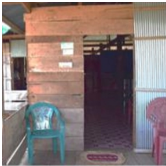
Figure 4.61: New style door where the floors inside and outside are flush with the door sill. Source : Result of survey 2015
