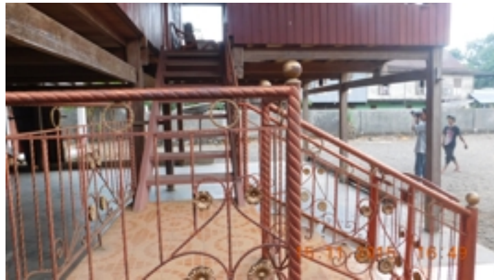
Figure 5.44: Z1-JS-27 : Stairs with tuka (landing) and a modern metal bannister and balustrade. Source : Field survey 2015
