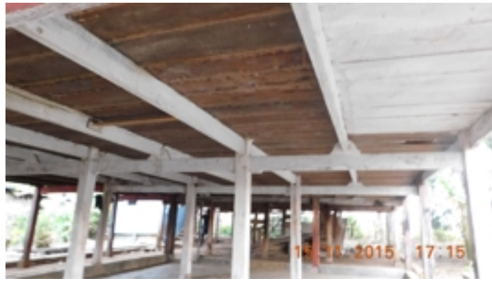
Figure 5.38: Z1-PR-28 : : Floor beams of an old style of a noble's house. Source : Field survey 2015
