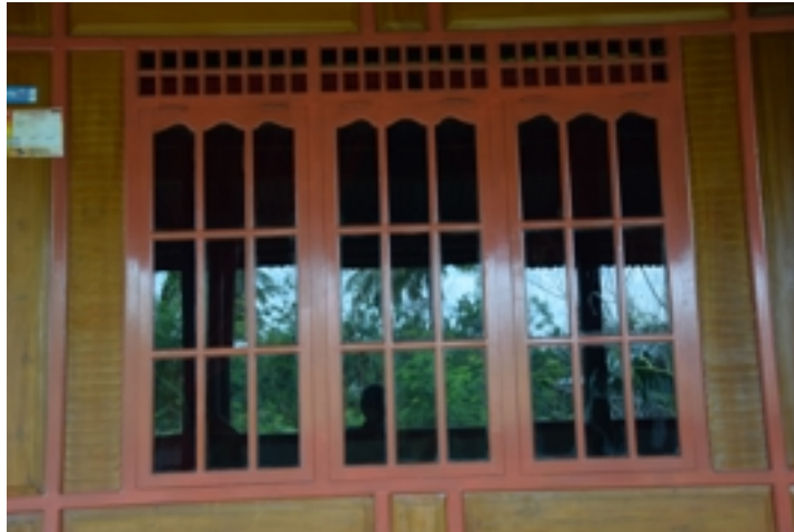
Figure 5.172: Z1-PR-17 : Triple wood frame window with plate glass with wood grill along the top. Source : Field survey 2015
