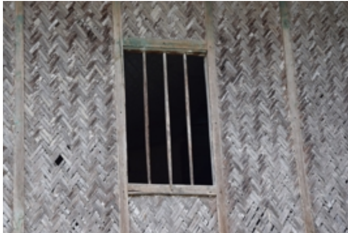
Figure 4.46: Bugis traditional window with three simple bars on a commoner's house. Source : Field survey 2015
