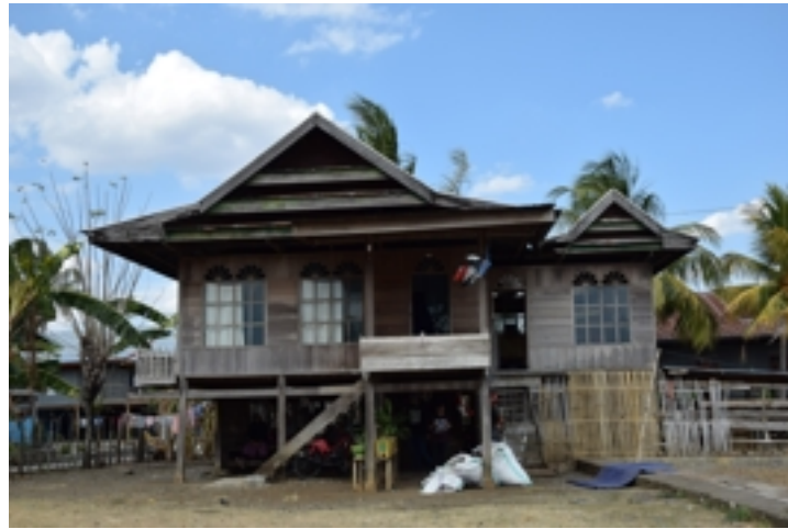
Figure 5.40: Z1-TL-22 : Façade with three timplaja . Source : Field survey 2015
