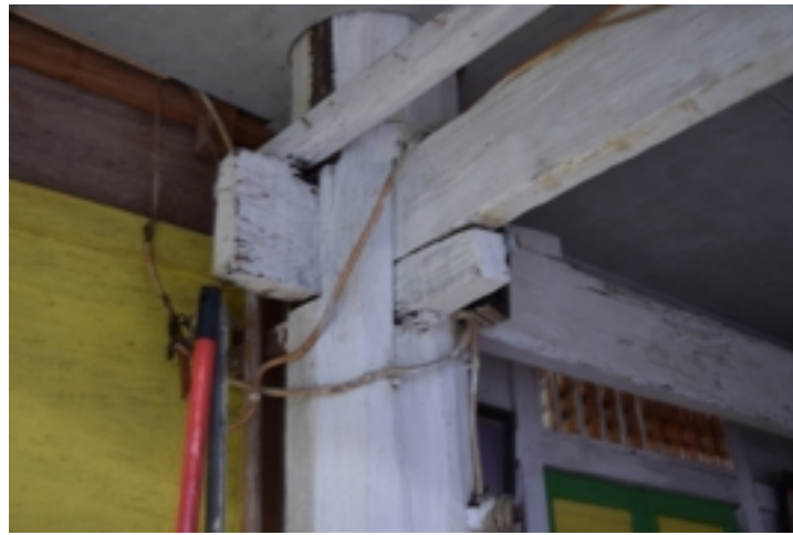
Figure 5.328: Z3-BT-26 : Circular pole and rectangular beams. Source : Field survey 2015
