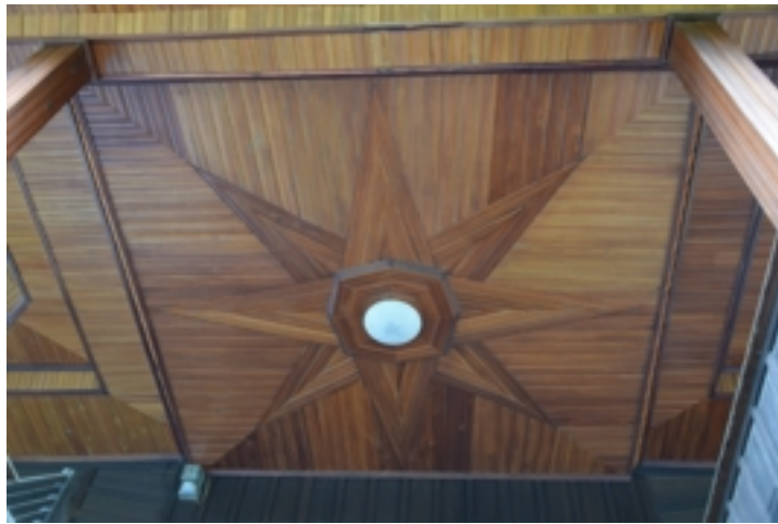
Figure 5.357: Z3-TJ-17: Parquet ceiling. Field survey 2015
