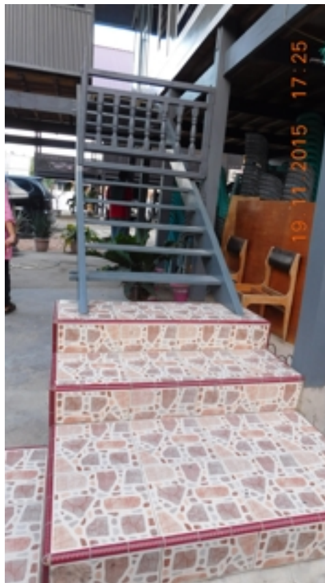
Figure 5.317: Z2-PA-29 :Stairs partially of ceramic and partially of wood.. Source : Field survey 2015
