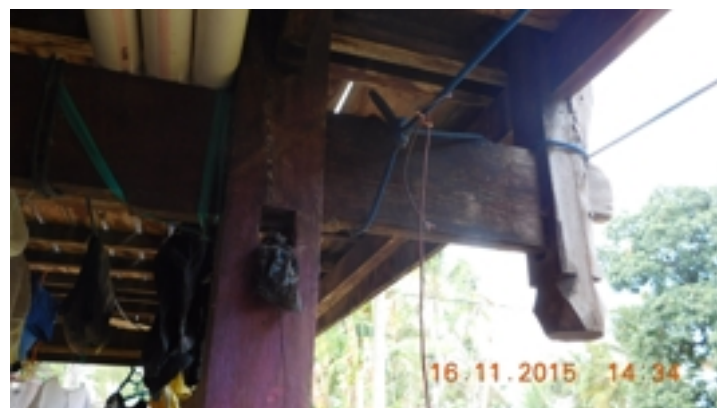
Figure 5.130: Z1-TL-23 : Former hole used for the original tamping floor. Source : Field survey 2015
