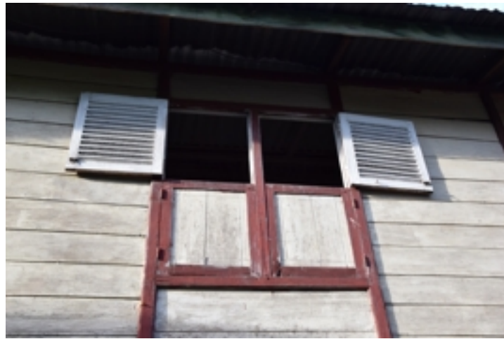
Figure 5.281: Z2-PA-23 : : Shuttered window with jalousie (fixed wooden slats) on top and wooden boards below. Source : Field survey 2015
