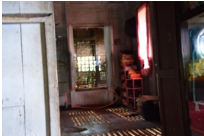
Figure 5.339: kappa-kappang under door between main house and kitchen house. Source Field survey 2015
