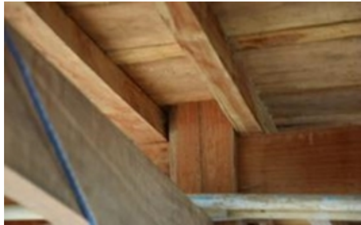
Figure 4.77: Placement of the floor beam must be tight to the pole to prevent thieves from entering the house. Source : Field survey 2015
