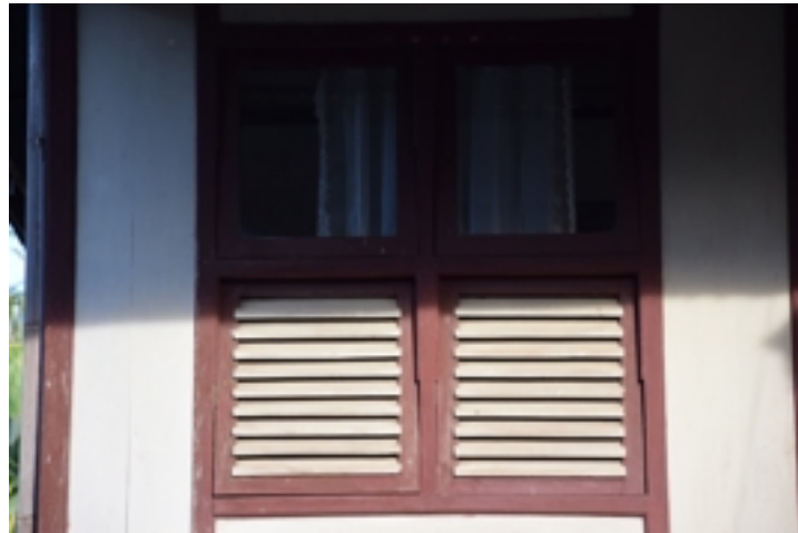
Figure 5.282: Z2-PA-23 : Shuttered window with plate glass on top and jalousie (fixed wooden slats) below. Source : Field survey 2015
