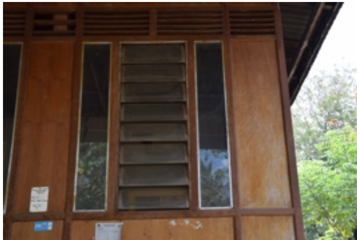
Figure 5.105: Z1-PR-11 : Jalousie window with fixed plate glass leaves on either side.
