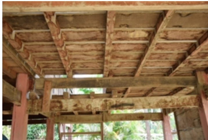
Figure 5.67: Z2-PL-32 : Connection between pole and beams of pattolo and arateng . Source : Field survey 2015
