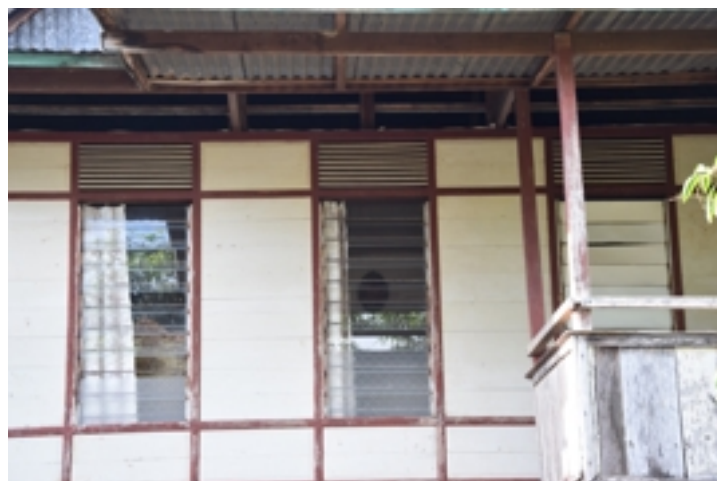
Figure 5.262: Z2-PA-19 : Jalousie windows with wooden slat transoms. Source : Field survey 2015
