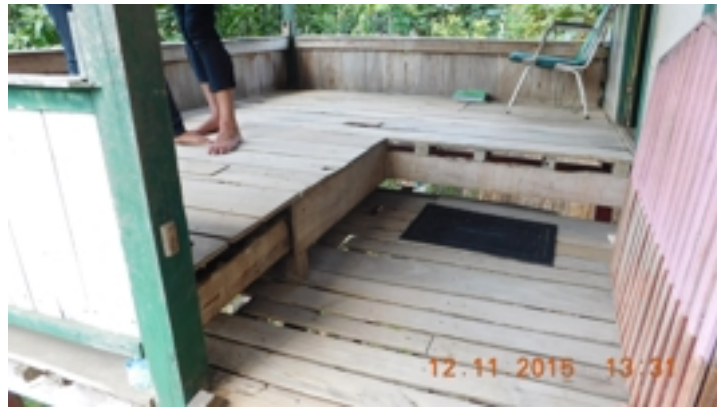
Figure 4.64: lego-lego adopted a two level floor. Source : field survey 2015
