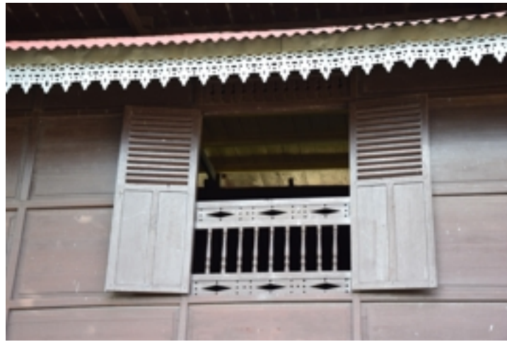
Figure 5.28: The window of Z1-GL-24 uses nine bars.
