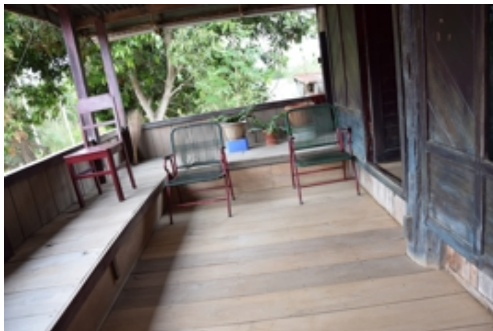
Figure 5.60: Z1-PL-30 : lego-lego with a raised bench and a floor lower than the watangpola floor. Source : Field survey 2015
