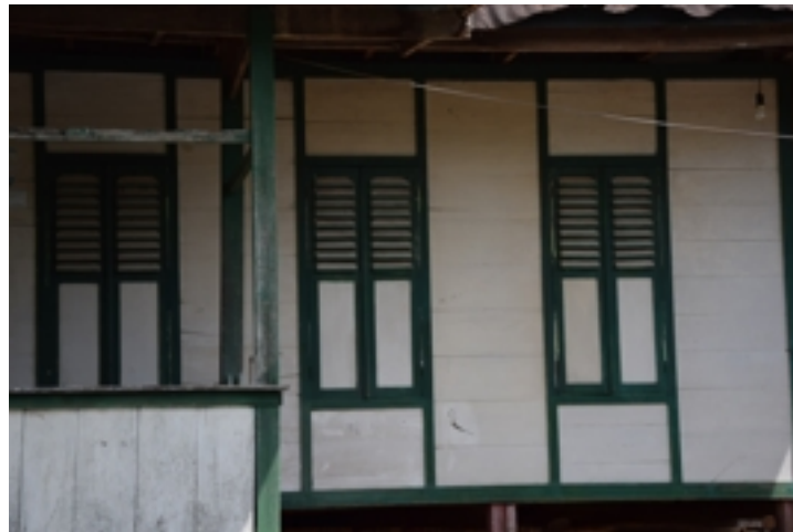
Figure 5.88: Z1-TT-06 : Closed shutters with each using plain boards below the mid rail and fixed slats above in the Malay style : Field survey 2015
