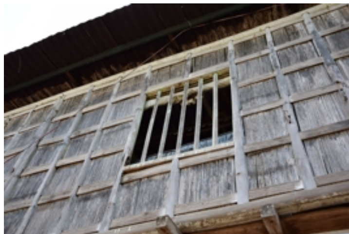
Figure 5.89: Z1-TT-06 : A traditional Bugis window using five bars installed on an exterior bamboo wall. Source: Field survey 2015
