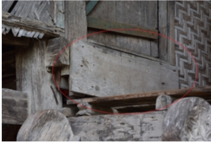
Figure 5.232: Z2-BL-32 : kappa-kappang under the door. Source : Field survey 2015
