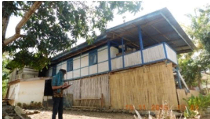
Figure 5.117: Z1-PR-19 : Bamboo wall enclosing wasaubola . Source : Field survey 2015
