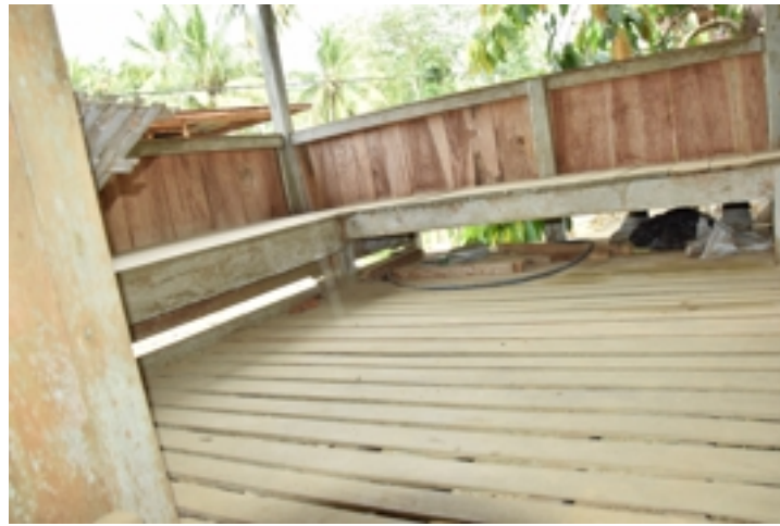
Figure 5.158: Z1-PR-40 : Lego-lego with a built-in bench . Source : Field survey 2017
