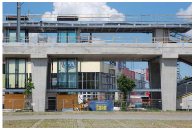
The construction of the tramway line crosses the railway and the motorway as an elevated track, without touching the ground.
