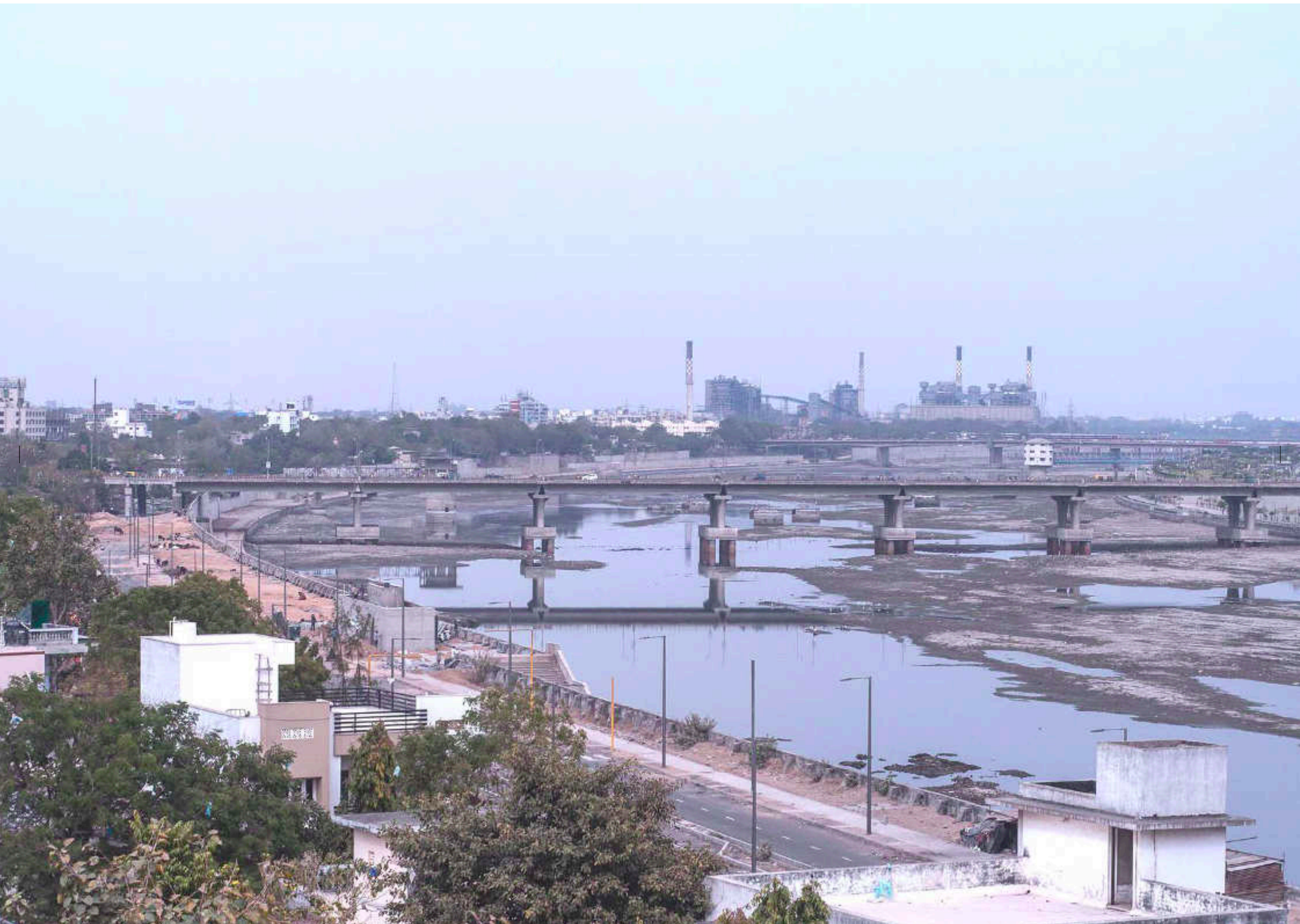
209 Date 21.02.2014; Sabarmati River Front, one of the top goal-developments in Ahmedabad, entirely straightened river banks can cause problems in high rain seasons
