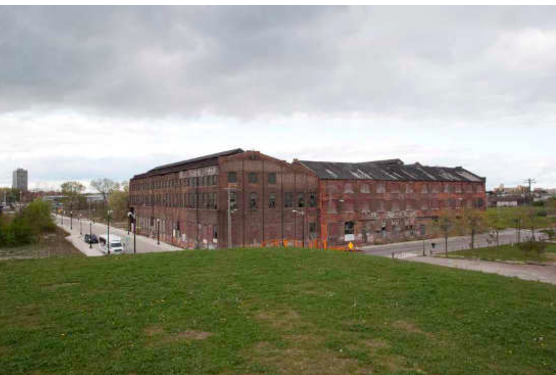
216 Date 26.04.2012; Seemingly at random one comes across vacant buildings, half of this building no longer exists the other half has been renovated, Atwater Street 1801, Detroit
