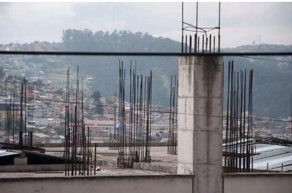
148 Date 22.02.2013; Very common, structural steel for the next story, in- years can pass between phases of building, in the centre of Quito
