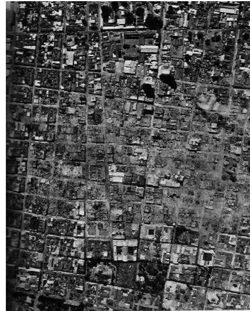
170 Aerial view after the Managua earthquake of 1972,
