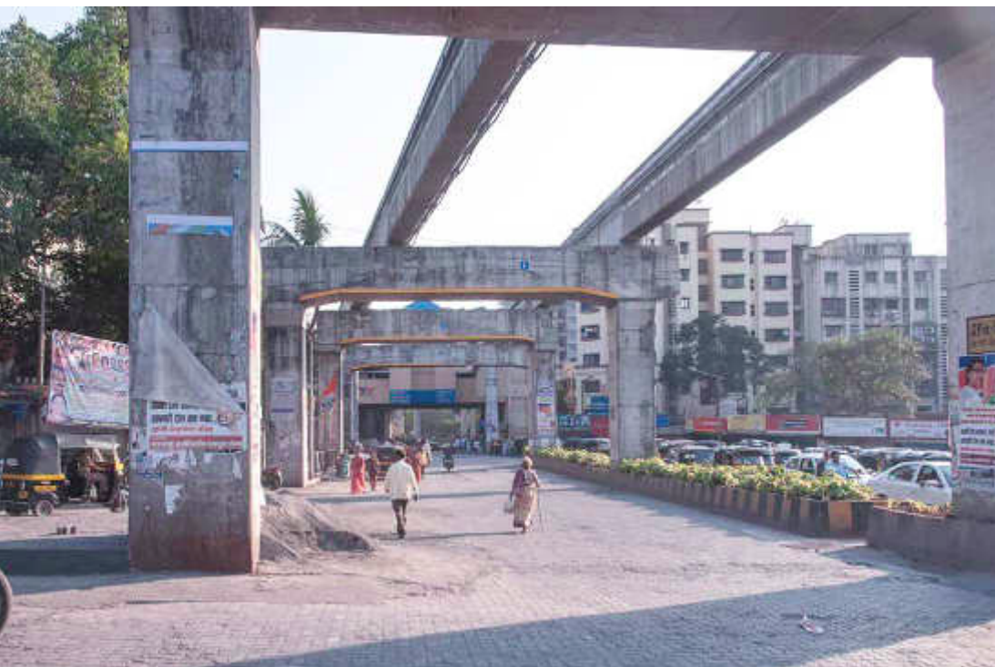
080 Date 17.02.2014 ; Mumbai, Monorail columns, the capacity of this Metro/High-Line might not have enough capacity for the densely populated city of Mumbai
