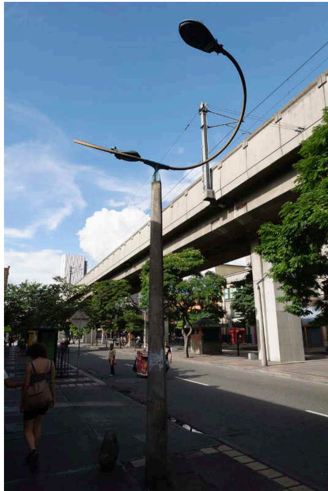
189 Date 21.04.2013, The metro of Medellín, actually a high line
