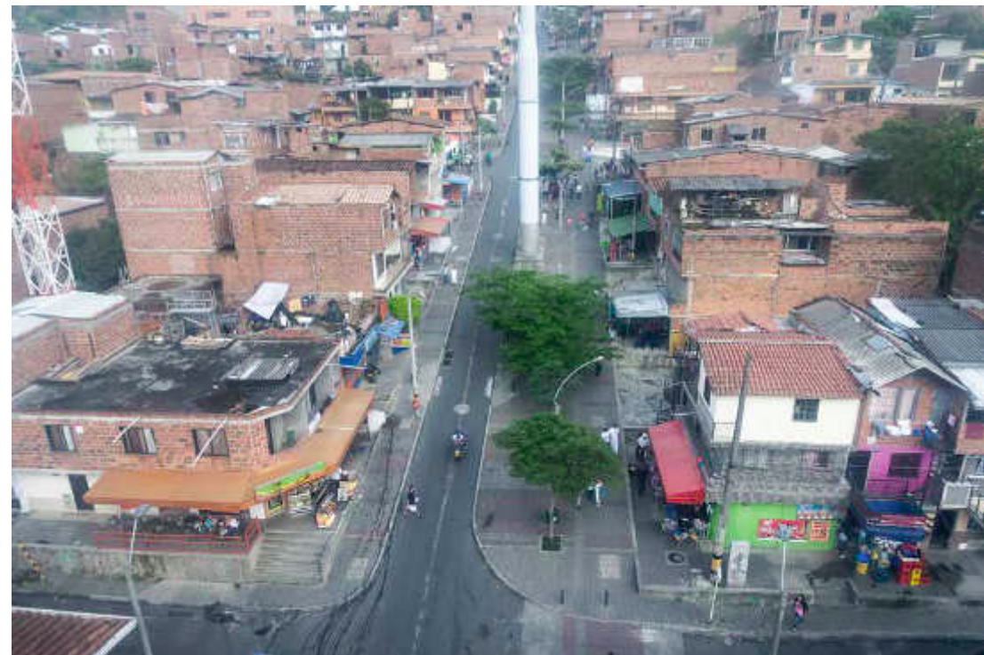
196 Date 21.04.2013; Adaptation of the public space beneath the Metro Cable
