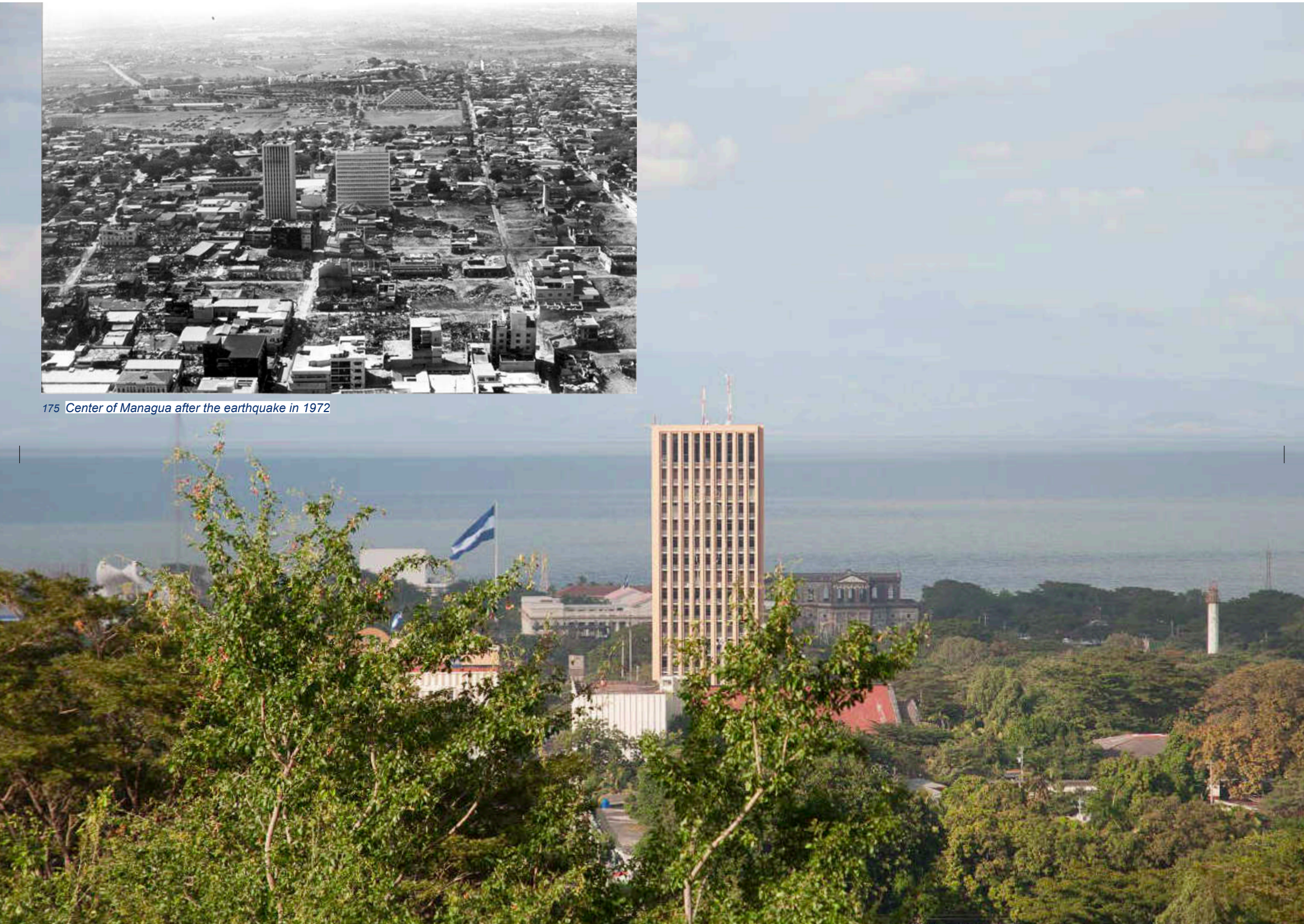
176 Date 11.12.2012; View of buildings which endured the earthquake of 1972, In the centre, the former Bank of America building built in the 60's cracked but did not collapse, statics by Lin Tung Yen, Managua
