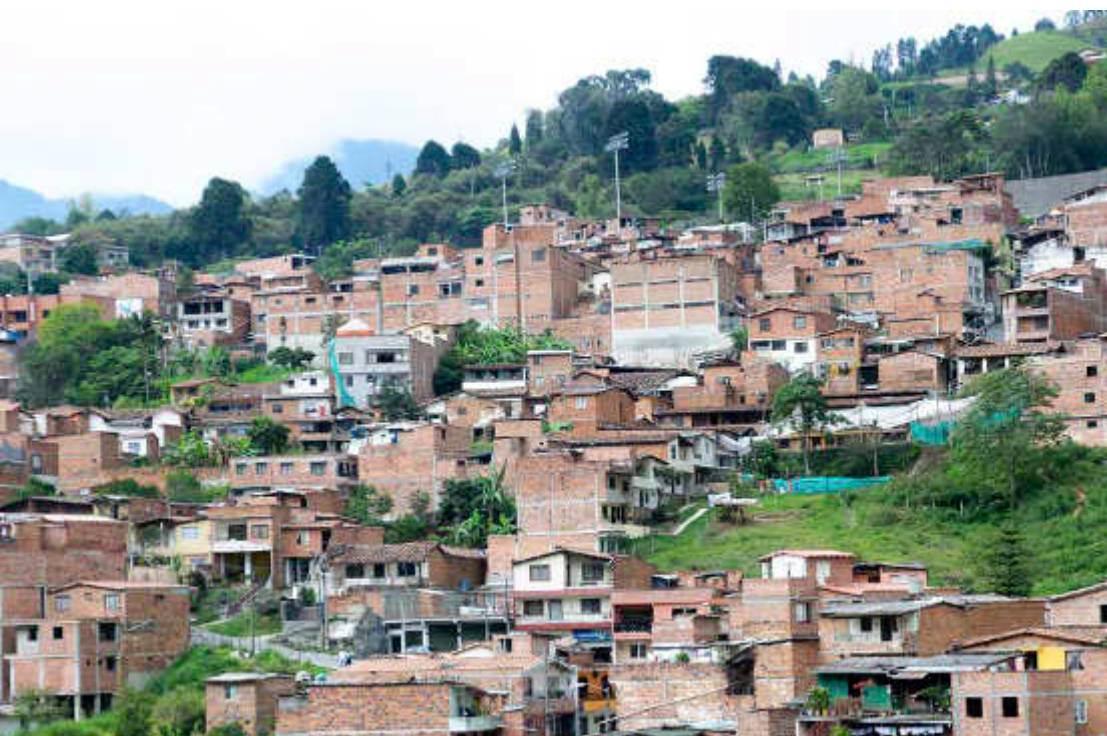
188 Date 22.04.2013; Seen from the "Metro-Cable" station Santo Domingo Savio, Medellín
