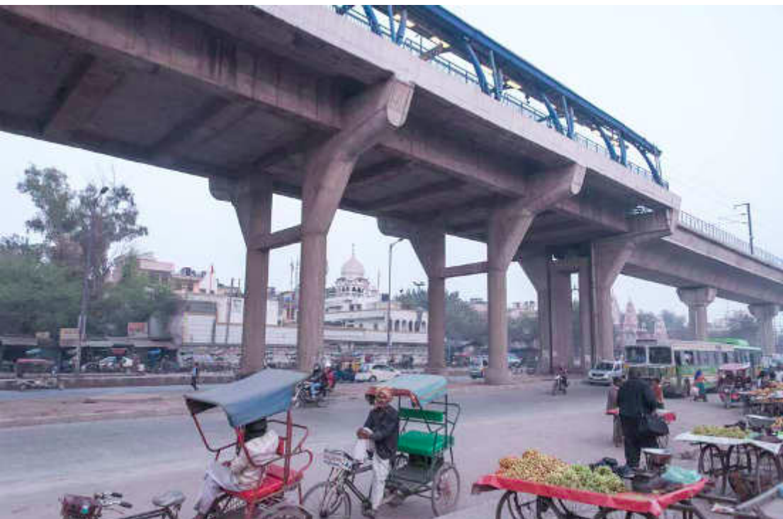
106 Date 23.02.2014; New Delhi, raised subway station
