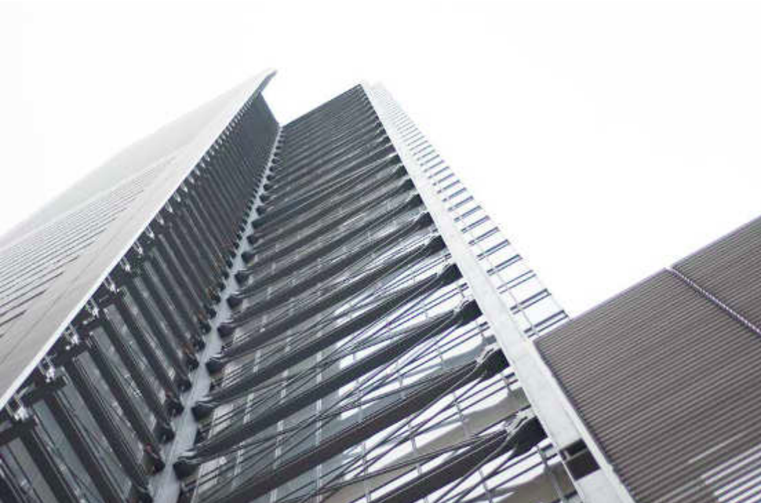
061 Date 15.10.2012; Detailed, balanced and sustainable architecture in the Times-square district, New York Times Tower, opened 2007, Design by Renzo Piano
