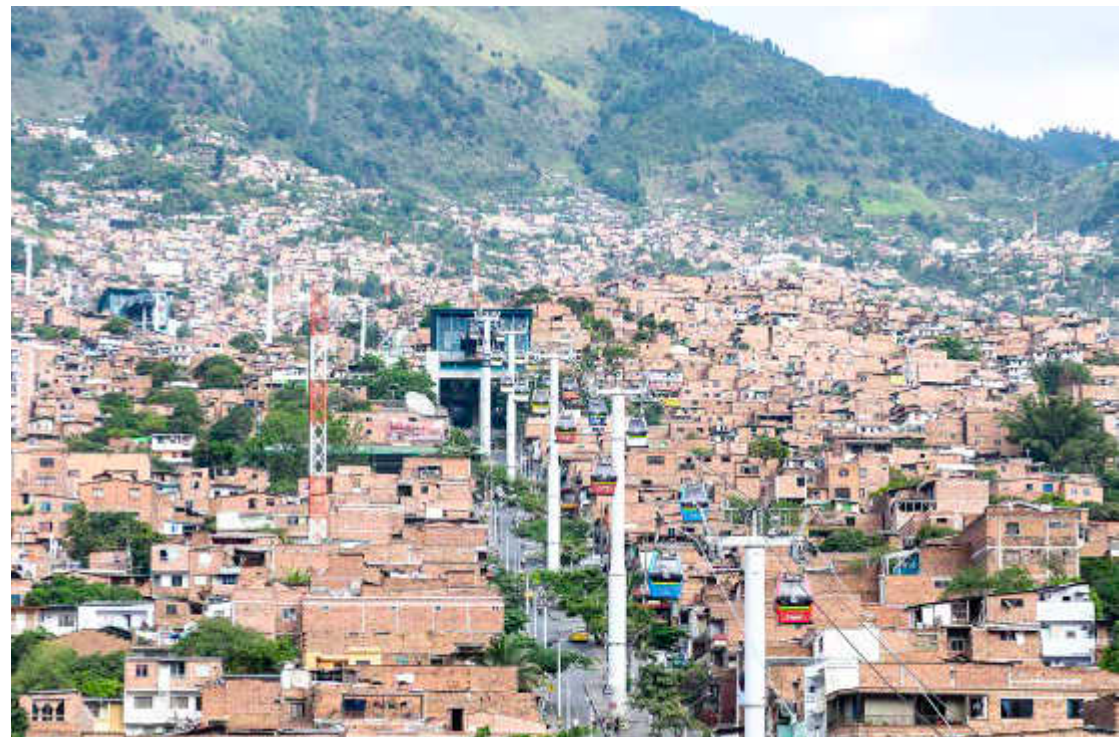
192 Date 21.04.2013; Metro Cable Linea K, gondolas and pillars
