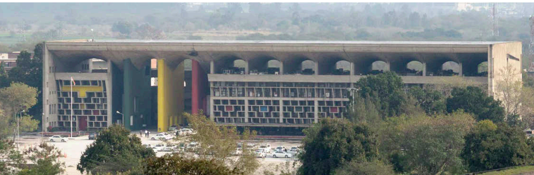
095 Date 28.02.2014; High Court Chandigarh, design by Le Corbusier
