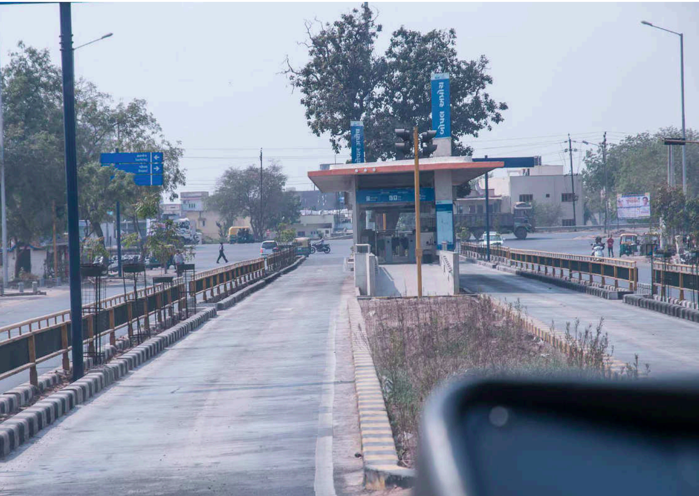
208 Date 20.02.2014; A bus stop and the separated bus line of the Janmarg or BRTS Ahmedabad, Bus Rapid Transit, first operated in 2009, running some 160 buses by now
