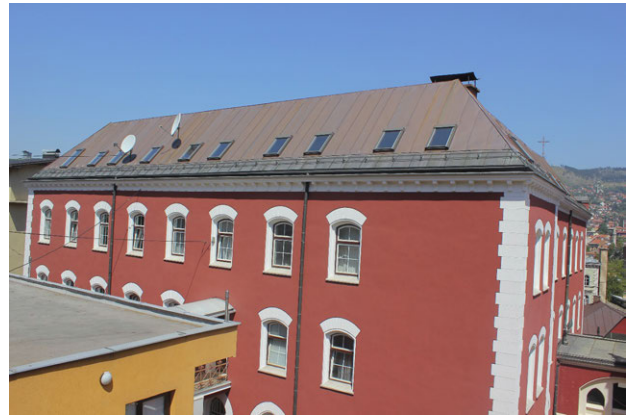
Figure A.16 The Convent of Saint Anthony of Padua, Bistrik: view of the south-western corner from the southern terrace above the complex (2013)
