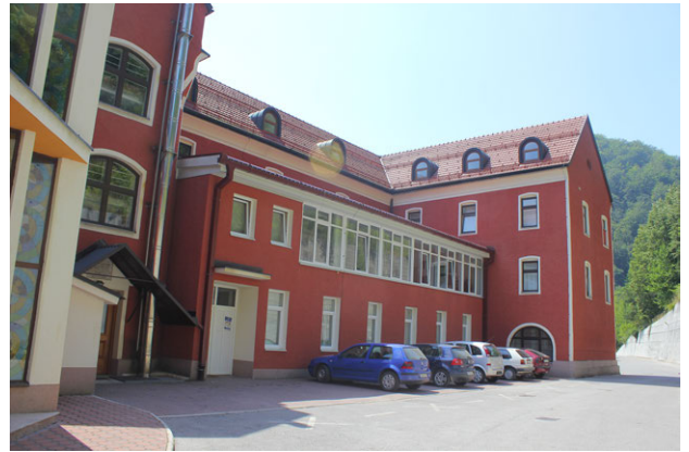
Figure A.150 The Convent of Saint Catherine: view of the northern façade, with the entrance on the far left (2013)
