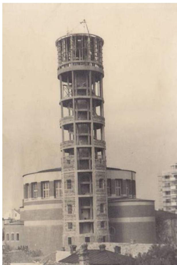
Figure 165 The Parish Church of Saint Anthony of Padua: bell-tower during the construction (Private archive)
