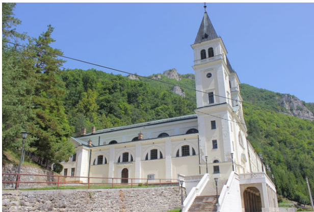
Figure 142 The Parish Church of Saint John the Baptist, Kraljeva Sutjeska: view from the west (2013)
