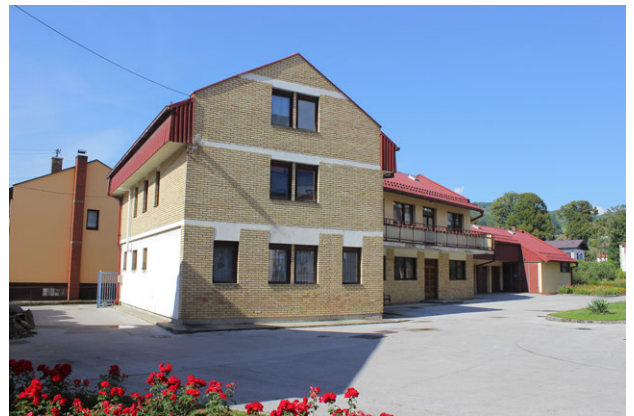
Figure A.278 Nuns' house: view from the south (2013)
