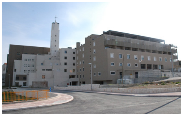
Figure 94 The Franciscan clericate of Friar Ante Antić, Split: completed in 2007, according to project done by Jerko Rošin ("Samostan – Trstenik")
