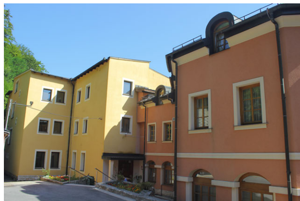
Figure 109 The Convent of the Holy Spirit, Fojnica: view of the link between the first and second wing from the inner courtyard, on the left, wing built by Franjo Lavrenčić in 1940, on the right re-built building of the first wing, built in 2001 (2013)
