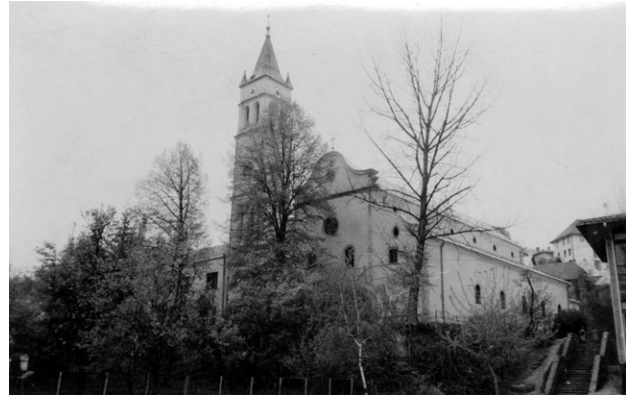
Figure A.132 The Parish Church of the Assumption of the Blessed Virgin Mary, Jajce: view of the main façade from the east; photograph taken before 1991 (Archive Tolisa)
