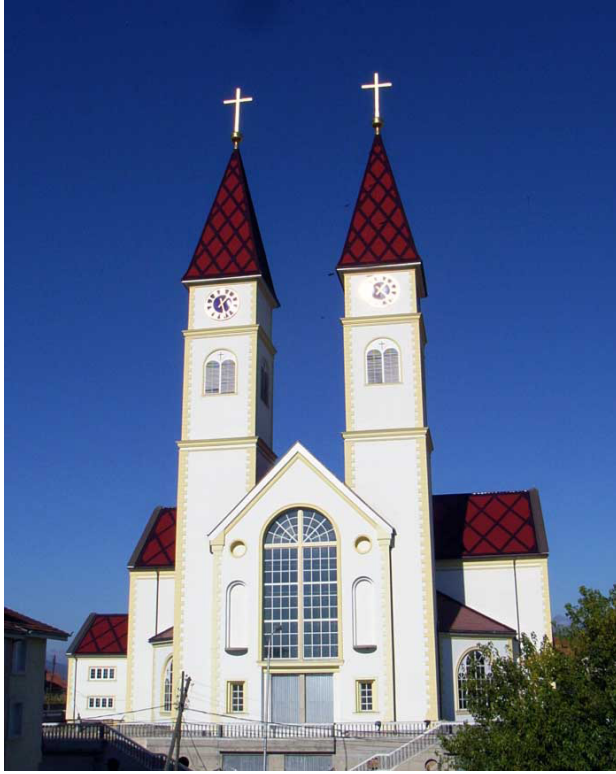
Figure A.65 The Parish Church of Saint Peter and Paul, Đakovica: view of the entrance facade from the south-west (Archive Đakovica)
