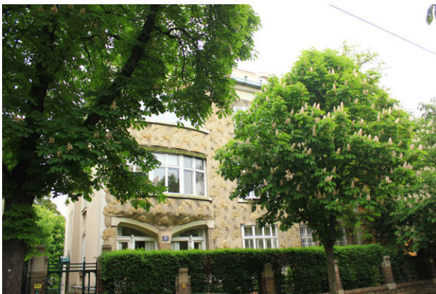
Figure A.314 Langerhaus in Vienna (1900): according to project done by Jože Plečnik (2014)
