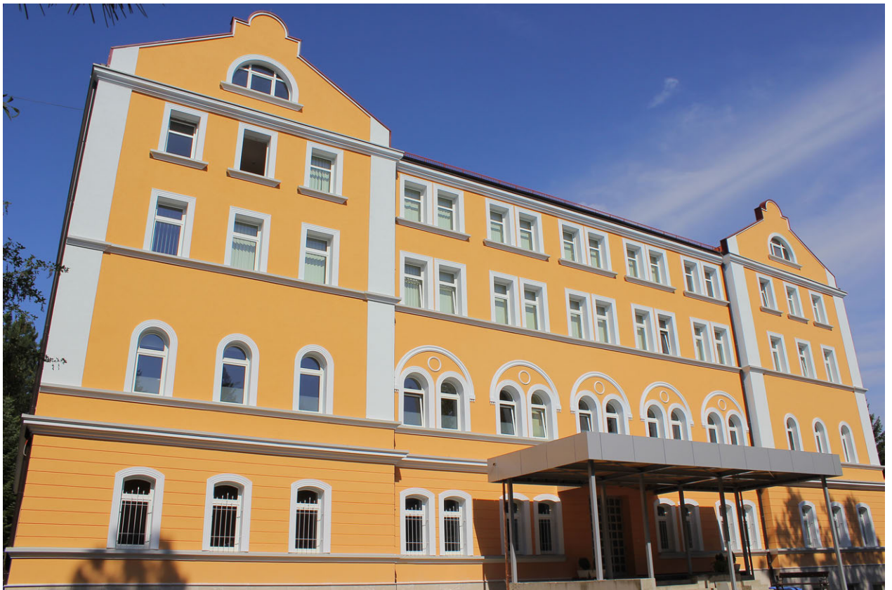
Figure A.288 The Convict of the Convent of Saint Bonaventure, Visoko: view of the main facade from the west (2013)
