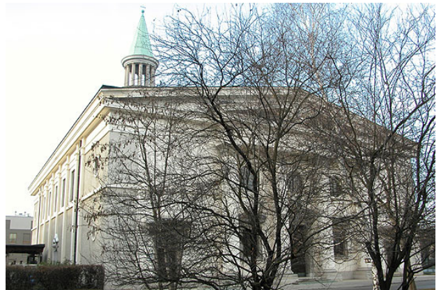
Figure A.325 Church of St. Francis of Assisi in Šiška, Ljubljana, (1925–1927): close-up view of the entrance façade; present condition ("Jože Plečnik - Cerkev Sv. Frančiška v Šiški")
