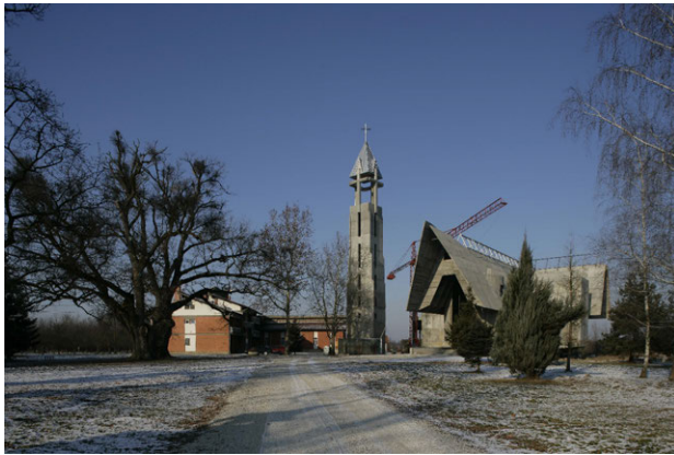
Figure A.50 The Parish Church of Sinless conception of the Blessed Virgin Mary, Dubrave: view from the south; photograph taken during the construction works on the church in 2006. Photo credit: Goran Vranić, Zagreb (Archive collection Dubrave)
