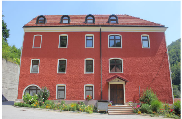
Figure A.154 The Convent of Saint Catherine: view of the western façade (2013)
