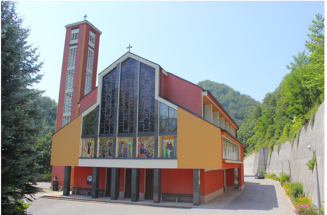
Figure A.172 The Parish Church of Assumption of Mary, Kreševo: view of the main façade from the north-east (2013)
