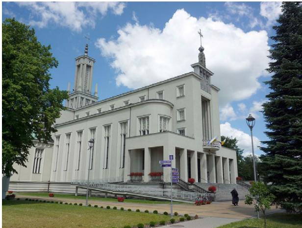
Figure 70 The Franciscan convent and the church of Blessed Virgin Mary the Immaculate (Shrine of St Maximilian Kolbe) in Niepokalanów, Teresin near Warsaw (Poland): view of the church erected 1948-1954 by Zygmunt Gawlik; site founded in 1927 ("Niepokalanów")
