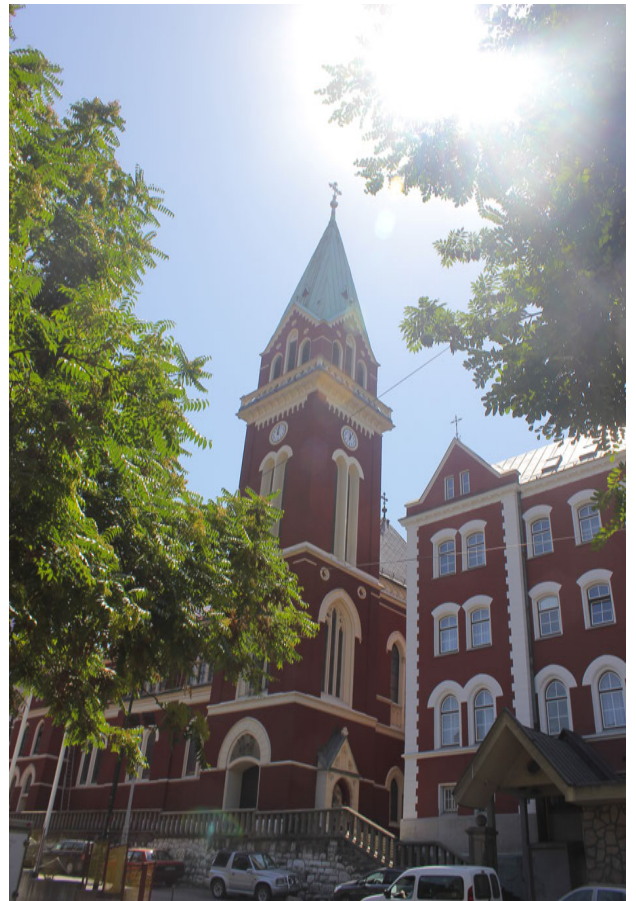
Figure A.14 The Convent and the convent church of Saint Anthony of Padua, Bistrić: view of the entrance staircase from the north-east (2013)
