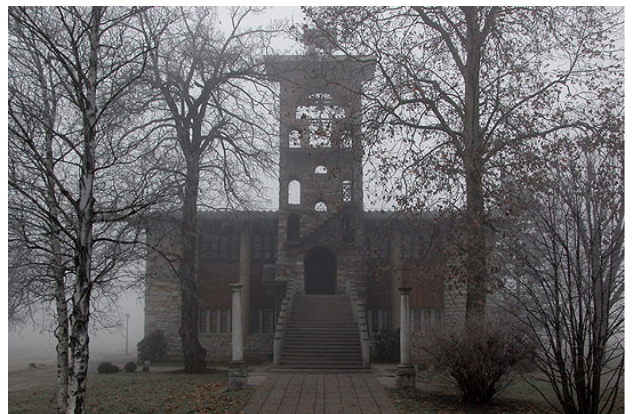
Figure A.326 Church of the Archangel Michael on the Marsh in Črna vas near Ljubljana, (1925–1939): view of the entrance façade; present condition ("Jože Plečnik - Cerkev Sv. Mihaela na Barju")
