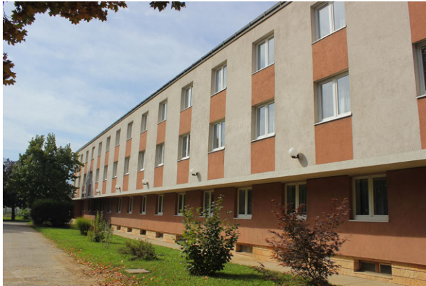
Figure A.7 The Convent of Saint Paul, Nedžarići: view of the north-eastern façade (2013)
