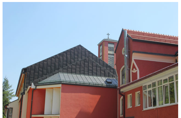
Figure A.174 The Convent and The Parish Church of Assumption of Mary, Krševo: close-up view of the back side of the church and the link to the convent, with the bell-tower in the background (2013)
