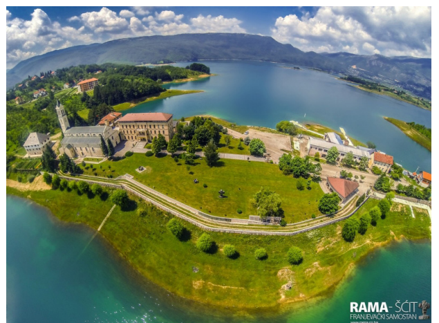
Figure A.216 The Convent and the Parish Church of Assumption of Mary, Rama-Šćit: aerial view of the site from the east (Fotogalerija Rama-Šćit)
