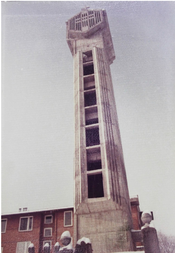
Figure 196 The Convent of the Holy Trinity: close up view of the campanile, view from the east; photograph taken after 1984 (Gradnja tornja 1984)
