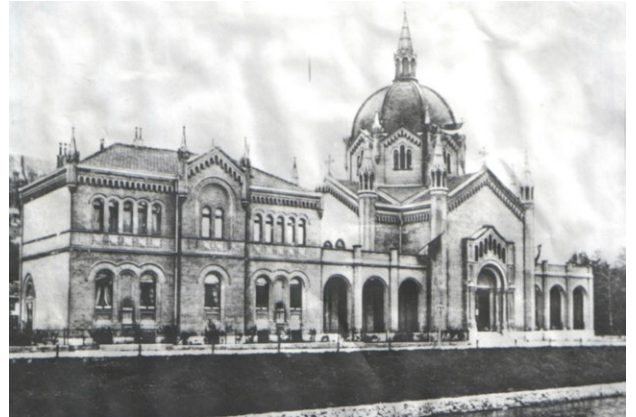
Figure A.307 Evangelistic church and parish house: view from the opposite side of the Miljacka River, built 1899-1911, according to project by Karel Pařík; photograph taken in the first years after the construction (Dimitrijević 26.e)
