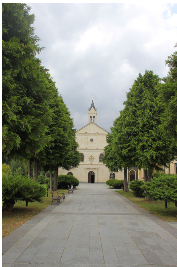
Figure A.206 The Parish Church of Assumption of Mary, Rama-Šćit: view of the access alley from the north (2013)
