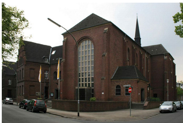
Figure 60 The Franciscan church of Saint Barbara and the convent of Fourteen Holy Helpers, Mönchengladbach (Germany): view of the complex built in 1889 ("Franziskanerkirche St. Barbara mit Kloster (Mönchengladbach)")
