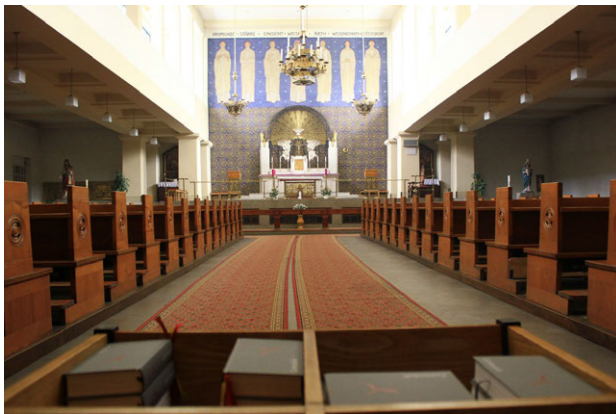
Figure A.316 Heilig-Geist-Kirche in Ottakring, Vienna: view of the main nave; present condition (2014)
