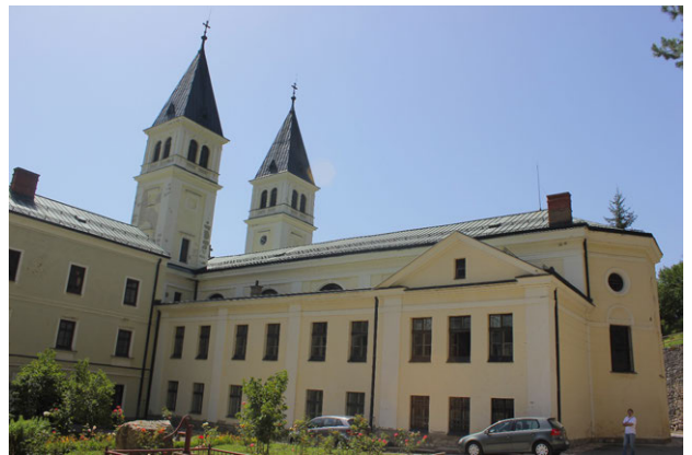
Figure 141 The Convent and the Parish Church of Saint John the Baptist, Kraljeva Sutjeska: view of the south-eastern wing of the Convent and the Church (2013)
