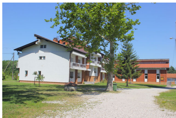
Figure A.39 The Convent of Saint Anthony, Dubrave: view of the convent buildings from the south (2013)
