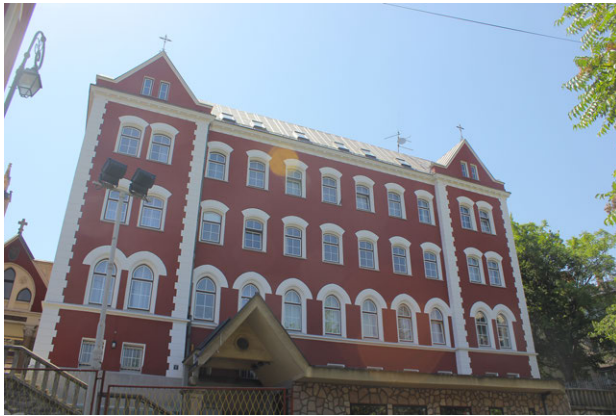
Figure A.15 The Convent of Saint Anthony of Padua, Bistrik: view of the northern façade (2013)
