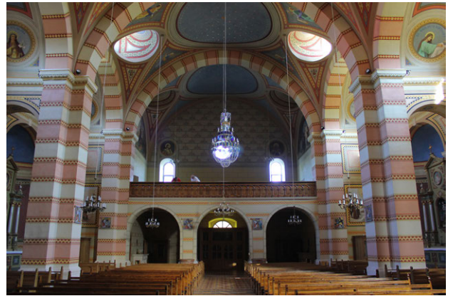
Figure A.89 The Church of Saint Peter and Paul, Gorica: Interior view of the main nave with the choir platform in the background (2013)
