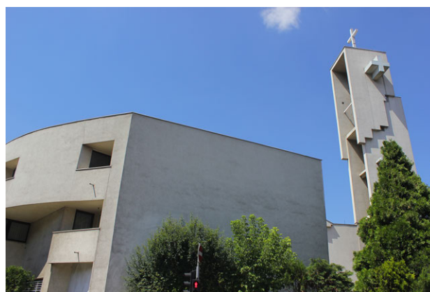
Figure 222 The Convent and the Parish Church of Saint Peter and Paul, Tuzla: view of the complex from the south (2013)
