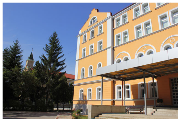
Figure A.289 The Convict of the Convent of Saint Bonaventure, Visoko: view from the southeast of the main facade in the foreground, with the Gymnasium building in the background (2013)
