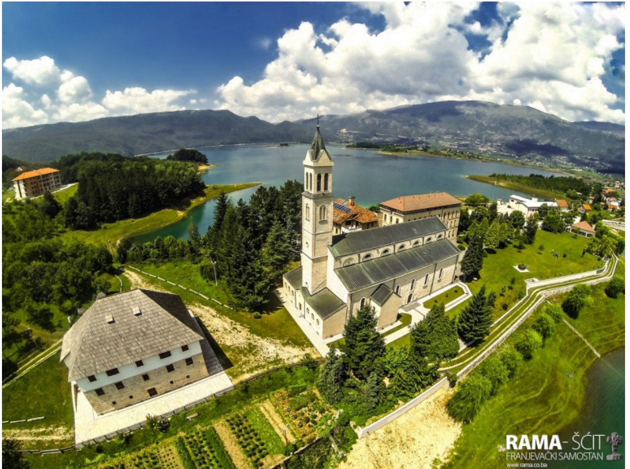
Figure A.217 The Convent and the Parish Church of Assumption of Mary, Rama-Šćit: aerial view of the site from the south-east (Fotogalerija Rama-Šćit)
