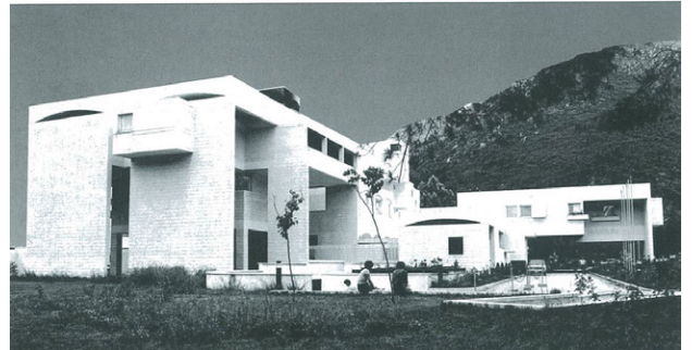
Figure A.339 Hotel "Ruža," Mostar; model and street view; done according to project by Zlatko Ugljen (1972-1975) (Ugljen, Bernik et. al, 96)
