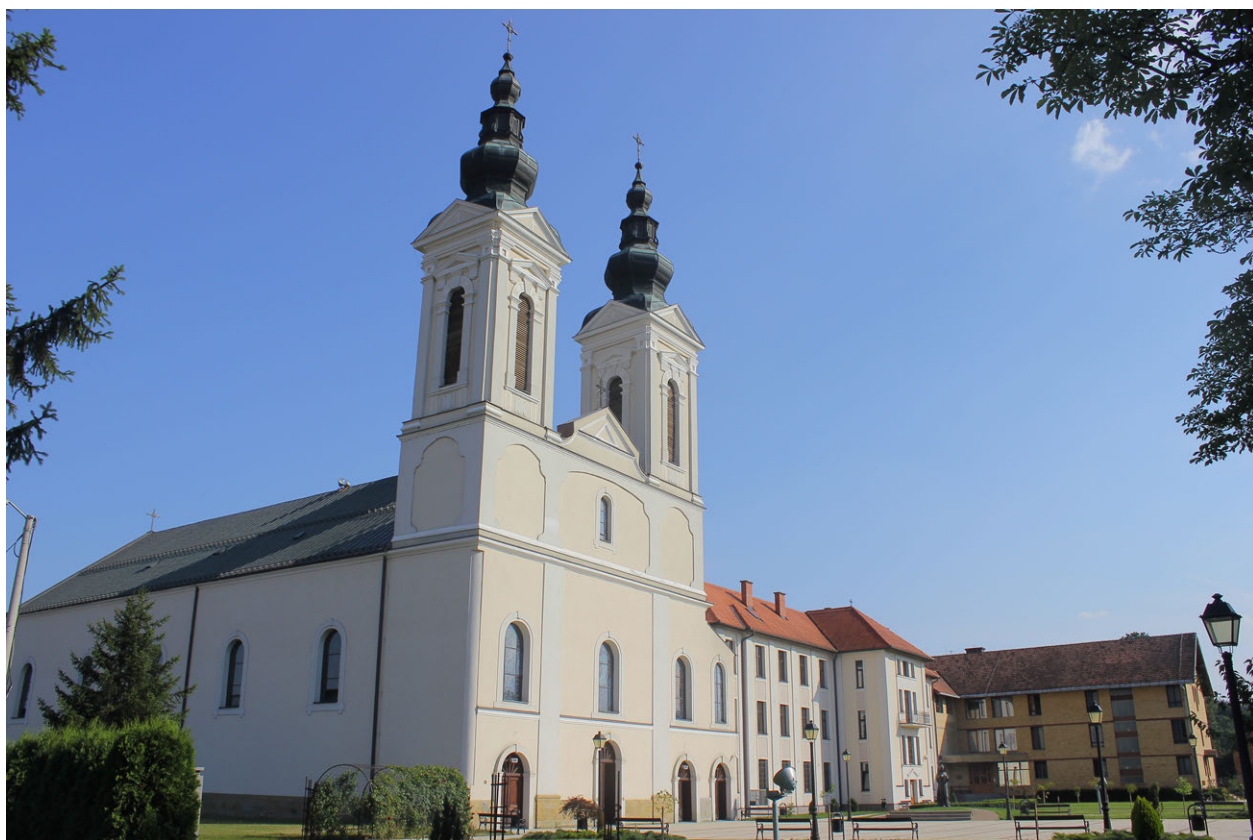
Figure A.261 The Convent and The Parish Church of the Assumption of Mary, Tolisa: complex, view from the north (2013)
