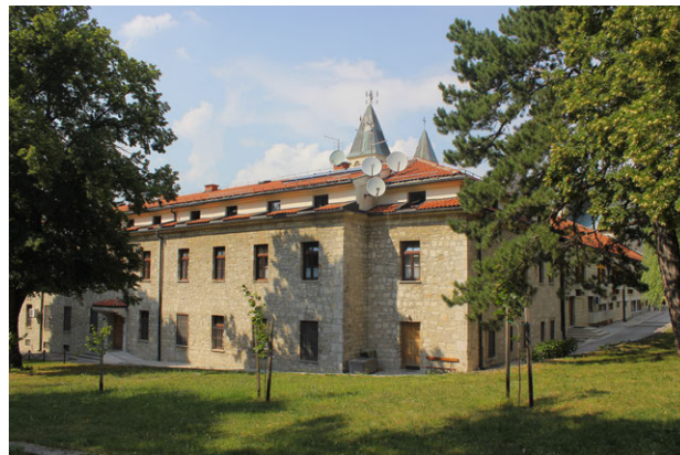
Figure A.75 The Convent of Saint Peter and Paul, Gorica: Close up view of the eastern corner (2013)
