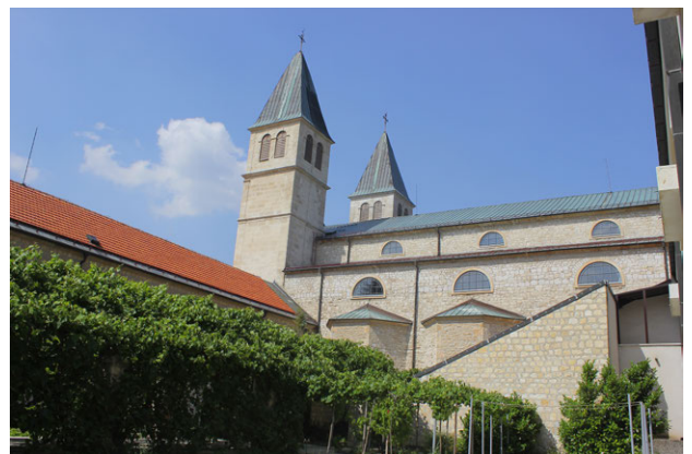
Figure A.87 The Convent and the Church of Saint Peter and Paul, Gorica: Close up view of the northern corner of inner courtyard (2013)
