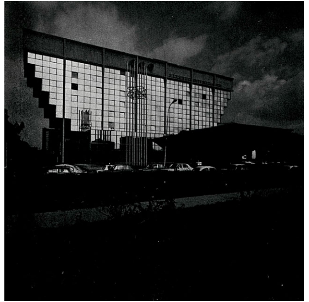
Figure A.330 BH Electric Power company headquarters, Sarajevo; done according to project by Ivan Štraus in 1978 (Štraus, Kurto et al. 1986)
