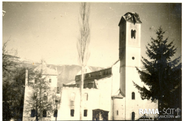
Figure A.204 The Convent and the Parish Church of Assumption of Mary, Rama-Šćit: view of the site from the south-west after the demolition in WWII (Fotogalerija Rama-Šćit)
