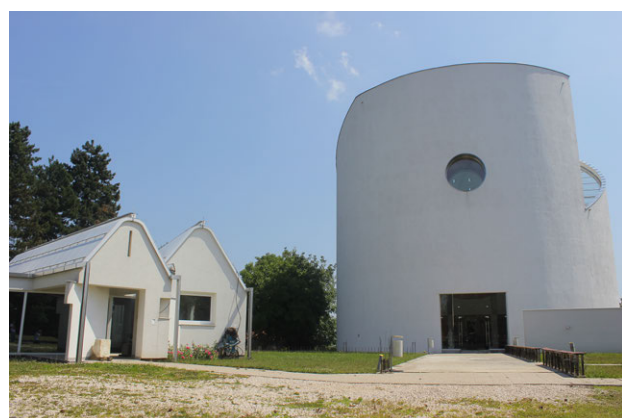
Figure 242 Plehan Religious and Cultural Centre: view of the sacristy and administrative buildings on the left and the Parish Church on the right (2013)
