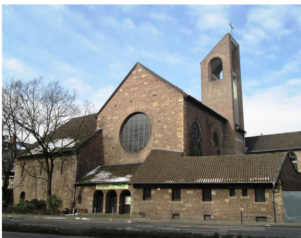
Figure 72 Former Franciscan convent and the church of Saint Mary, Köln: view of the complex done by Karl Schellen in 1893-1900, and remodeled by Emil Steffann in 1952-1958 ("Franziskanerkloster Köln")
