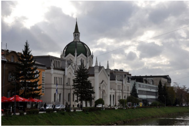
Figure A.306 Evangelistic church and parish house: view from the opposite side of the Miljacka River, built 1899-1911, according to project by Karel Pařík; present condition of the complex, currently the seat of Academy of Arts in Sarajevo ("Akademija likovnih umjetnosti u Sarajevu")
