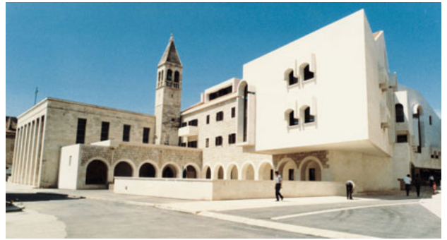
Figure 92 The Convent and the Parish Church of Our Lady of Health, Split: church done 1936-1937 by Lavoslav Horvat and convent done 1984-1986 by Slaven Rožić ("Split - samostan i župa Gospe od Zdravlja")
