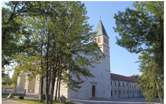
Figure A.80 The Convent and the Church of Saint Peter and Paul, Gorica: View of the complex from the north (2013)
