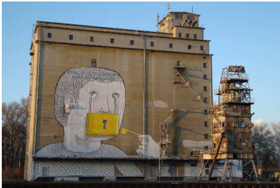
Abb.39. Silospeicher in Albern
