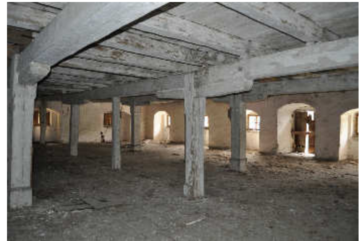
Abb.124. Blick Wand b/c
