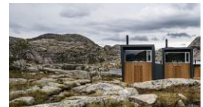
Abb.0 77 Zugang zu Mountain Cabins
