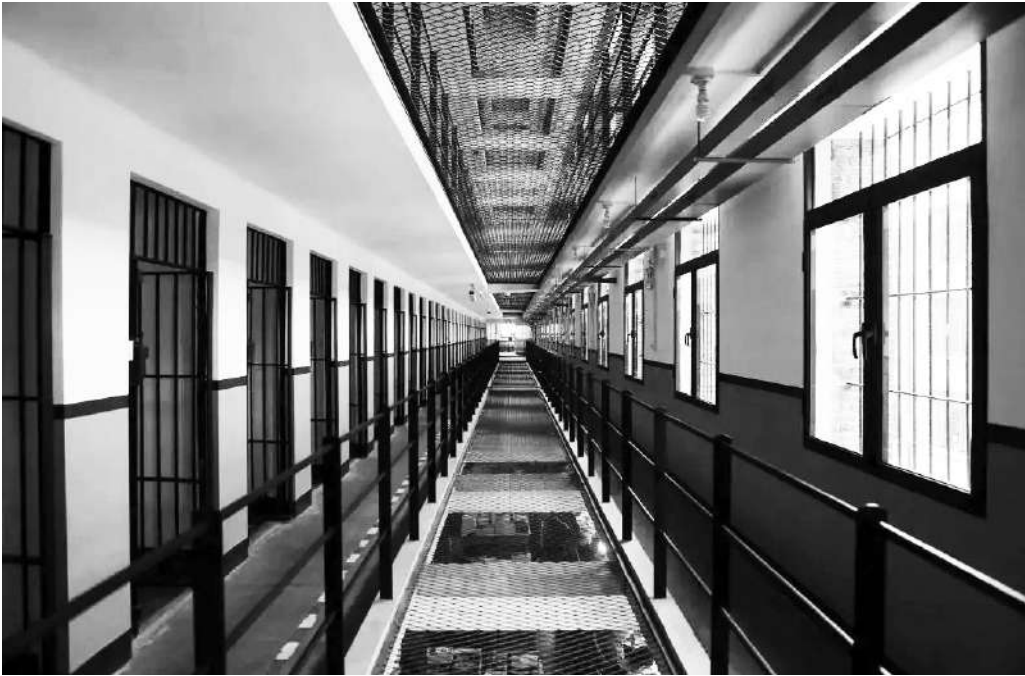
Fig.24 Cells Block from the inside
