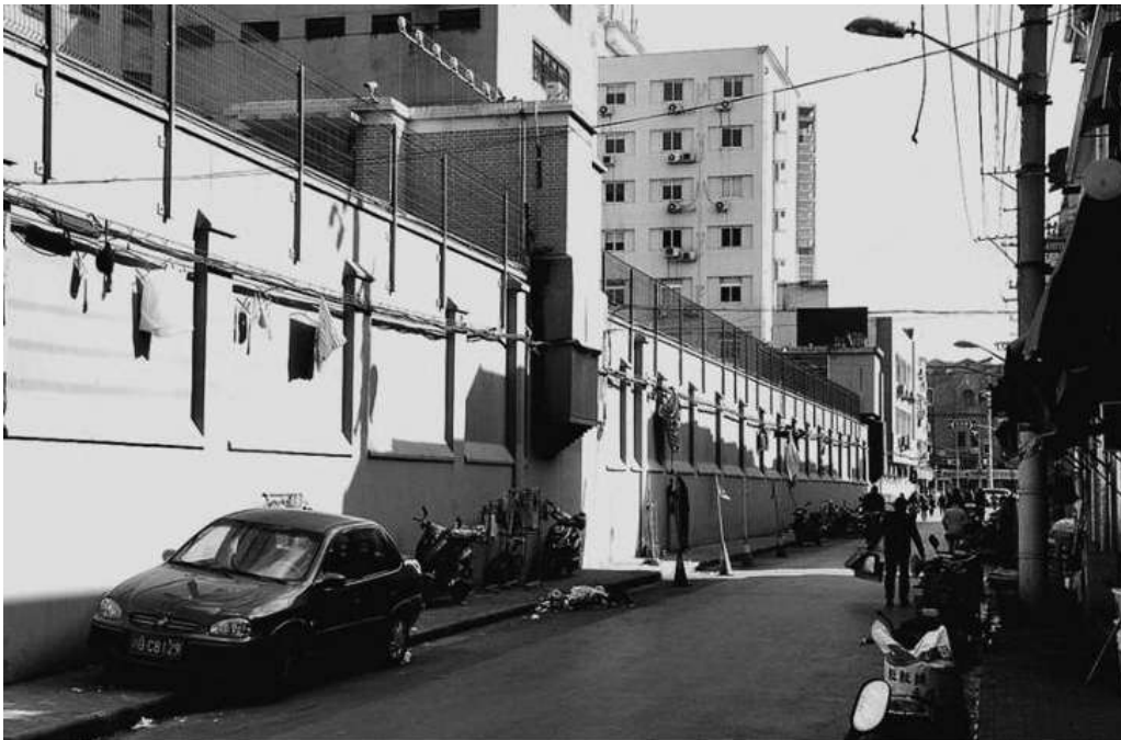
Fig.29 Ward Road Gaol surrounding wall
