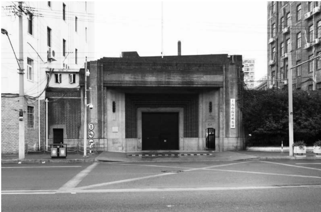
Fig.28 Ward Road Gaol main gate
