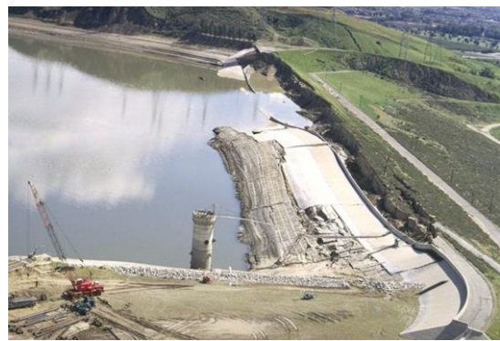
Figure 7 “Near” failure of Lower San Fernando Dam (Wieland 2013)
