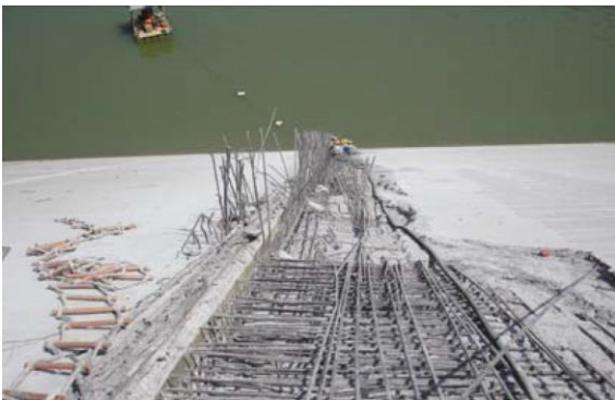
Figure 93 Repair works at vertical slab joints (Guan 2009)
