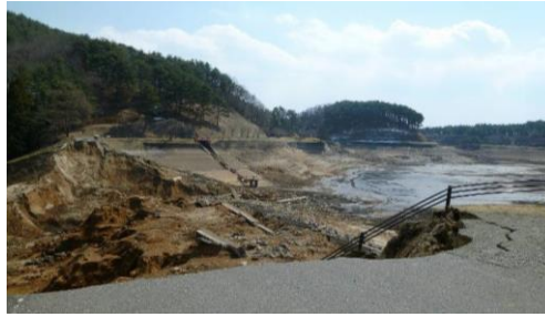
Figure 9 Failure of Fujinuma-ike dam after the Tohoku earthquake (Matsumoto 2011)
