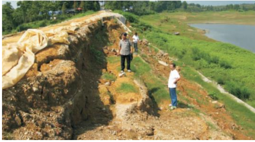
Figure 8 Upstream slip surface Wenchuan earthquake 2008 (Wieland 2013)
