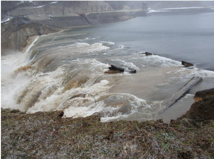
Figure 110 Overtopped crest of Fujinuma dam (EERI, 2011)
