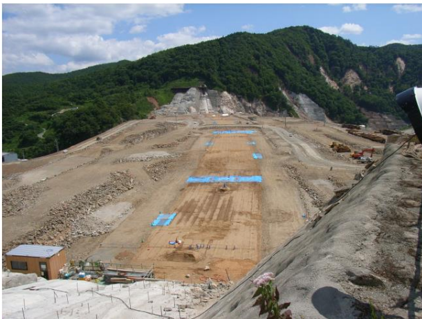
Figure 42 Isawa dam during construction after Iwate /Miyagi earthquake in 2008 (Ohmachi 2008)
