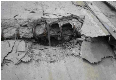
Figure 4 Horizontal construction joint of Zipingpu CFRD (Chen and Sheng-Shui n.d.)
