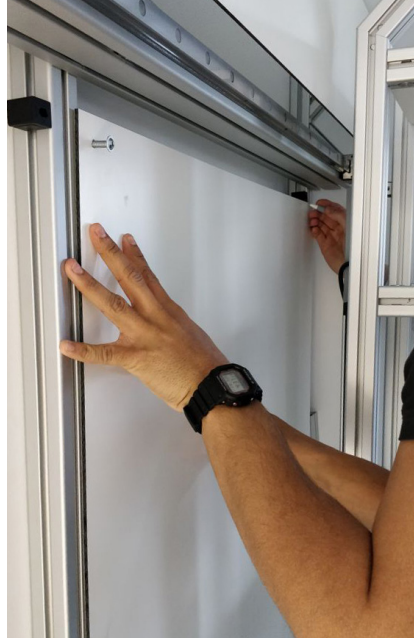
5.25 Scenario - Maintenance: removing and mounting of wall panel, movable racks allow to open up space for the task.
