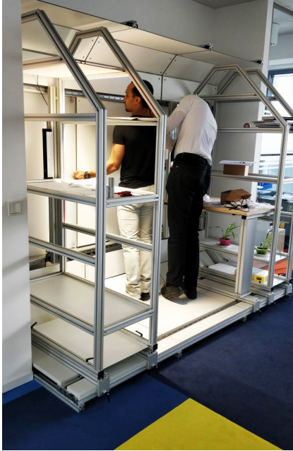
5.25 Scenario - Maintenance: removing and mounting of wall panel, movable racks allow to open up space for the task.
