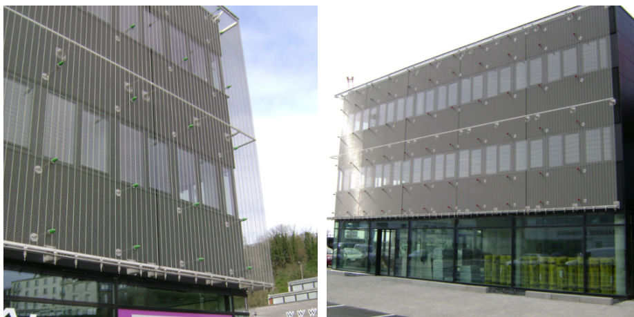
Figure 6. Office building, Brest – Northwest France
