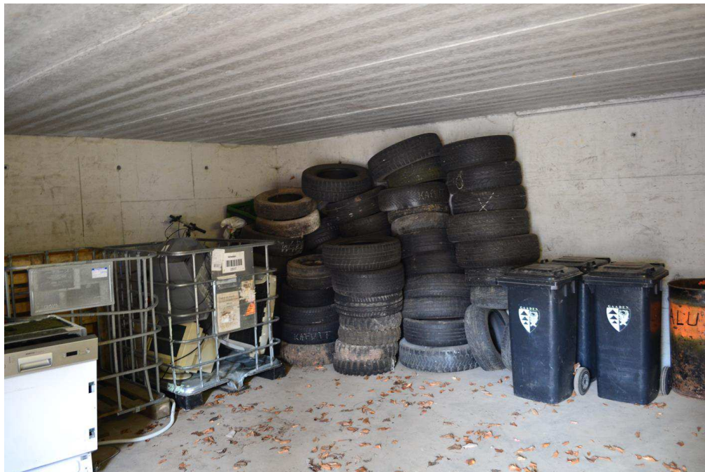
Figure 11. – Unspecific storage area for old tires.
