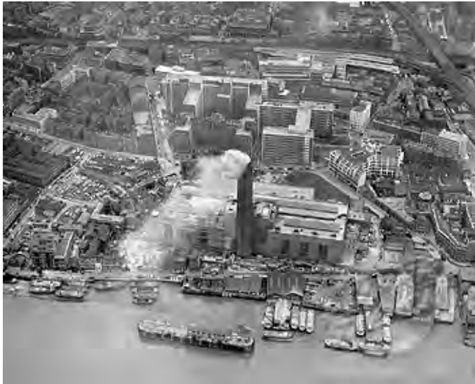
The oil-fired Bankside Power Station operating in 1963 in Southwark, London, designed by Sir Giles Gilbert Scott.
