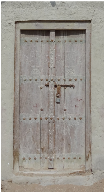
figure 4.20. door in Laaft (Doubrawa, 2015d)
