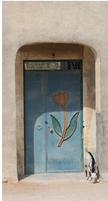
figure 4.18. door in Chahu Sharghi (Doubrawa, 2015b)
