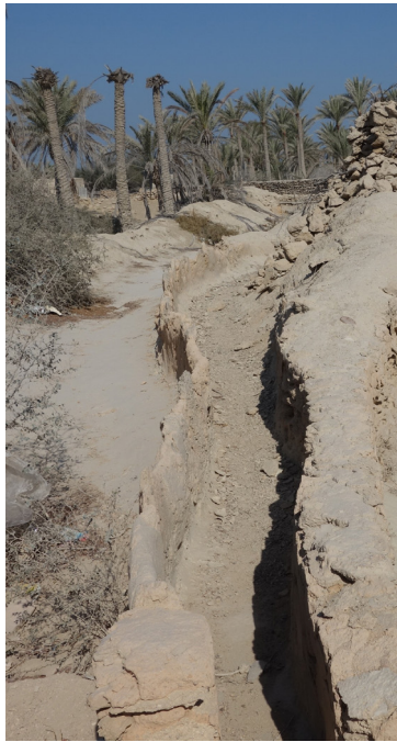
figure 4.40. channel made out of sarooj for watering palm trees (Rieger- Jandl, 2015p)
