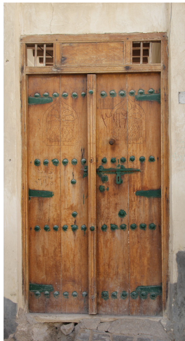
figure 4.21. door in Laaft (Doubrawa, 2015e)
