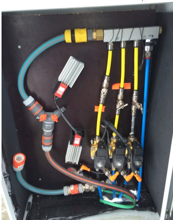
Figure 3.1: Water distribution system
