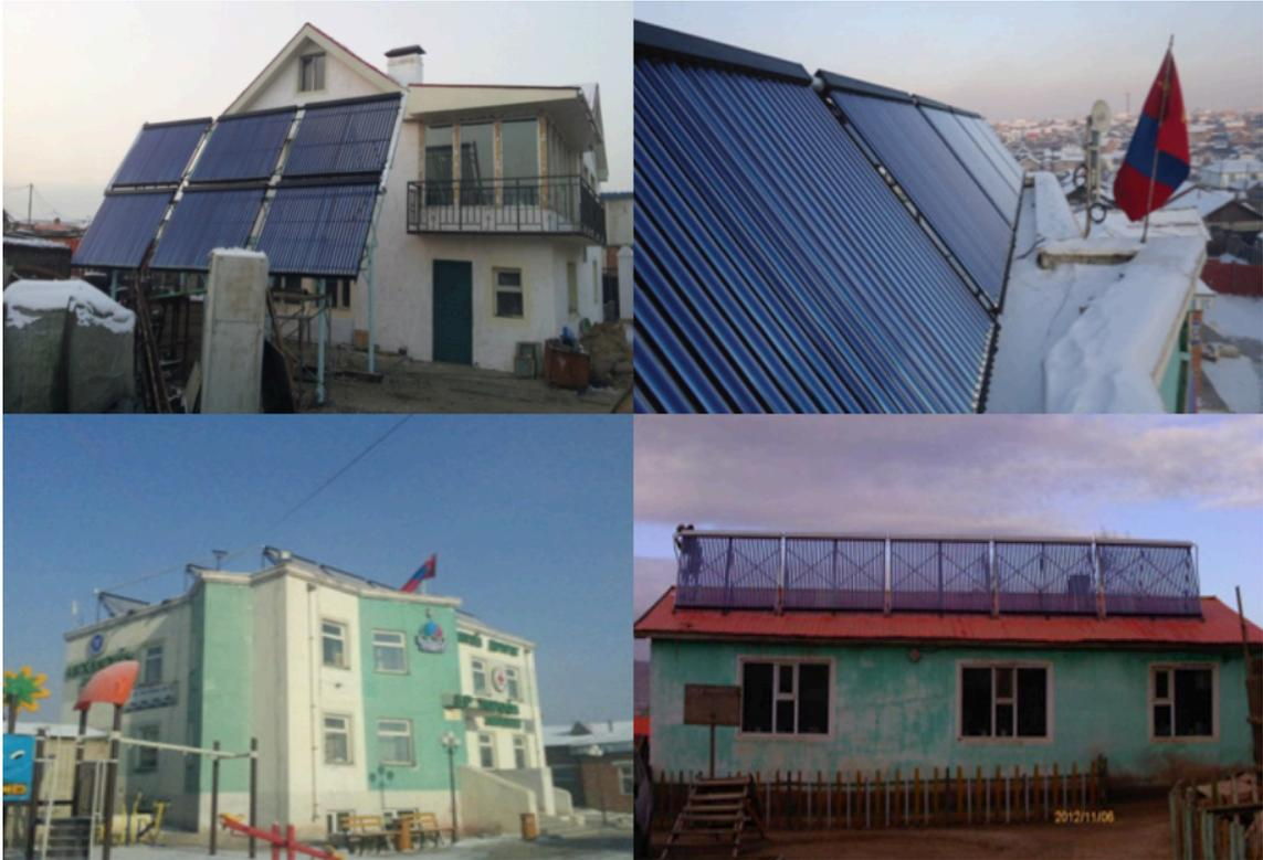
**Figure 17:** Solar air collectors with water-based delivery systems installed on buildings in Ulaanbaatar's ger districts. *Source:* City Air Quality Department 2013.
