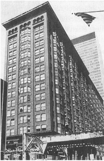
Abb.10. Monadnock Building in Chicago, Holabird & Roche 1893 ©Hascher/Jeska/Klauck
