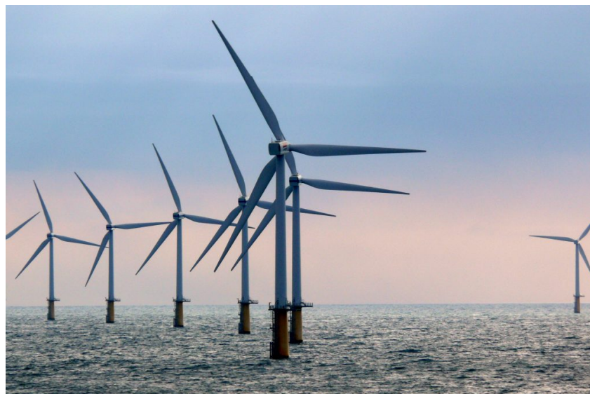
Figure 15: Offshore Wind Energy Harvesting. Princess Amalia Wind Farm in the North Sea. 62
