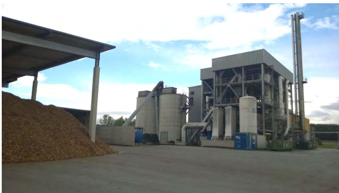
Figure 4.3: Picture of the DFB biomass steam gasification power plant Oberwart in 2014; from the left to the right: storage of wood chips, biomass feeding system, dryer, steel construction with gasification and gas cleaning, engine room, stack.
