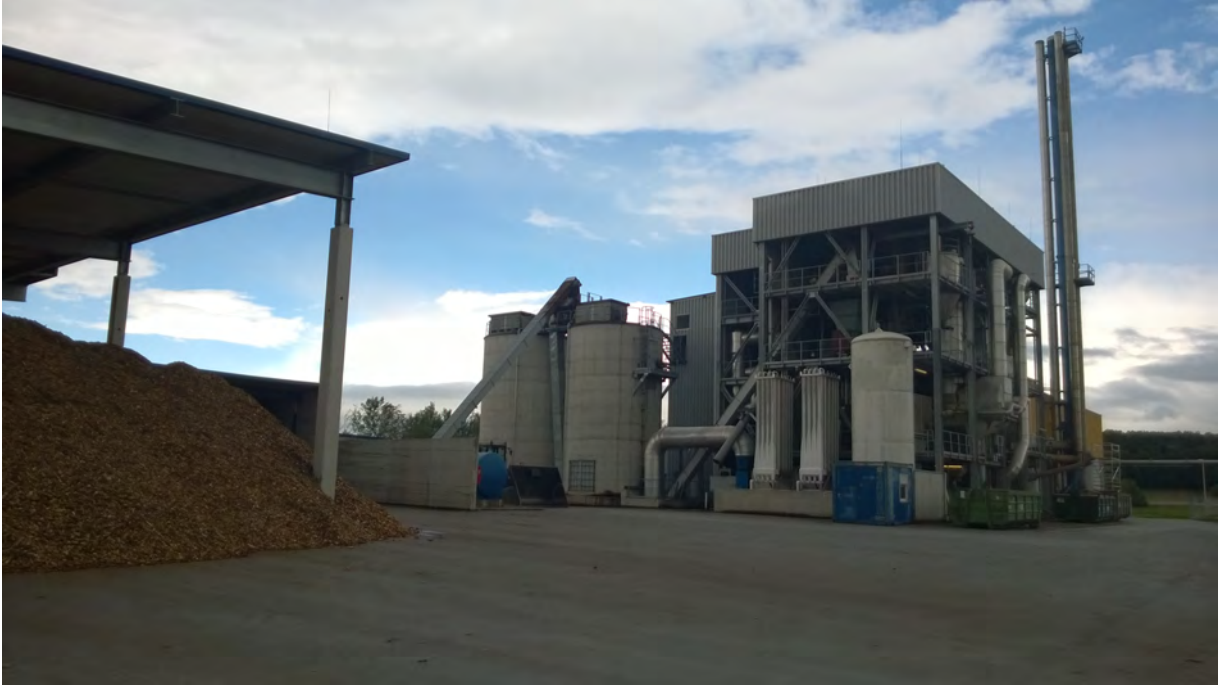
Figure 1: S1 – Picture of the CHP plant Oberwart, Austria.
