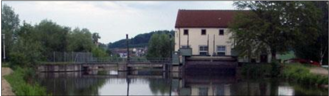
Figure 37: Ellzee, run-of-river plant 49
