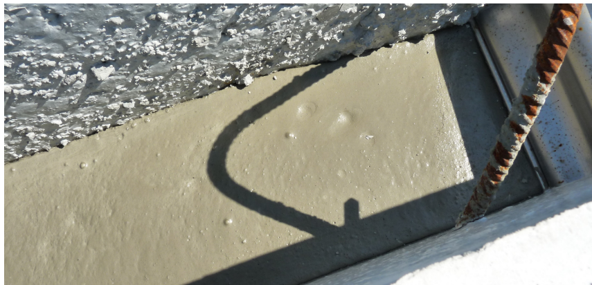
Figure 3.46: The upper surface of the self compacting concrete after the concreting process
