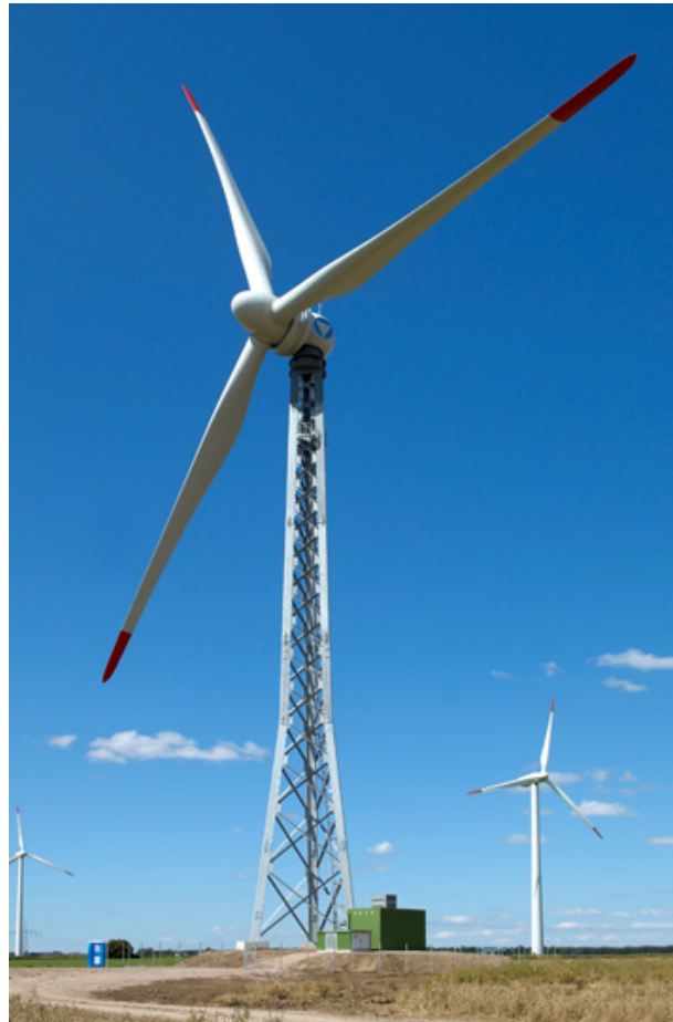
Figure 2.6: Lattice tower of voestalpine, taken from Voestalpine (2013)
