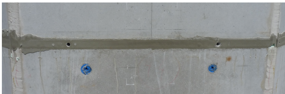
Figure 3.38: Concreted horizontal joint along the double wall element displaying that the EPDM equalizing layer fulfilled its task
