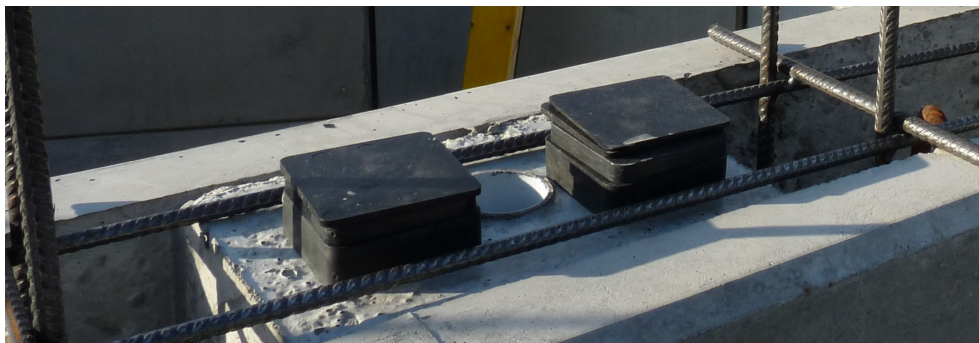
Figure 3.31: Plastic spacers on a concrete block providing the horizontal joint size of 30 mm and the needed horizontal plane
