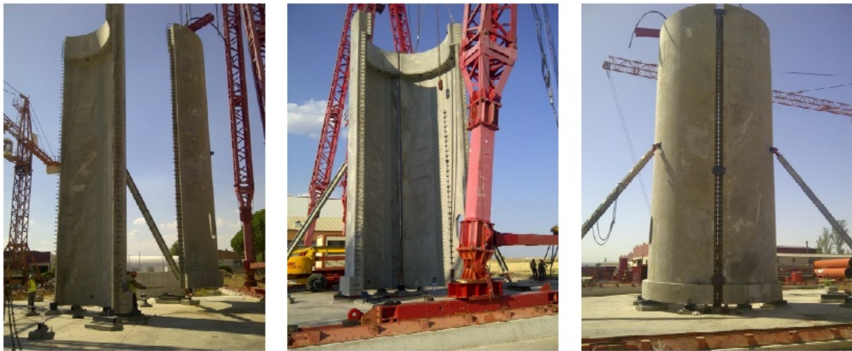
Figure 2.14: Assembling a prototype segment out of three precast elements showing the vertical joints of the telescopic tower, taken from Mendizabal (2014)
