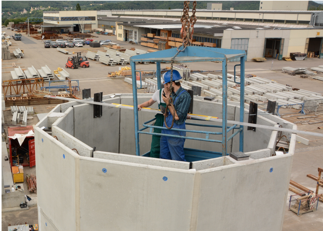
Figure 3.49: Placing distance plates to set up the horizontal plain, determined with a spirit level from a crane basket
