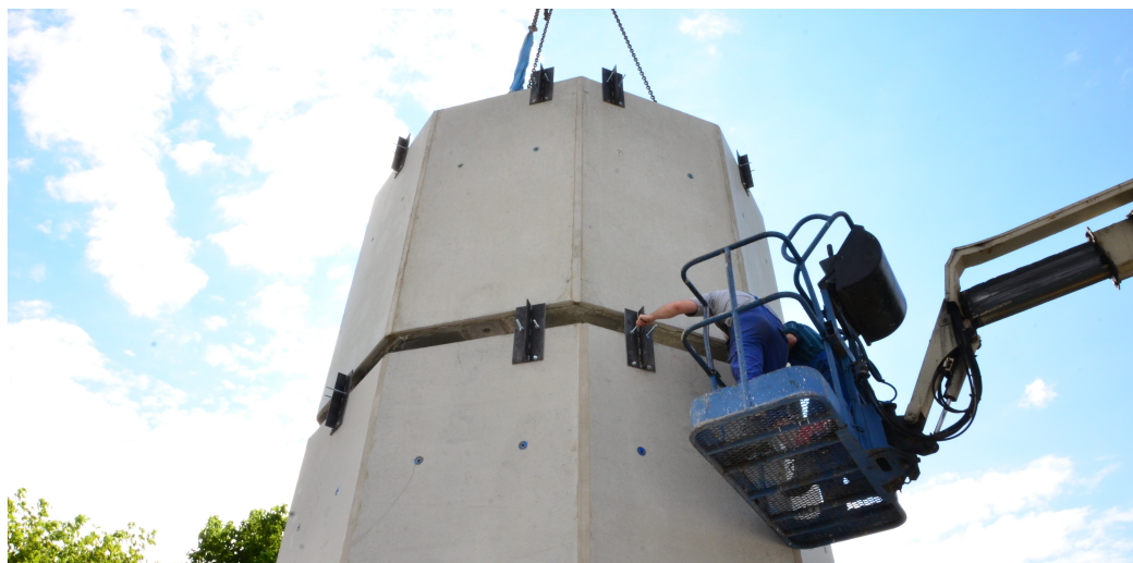
Figure 3.50: Placement of the segment 3 performed from a cherry picker
