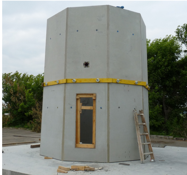
Figure 3.45: The two lowermost segments with the wooden formwork ready for concreting
