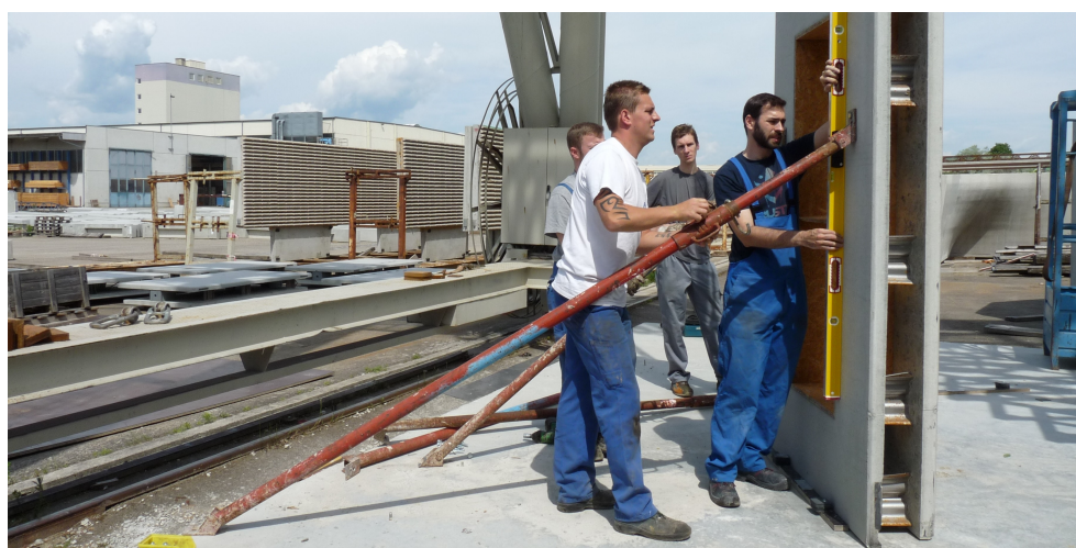
Figure 3.18: Final adjustment of the push-pull-props in order to establish the desired inclination of 1^\circ in relation to the vertical axis using a digital spirit-level to measure the inclination
