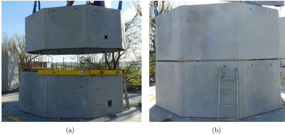
Figure 3.30: Placement of Segment 5 on Segment 4, (a) with the out-sticking reinforcement and the partially pre-assembled horizontal joint formwork, and (b) view of the horizontal joint without formwork
