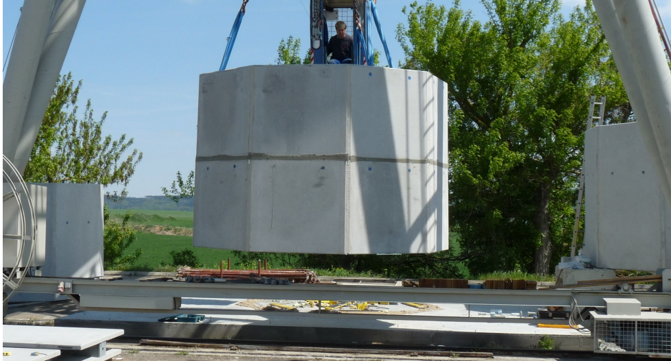
Figure 3.39: Lifting of the segments 4 and 5 after they had been concreted together
