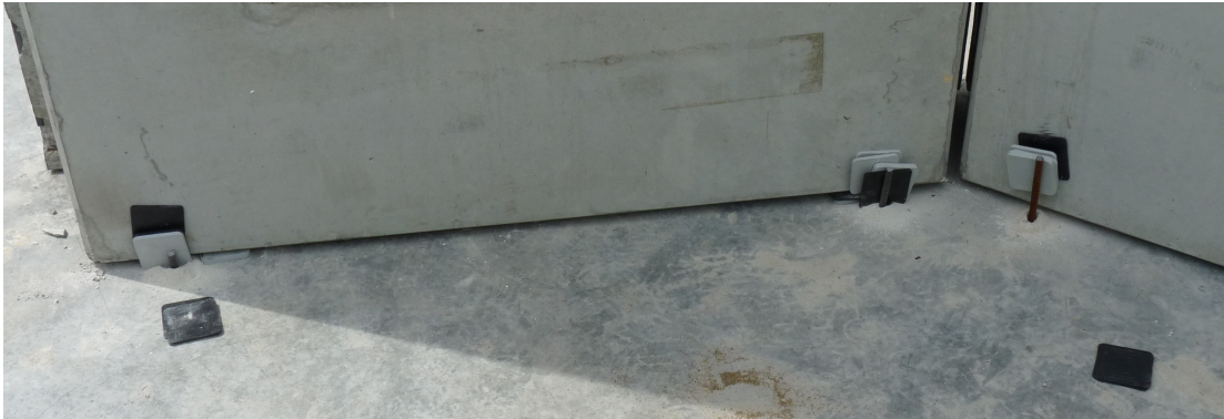
Figure 3.19: View from the inside of a segment showing steel bars with plastic plates used as wedges to clamp the double walls against the outer aligning board, therefore keeping the elements in the right position
