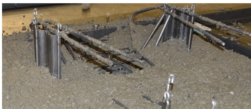
Figure 3.57: Additional concrete is poured onto the lifting hooks in order to provide a better anchoring, thus increasing the thickness of the slabs
