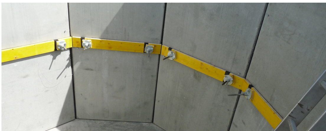
Figure 3.33: Horizontal joint formwork inside a segment
