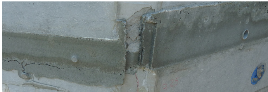
Figure 3.37: Imperfections of the concreted edge geometry
