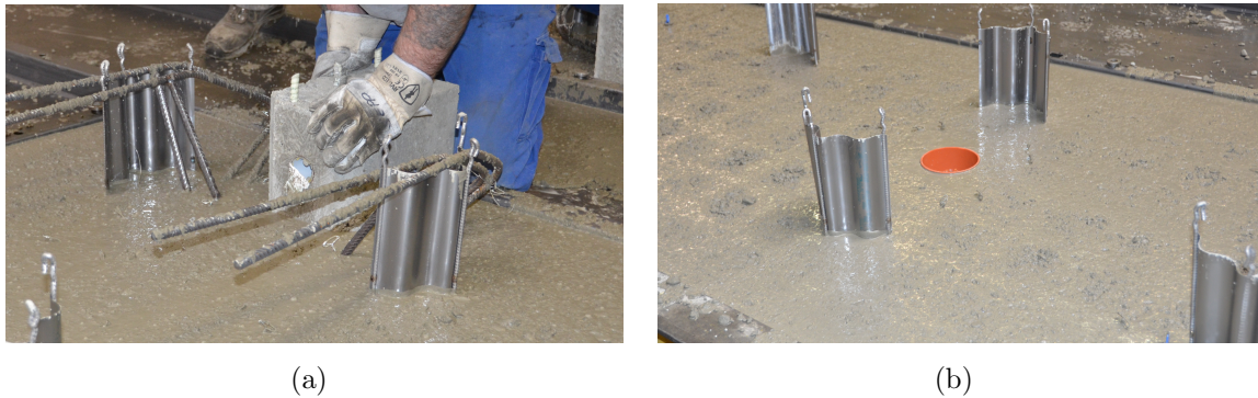
Figure 3.11: Double wall compacting by vibrating (a) whereby the concrete variant of the lifting and positioning embedment was held manually in position and (b) the result of the compacting process with a maybe too smooth surface of the inner side of the concrete slab
