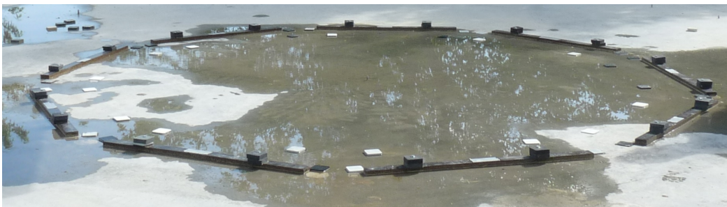
Figure 3.15: Prepared pre-assembly field with alignment boards and height adjusting plastic plates
