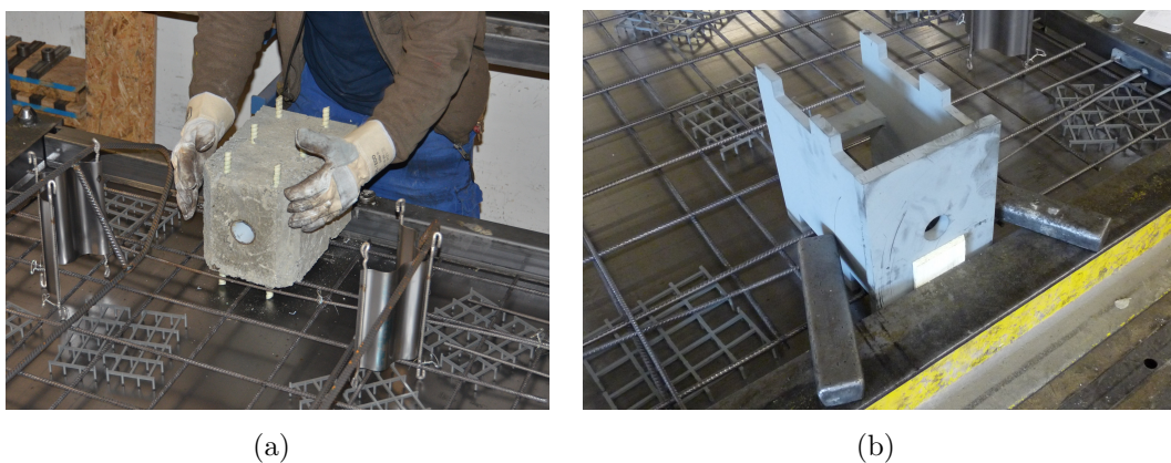
Figure 3.8: Lifting and positioning embedment in the shape of (a) concrete blocks fixed manually and (b) a " \pi " shaped steel part fixed by magnets
