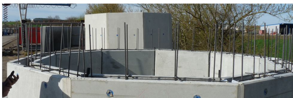
Figure 3.29: Vertical reinforcement cages placed into segment 4
