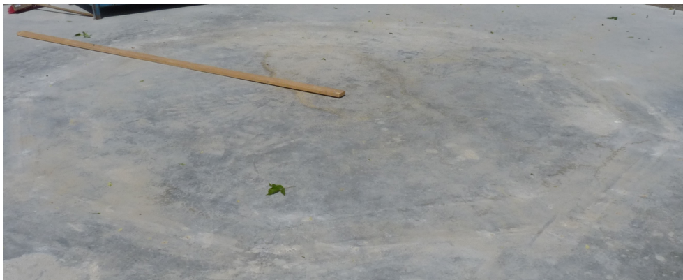
Figure 3.13: A wooden plank is used to draw the outer bottom circumference of the segments with the help of a reference point in the middle
