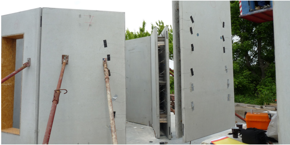
Figure 3.22: Positioning of the last double wall without horizontal reinforcement, showing the steel cable reinforcement in the neighbouring panels
