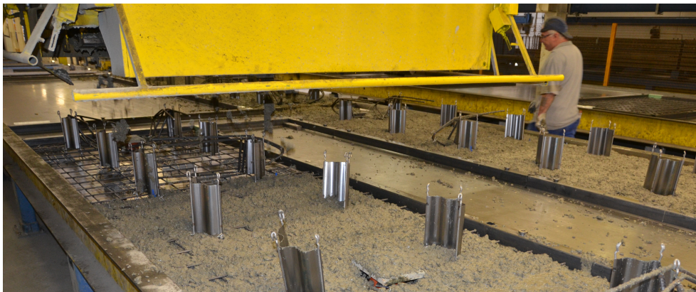
Figure 3.10: Crane bucket filling the formwork with concrete
