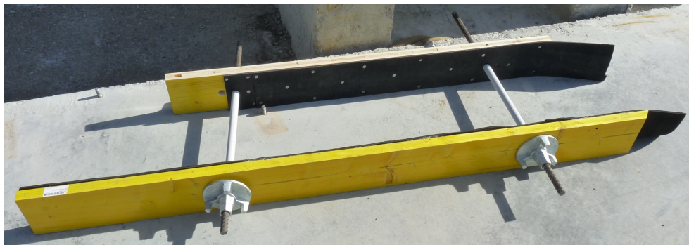
Figure 3.32: Formwork for horizontal joint of one double wall consisting of wooden boards with an onglued 5 mm thick EPDM layer connected by anchor bars and plates whereby the bars between the wooden boards are covered by plastic tubes
