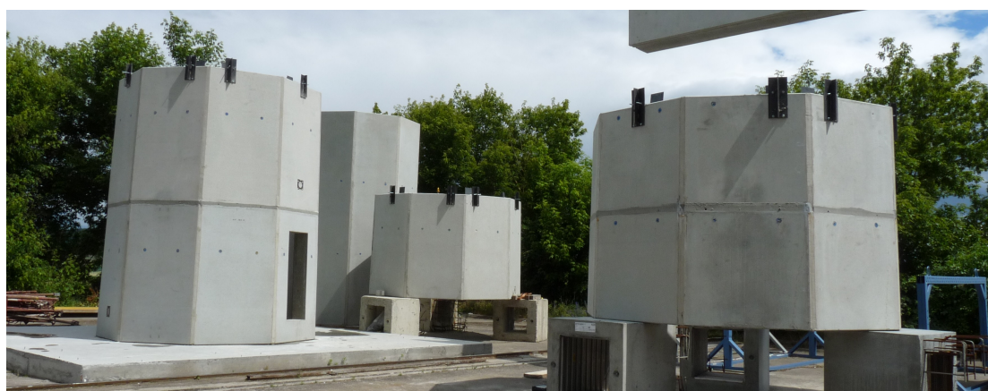
Figure 3.48: All segments on ground with the guiding parts easing segment placement
