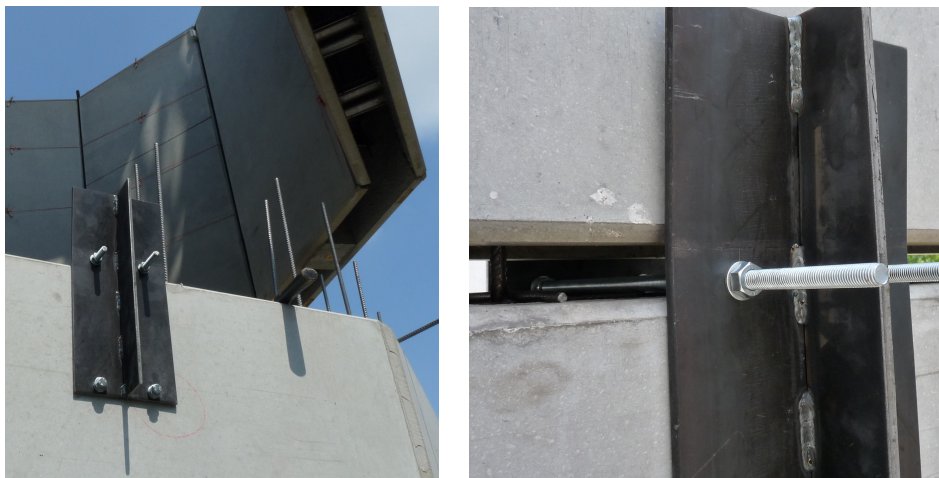
Figure 3.44: Guiding parts mounted to a segment during the positioning process
