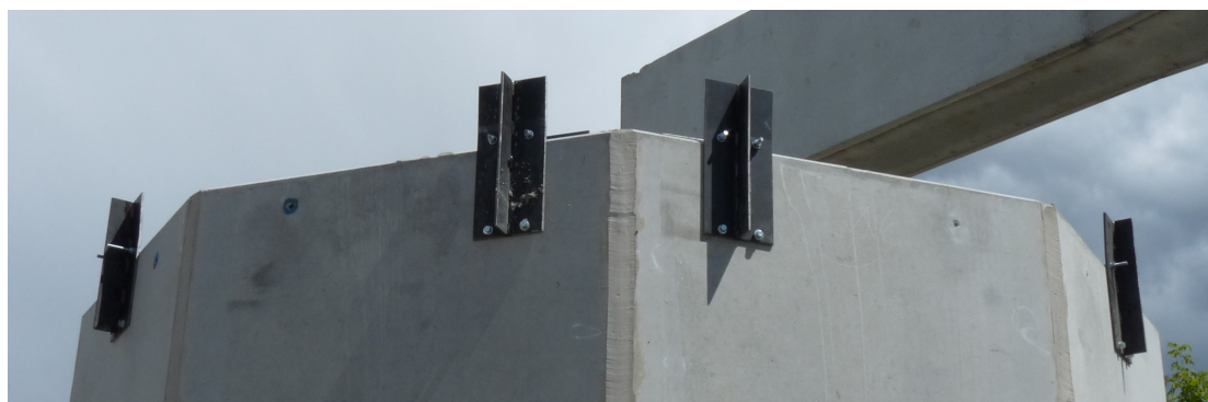
Figure 3.47: Distribution of the steel guidance parts at a horizontal joint
