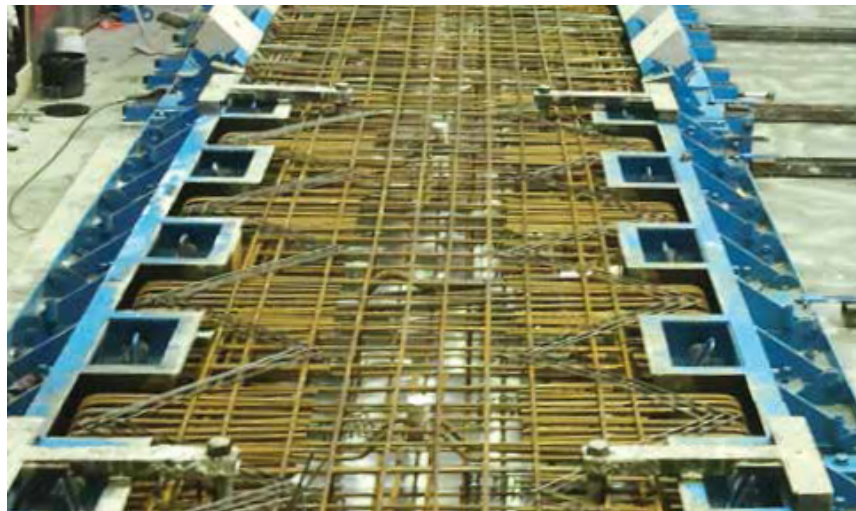
Figure 2.12: Steel formworks provide the expected accuracy of the elements, taken from Ventur (2013)
