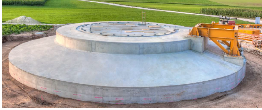
Figure 2.9: A foundation with the connection to the tower and the tower crane's steel foundation for a hybrid Max Bögl tower, taken from Max Bögl (2012)
