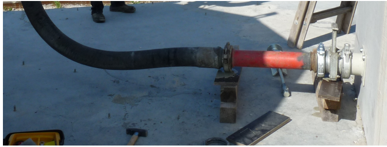
Figure 3.36: Concreting hose connected by a climp collar to an adapter tube (with a valve) bolted to a double wall
