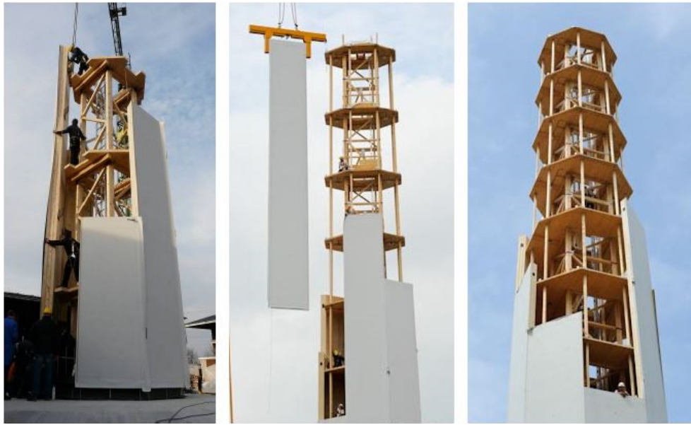
Figure 2.3: Assembling the sheathing panels in a spiral orientation, taken from TIMBERTOWER (2014)
