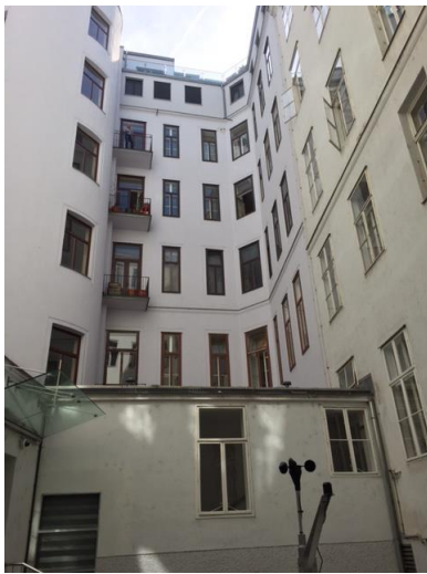
Figure 17: Courtyard at P1
