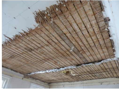
d.) Removing the last parts of the reed mats layer
