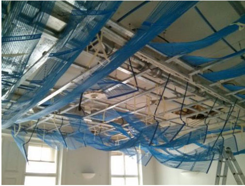
c.) After removal of gypsum cardboards
