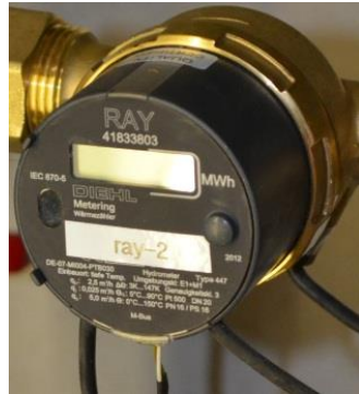
Figure 14. EWT Ray heat meter.
