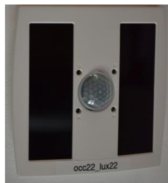
Figure 12. Thermokon SR-MDS Solar. Figure 13. Thermokon SR-MDS Solar in seminar room west.
