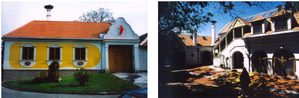
Figure 4 and 5. NAT after the renovation in 1996 (Source: NAT administration).
