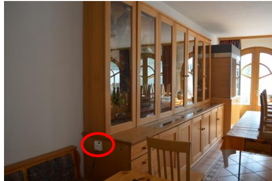
Figure 10. Thermokon SR04 CO2. Figure 11. Thermokon SR04 CO2 in seminar room east at NAT.
