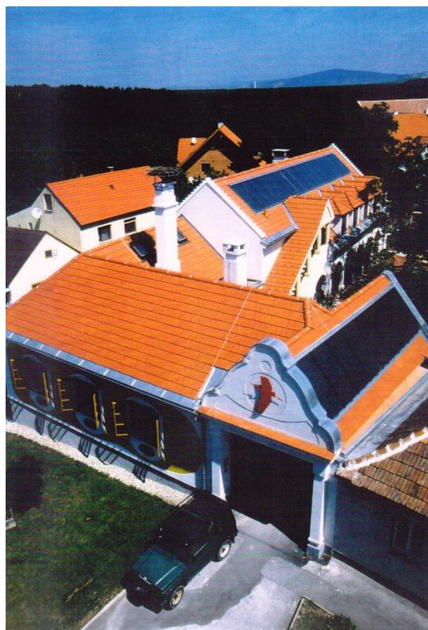
Figure 9. Aerial view on NAT after the renovation (Source: NAT administration).
