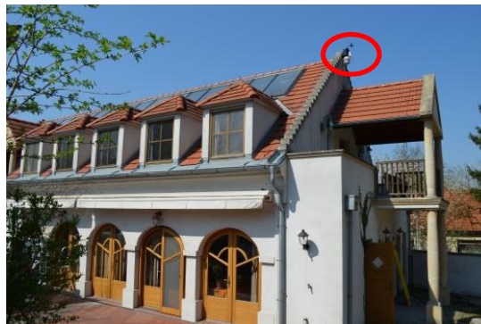
Figure 25. Weather station installed on NAT'S roof.
