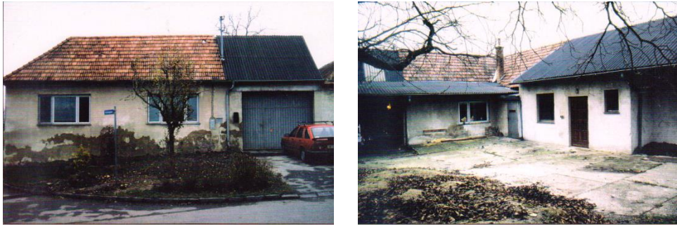
Figure 2 and 3. NAT before the renovation in 1994 (Source: NAT administration).
