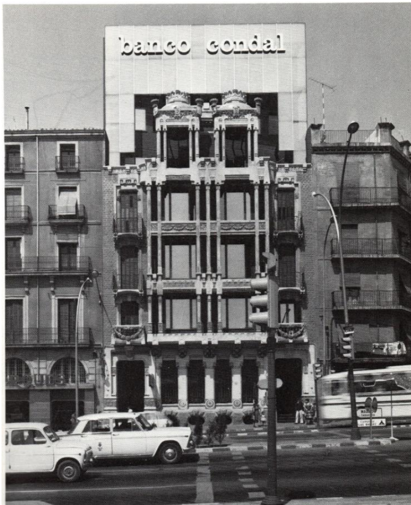
Abb. 147: Banco Condal in Lerida, Luis Domenech-Girbau, 1974
