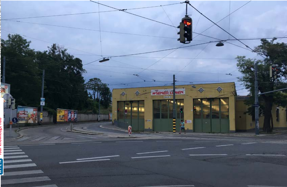
Figure 65 The tram garage north of the site.
