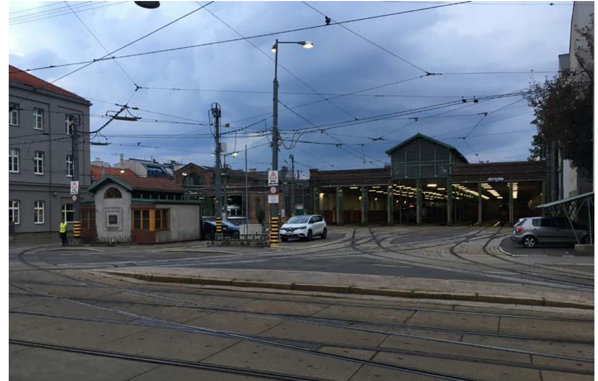
Figure 66 The tram garage south of the site.
