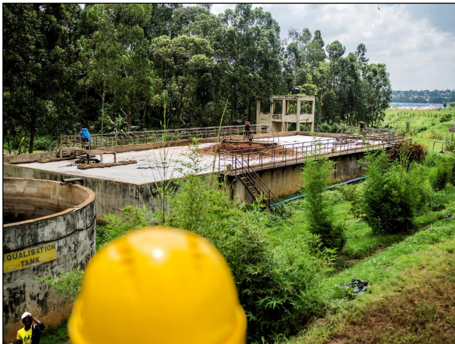
Figure 1.3: Inactive leachate aeration tank at the Kampala dumpsite SOURCE: The Uganda Waste Report, ©Timothy Bouldry, 2018
