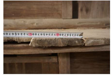
Fig.4.118 The floors of granaries are composed of 3 cm thick wooden planks with tongue and groove joints
