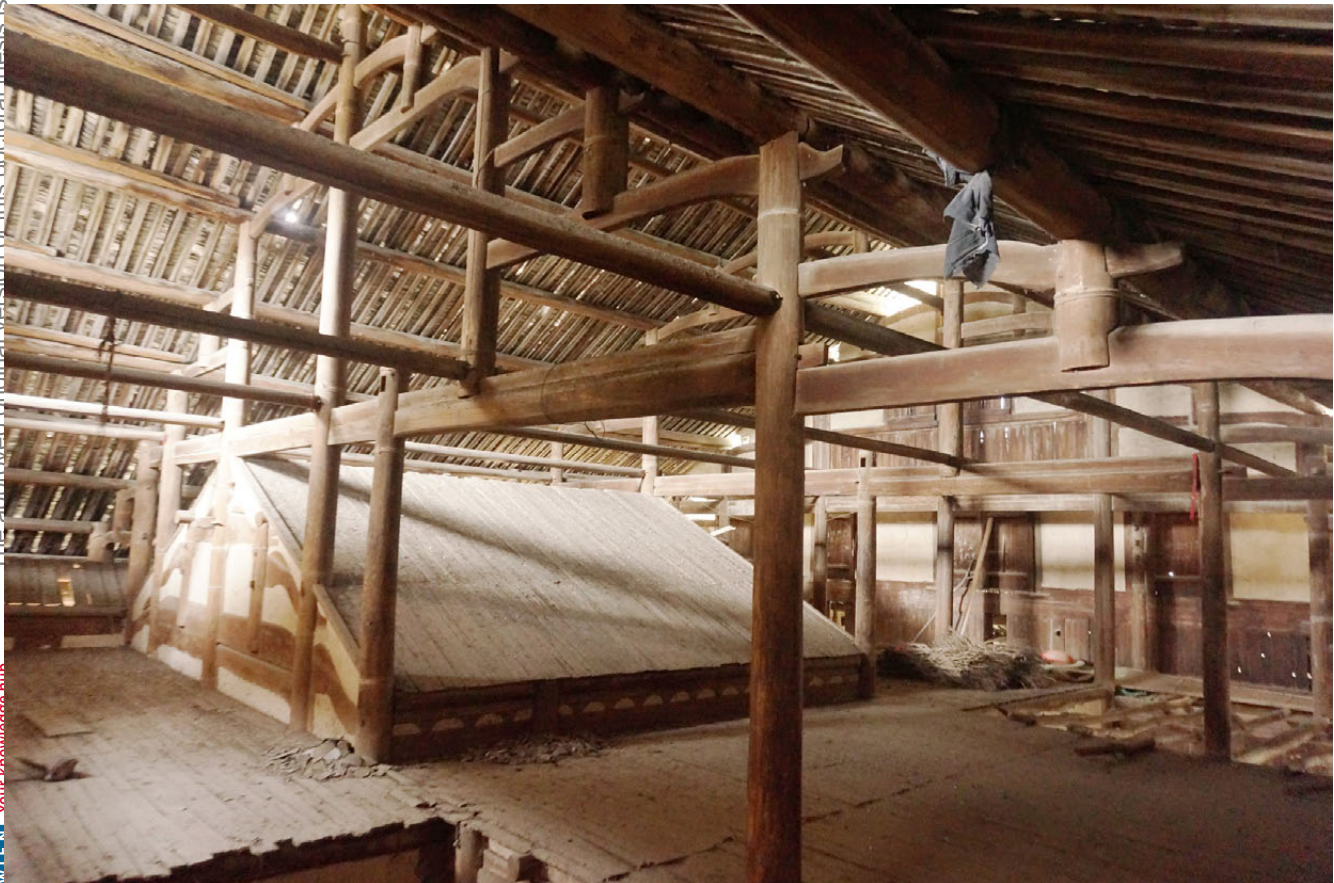
Fig 3.44 The attic area of the dwelling.
