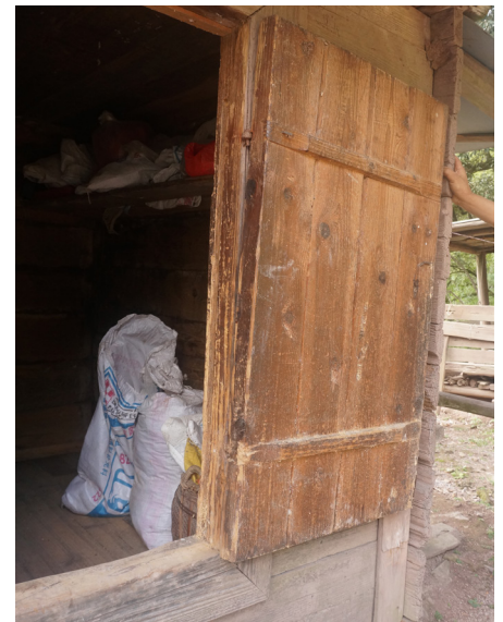
Fig 3.18 A groove in a door post of the granary.
