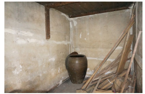
Fig 3.51 Plastered walls in a storeroom.
