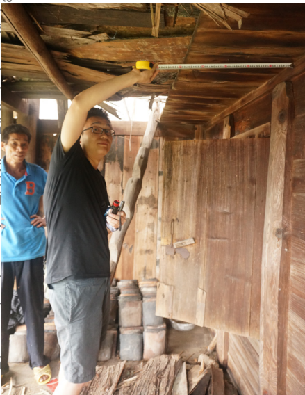
Fig. 4. 88 The extending ceiling planks.
