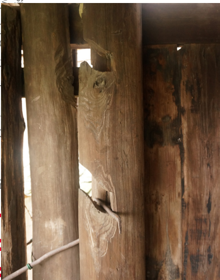
Fig. 4. 89 A wooden boards with notches in the granary
