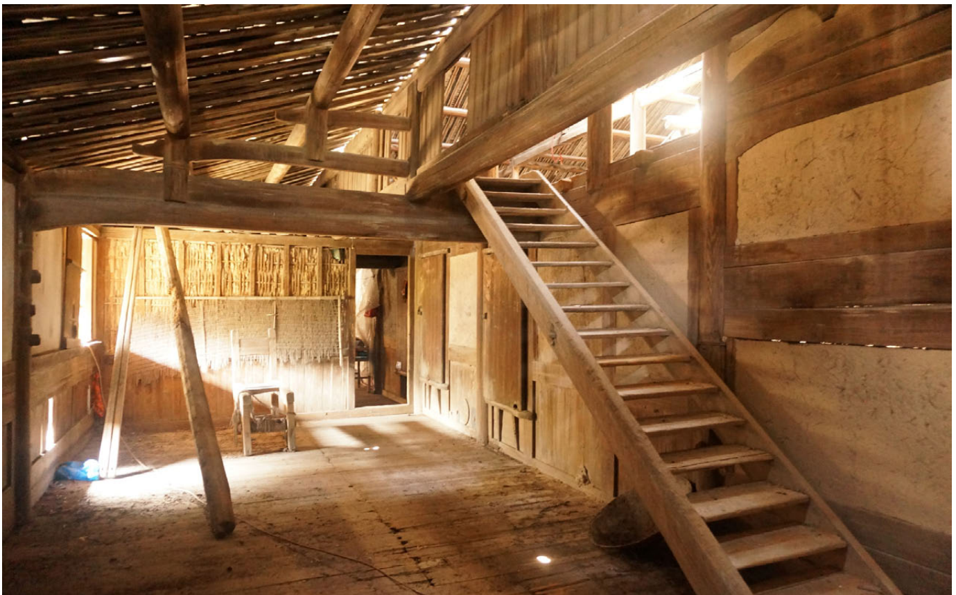
Fig 3.43 Storerooms along a veranda.
