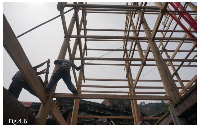
Fig.4.6 Adjustment work after the erection of the main framework.
