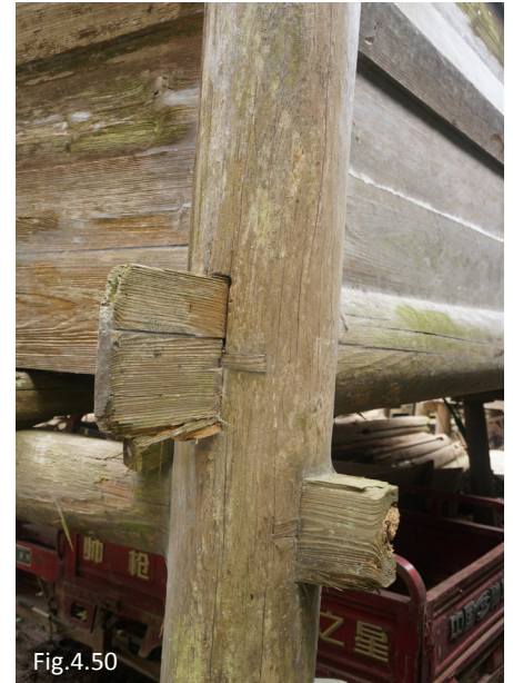
Fig.4. 49 The main framework of the granary
