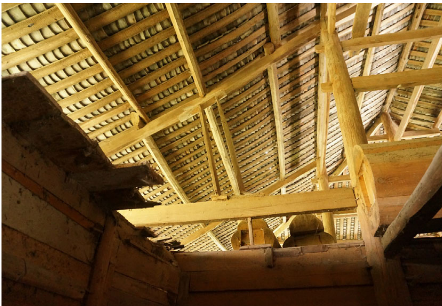
Fig.4. 71 Construction detail of a corner of the granary
