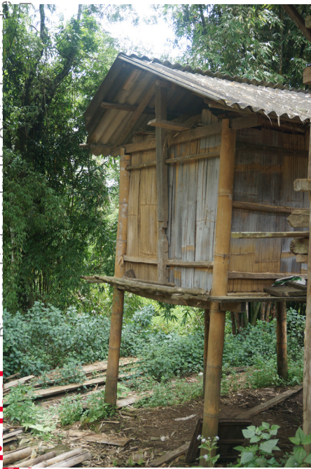
Fig. 5.23 A granary with the bamboo structure in Zhanglang.
