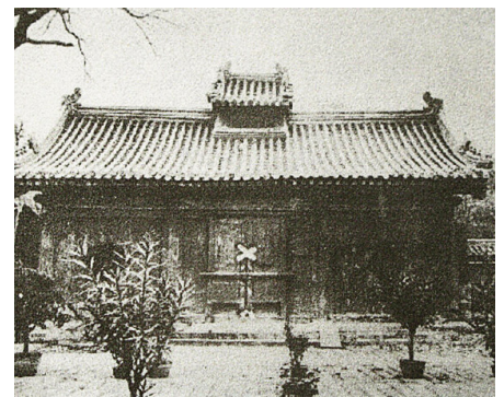
Fig 2.37 A typical Ao with three Jian in Xiannong Altar (source: Jhr mr dr A.J. van Citters)
