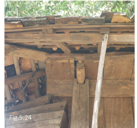
Fig. 5. 24 A perpendicular plank is used for fixing the ceiling boards.
