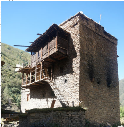
Fig. 6. 41 . Locals put a long wooden plank connecting the end of the lowest veranda to the ground floor as an inclined gangway.
