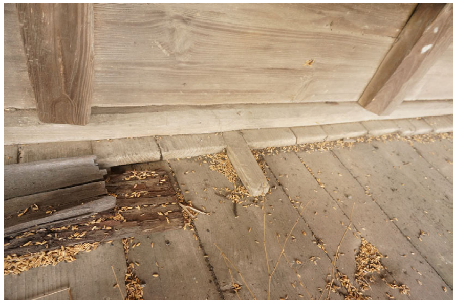
Fig. 4.117 The overlap floors beneath the front wall of storerooms.
