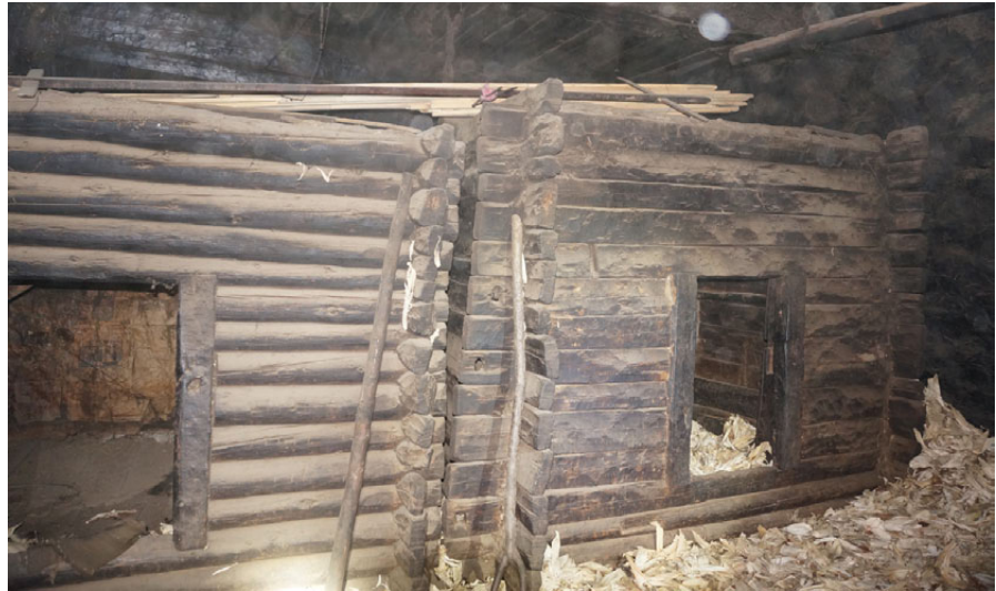
Fig.6. 45 Thick wooden planks are also used for building log constructions in some cases.
