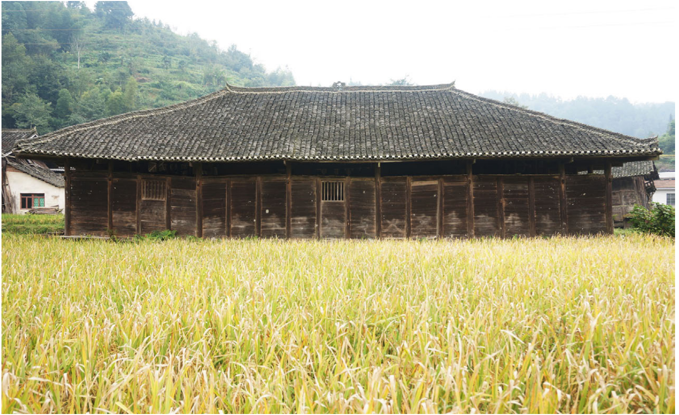
Fig 2.43 A large community granary, Qingzai, Liping, Guizhou.
