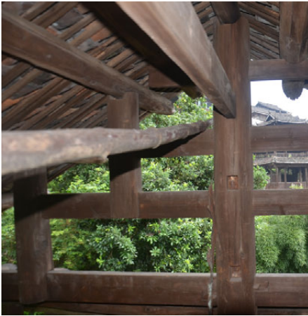
Fig.4. 87 Holes cut in the central pillar of the granary
