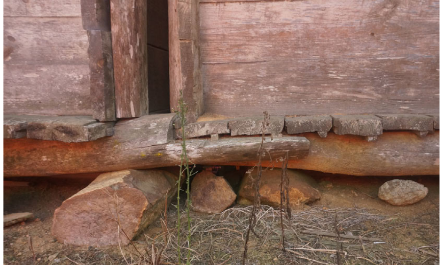
Fig 3.16 Wooden wedges were inserted between the floor and the external frame.
