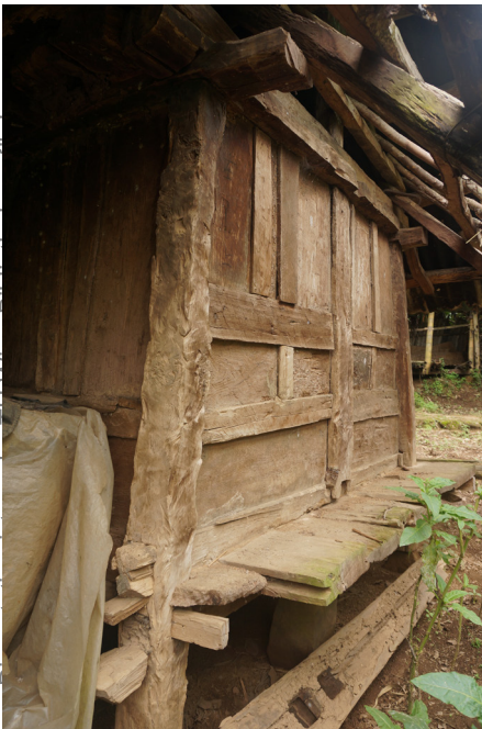
Fig. 5.08 A Wa granary with reused wooden members.
