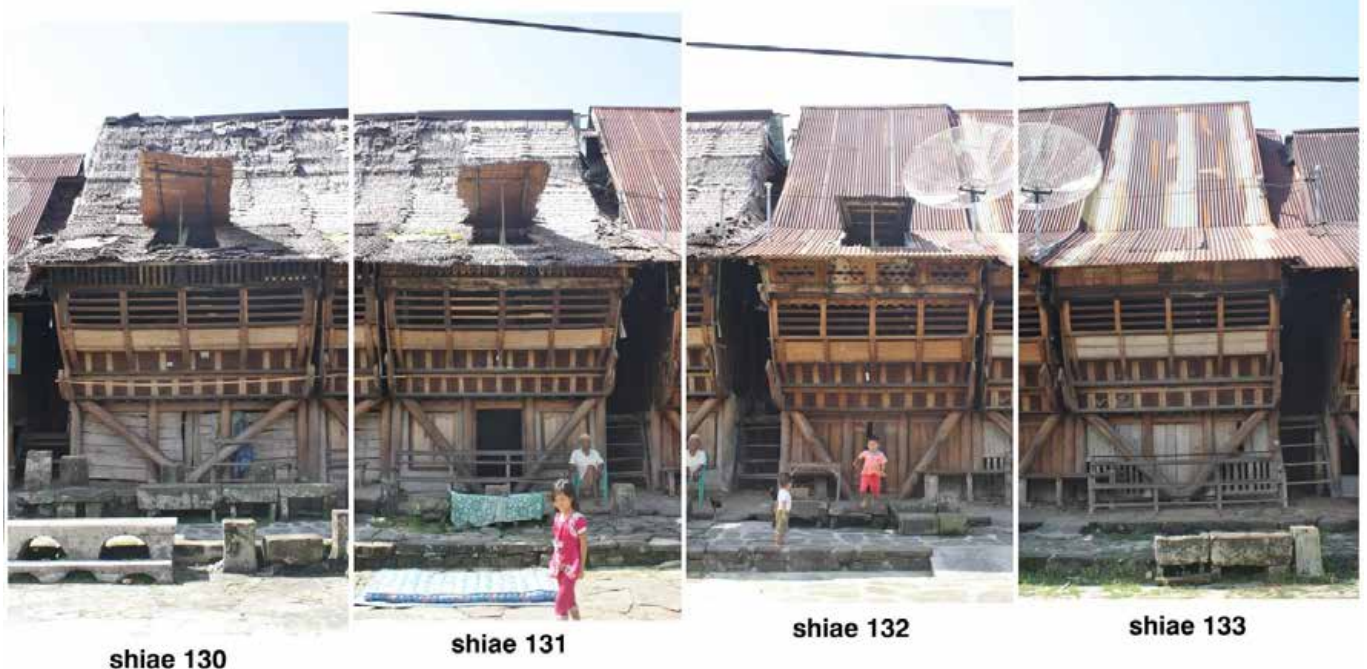
fig. 86: sago palm leaf covering – corrugated iron covering of the TSH
