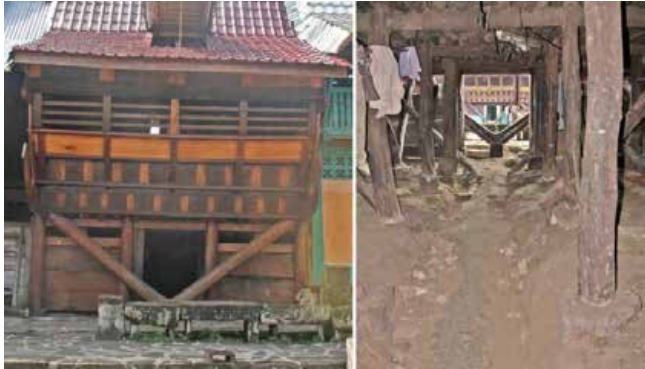
fig. 157: TSH "shiae 091" without the modification of the substructure
