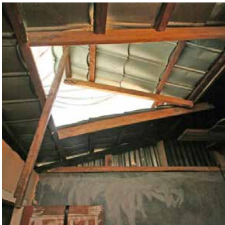
fig. 150: roof top window of the extension "shiae 123"
