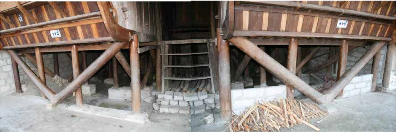
fig. 74: Substructure of two traditional houses in Bawögosali
