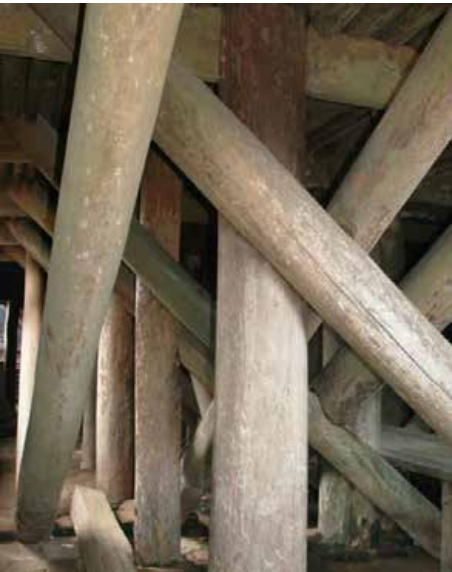
fig. 75: Substructure of the Omo Sebuva in Bawomataluo
