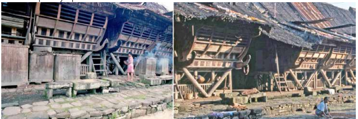
fig. 156: storage boxes in front of the substructure; without any changes of the substructure – in Hiliamaetaniha
