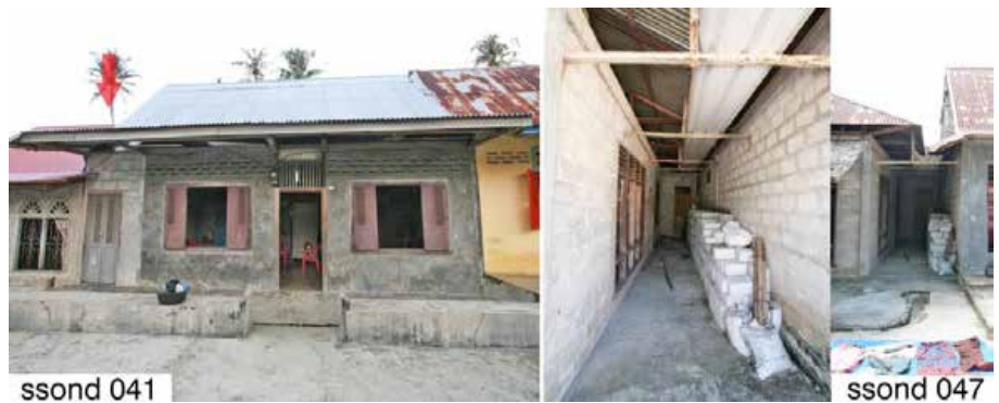
Fig. 202: access to the nourishment and sanitary are between the houses
