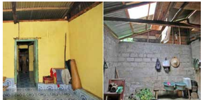
fig. 151: plastered and painted wall "shiae 042" and bricked wall "shiae 111"
