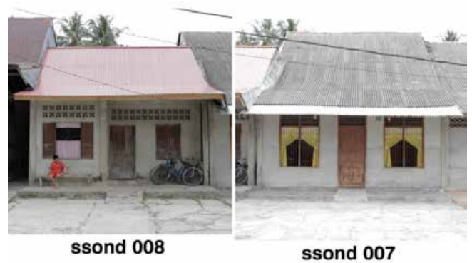
fig. 209: step back of the front facade
