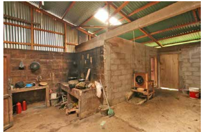
fig. 218: nourishment and sanitary area "ssond 025"
