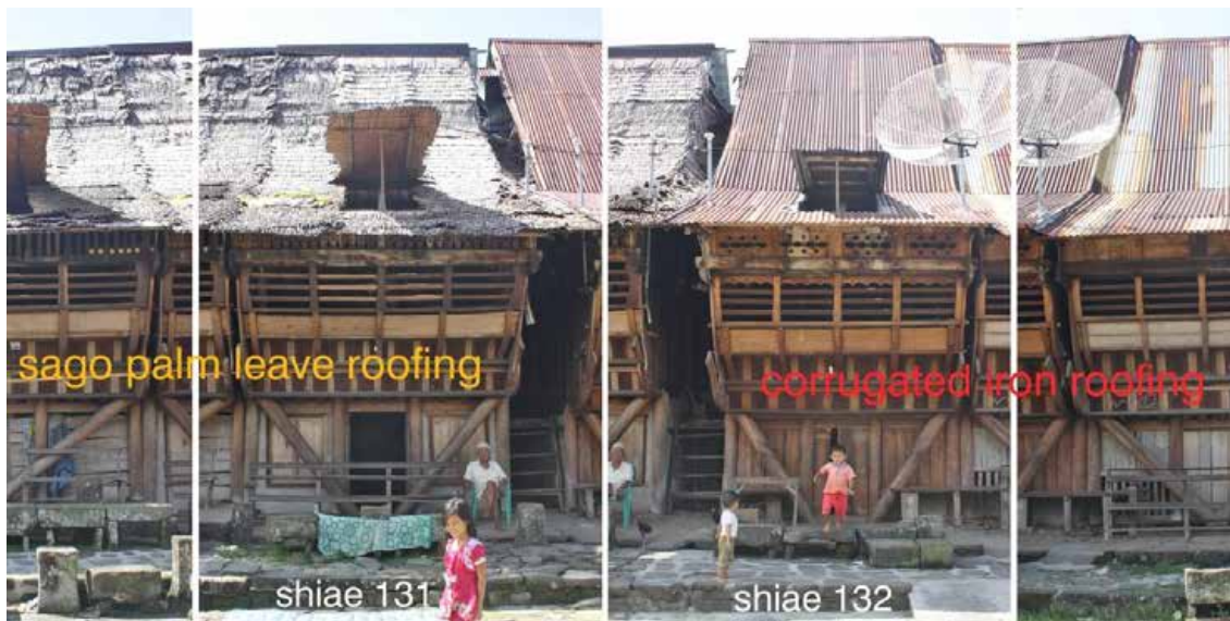
fig. 70: different types of roof covering
