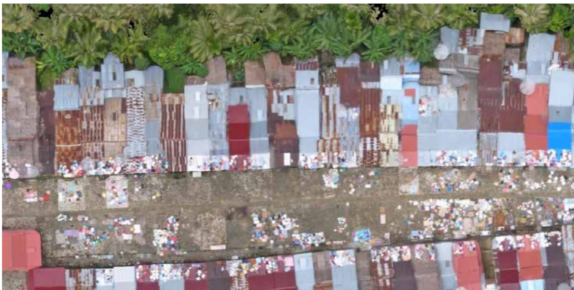
fig. 148: roof covering material of the extensions
