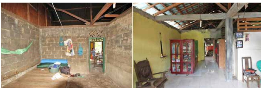
fig. 174: construction of the MH “shiae 516”, “shiae 506”
