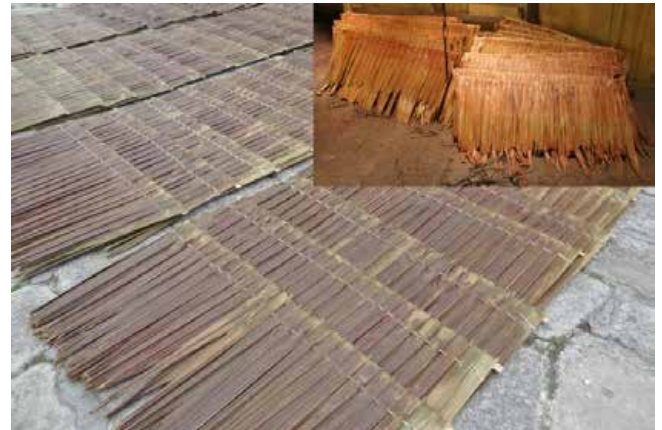
fig. 85: roof covering elements
