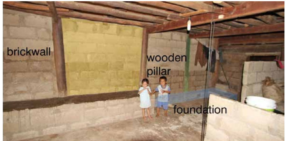
fig. 167: construction of the modification "shiae 043"
