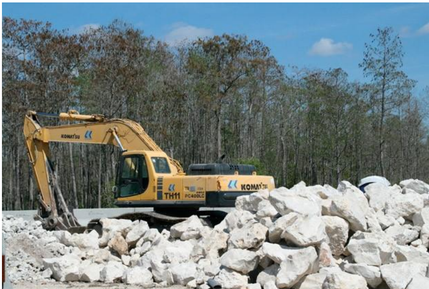
Figure 4 Limestone at a road construction site 11
