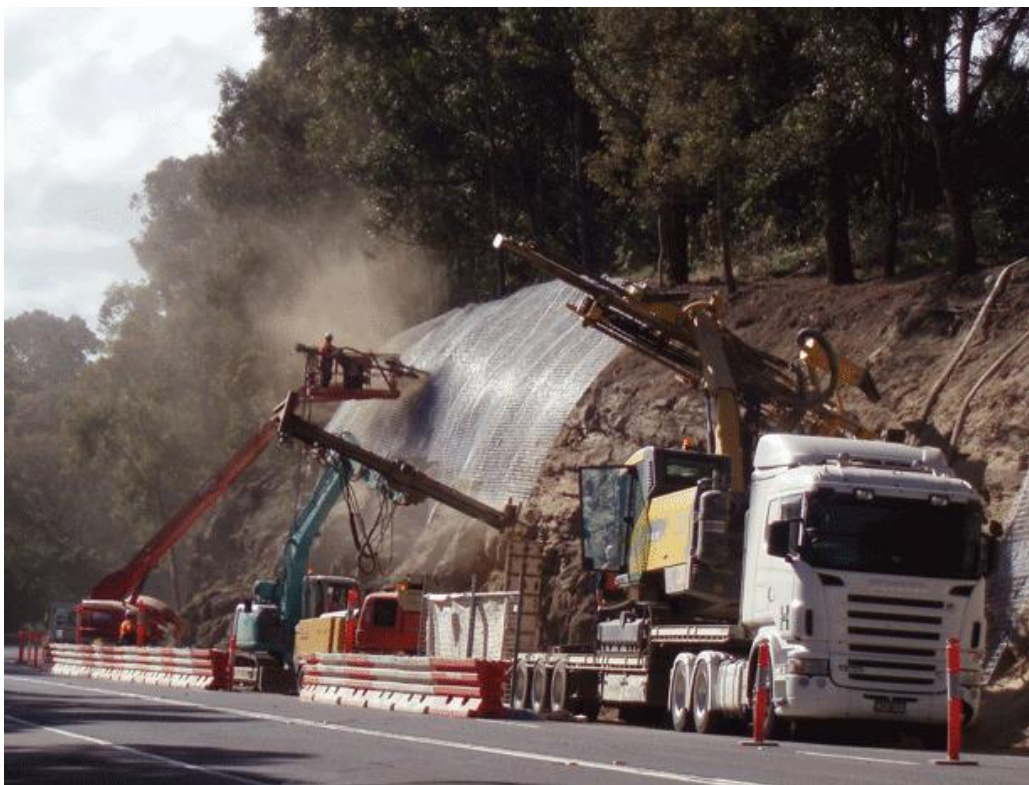
Figure 7 Drilling equipment securing a slope using metal mesh 22
