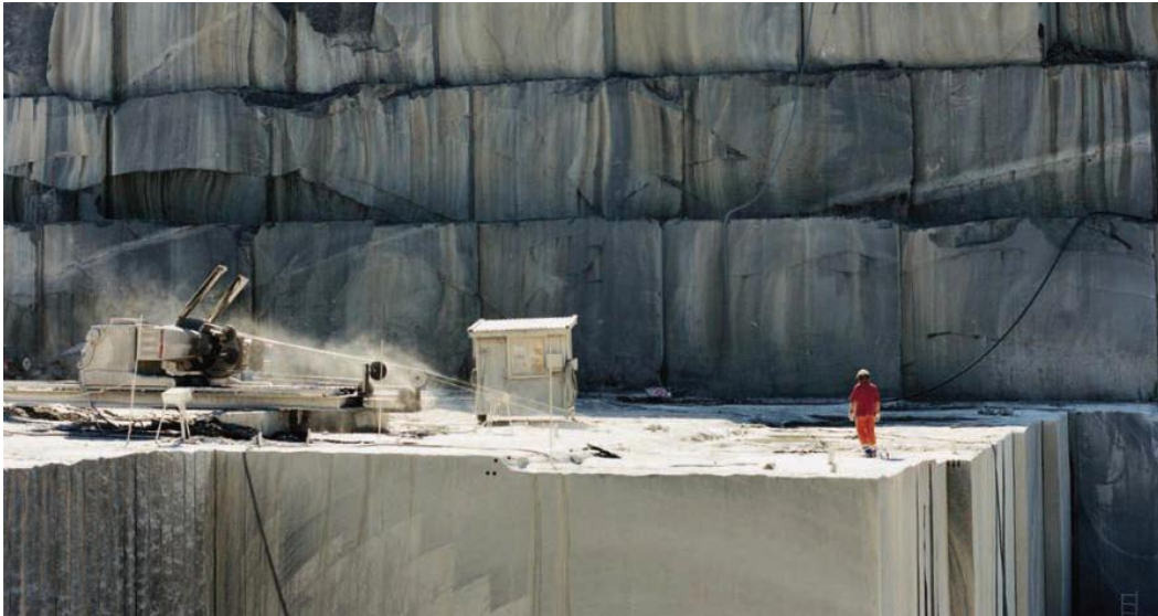
Figure 42 Deep cutting of marble using diamond wire 113
