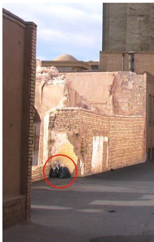
Figure 116: Garbage management in Yazd. Image from: author
