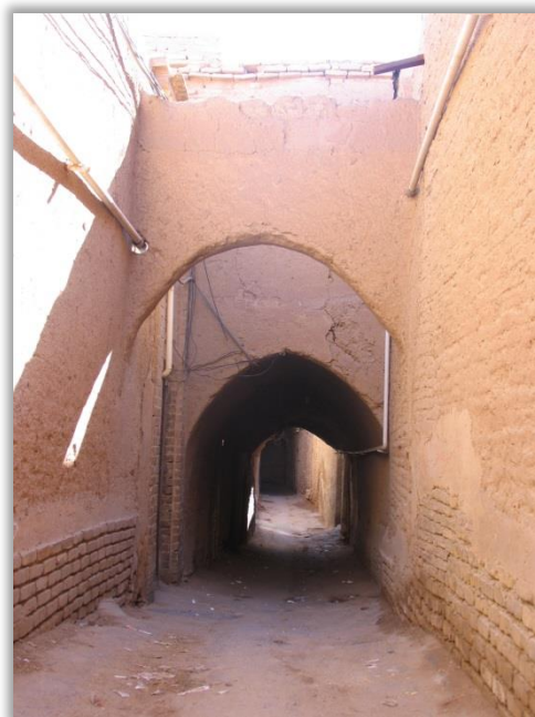
Figure 115: one narrow and covered passageway in Yazd. Image from: author
