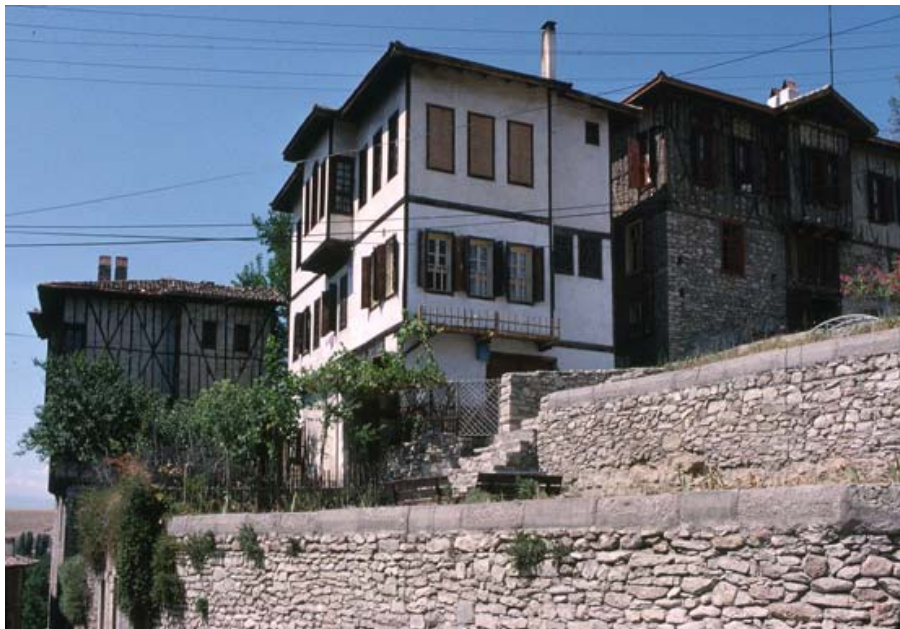
Fig. 23: Traditional houses viewed from Yokuşbaşı sokak, Safranbolu.
