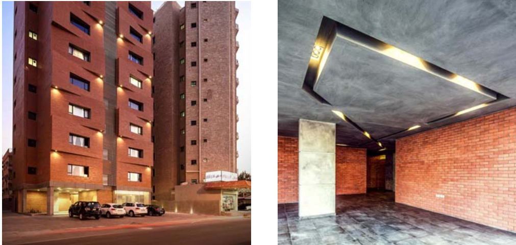
Fig. 65: Studio Toggle, Edges Apartments. Ground floor entrance is open to the street. Thus, the public space flows and transform into semi-public space, which leads further to the vertical circulation core.
