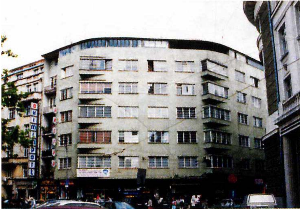
Fig. 32: Residential building, Hristo Berberov, Sofia 1939; An attempt to straighten the geometry of the building in the corners.
