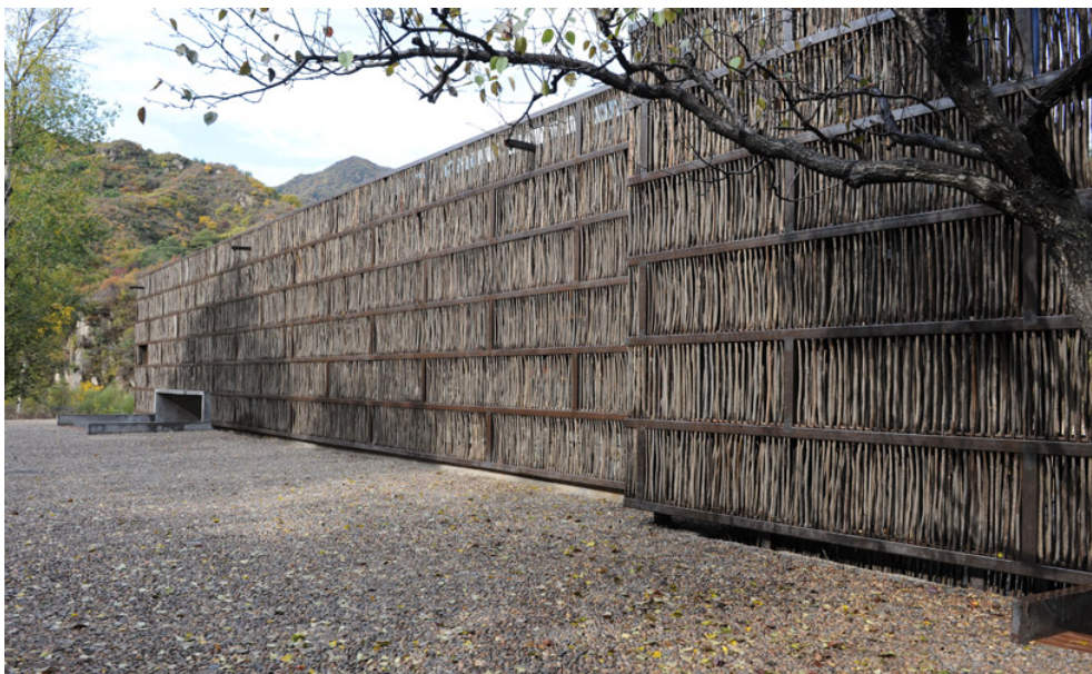
Fig. 5: Liyuan Library. The cladding of the building is extracted from textures, found in the local villages, and merge the Library with the environment.
